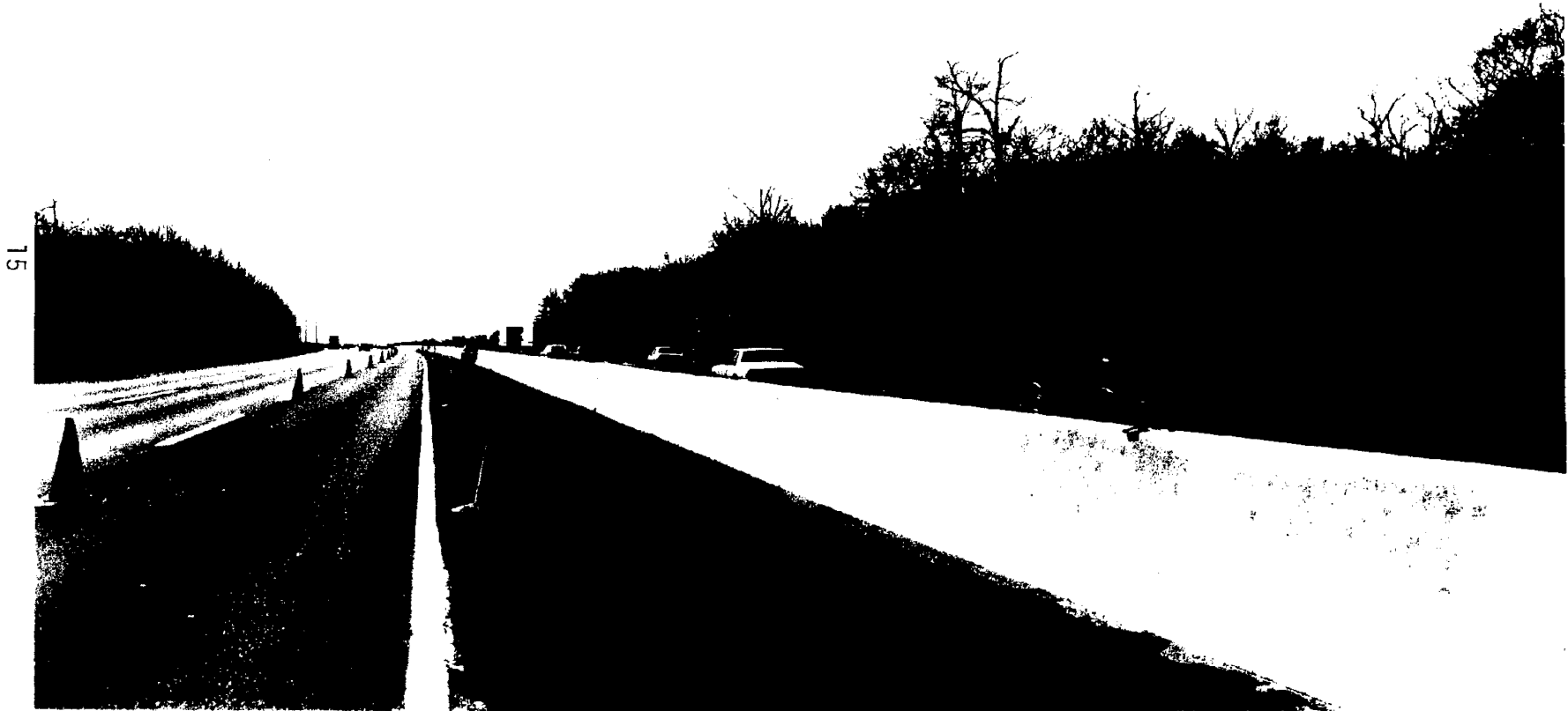
Figure 5. Completed barrier with asphalt shoulders in place.
