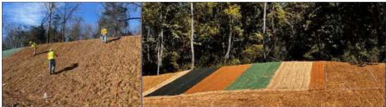
Figure 2. Seeding the Marked Subplots (left) and Completed Installation of Rolled Erosion Control Products (right). The photo on the right shows buffer zones around the study plots and a marked control plot (far right) prior to the contractor hydroseeding the remaining VDOT project area.
