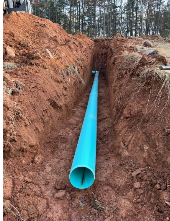
(b) trench for underdrain
