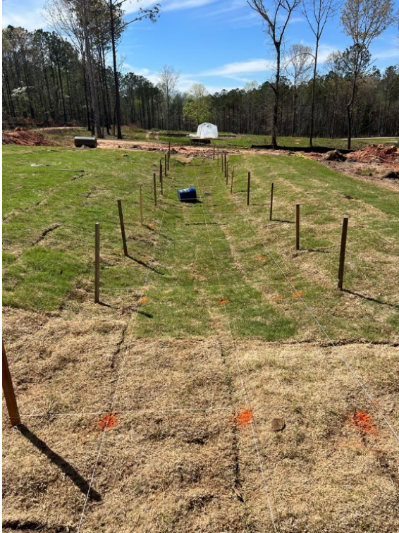
(a) wooden stakes and strings installation
