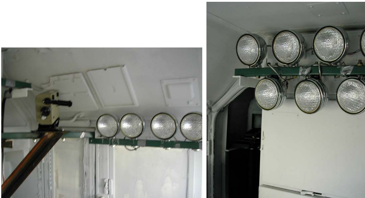
Figure 29. Experiment No. L-1, Aft-View and Oblique-Side-View Lights and Fixtures
