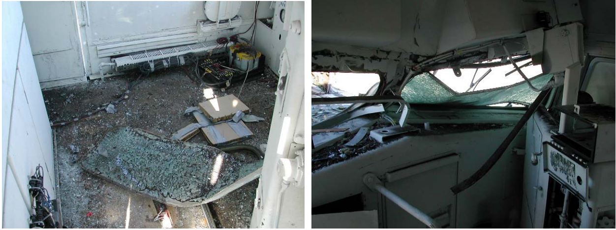
Figure 42. Experiment No. L-1 - Post-Test View of the Locomotive Interior
