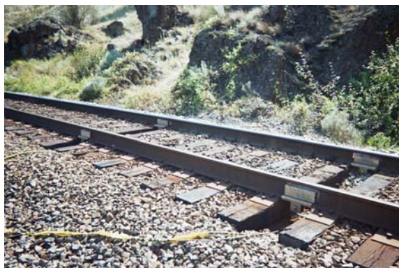
Figure 2 shows the instrumented cribs in 6 degree 30 minute curve at MP 11.95.
