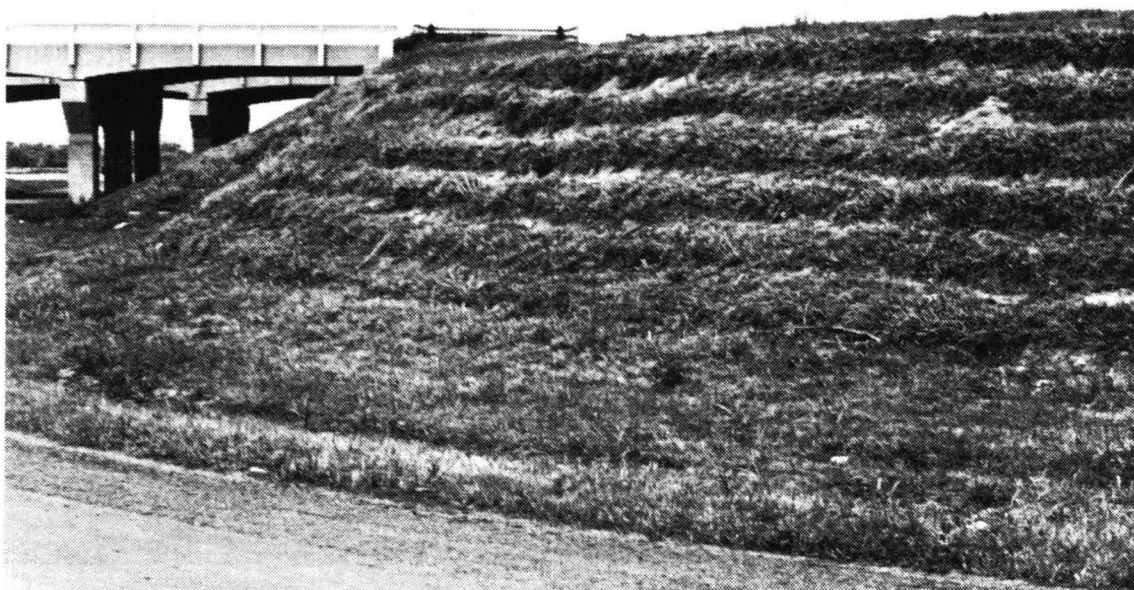
Figure 1.2. The operation of maintenance equipment, mowers particularly, on highly erosive cut (top photo) and fill (bottom photo) slopes destroys the vegetative cover and accelerates soil erosion by physically tearing the grass from the soil as the tractor slides in traversing the slope.
