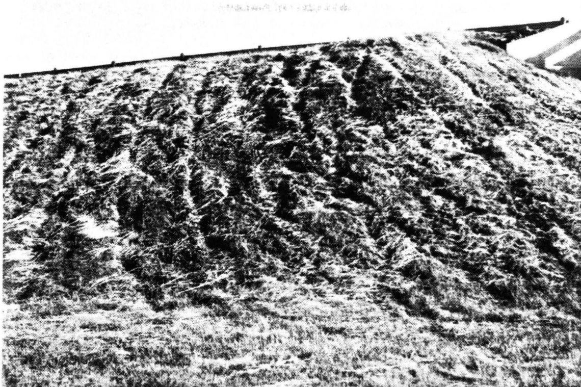
Figure 1.3. Soil erosion is greatly accelerated by the destruction of grass and the creation of ruts as the mower wheels spin as they ascend or slide in an attempt to stop or turn on the way down.
