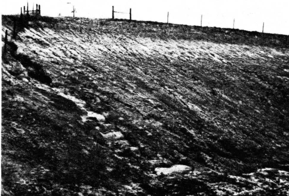
Figure 1.5. Soil erosion occurs as a result of improper design through omission of a physical barrier along the shoulder to concentrate and remove excess water (top photo), and because of inadequate rights-of-way interceptor ditches could not be constructed on top of cut slopes particularly for the orderly removal of excess water (bottom photo) from terrace outlets, or adjacent watershed.
