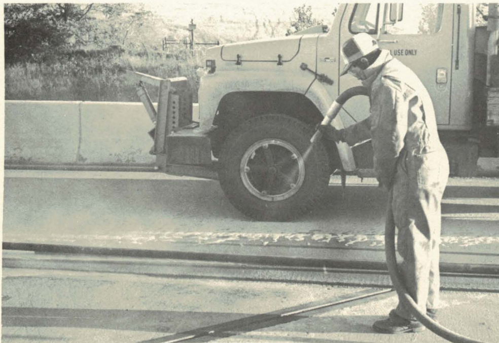
Figure 8. The deck was thoroughly sandblasted clean.
