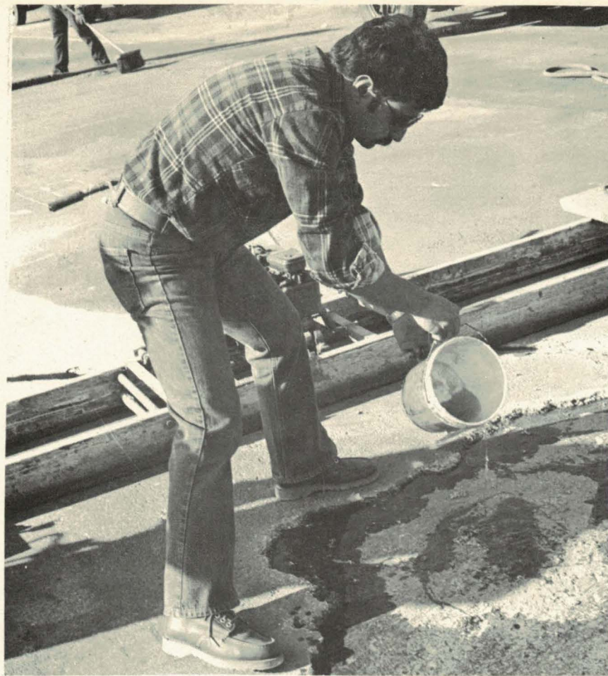
Figure 23. Delaminations were generously tackcoated.
