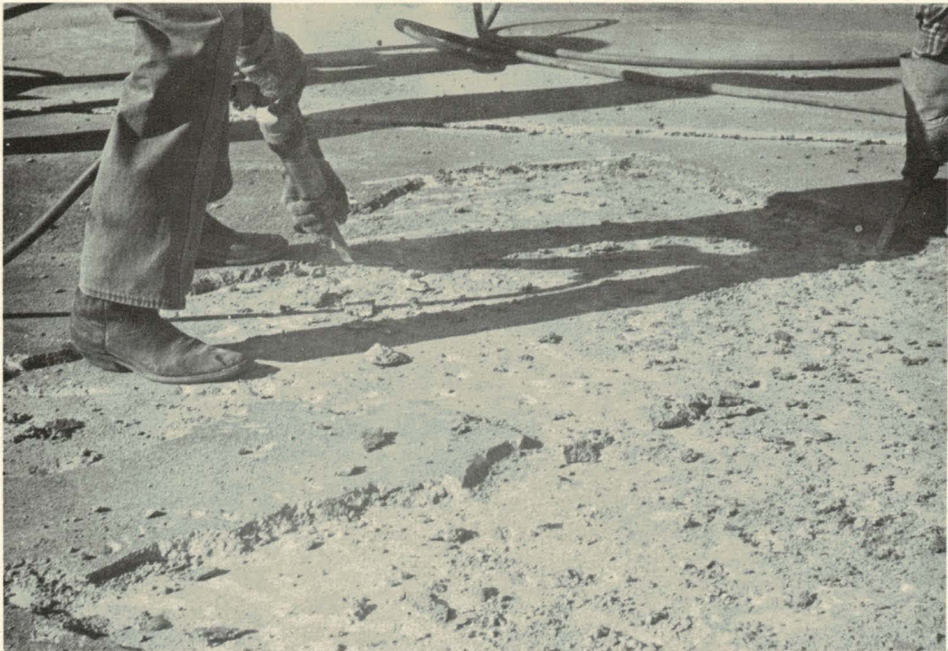
Figure 21. Unsound polymer concrete was jackhammered away.
