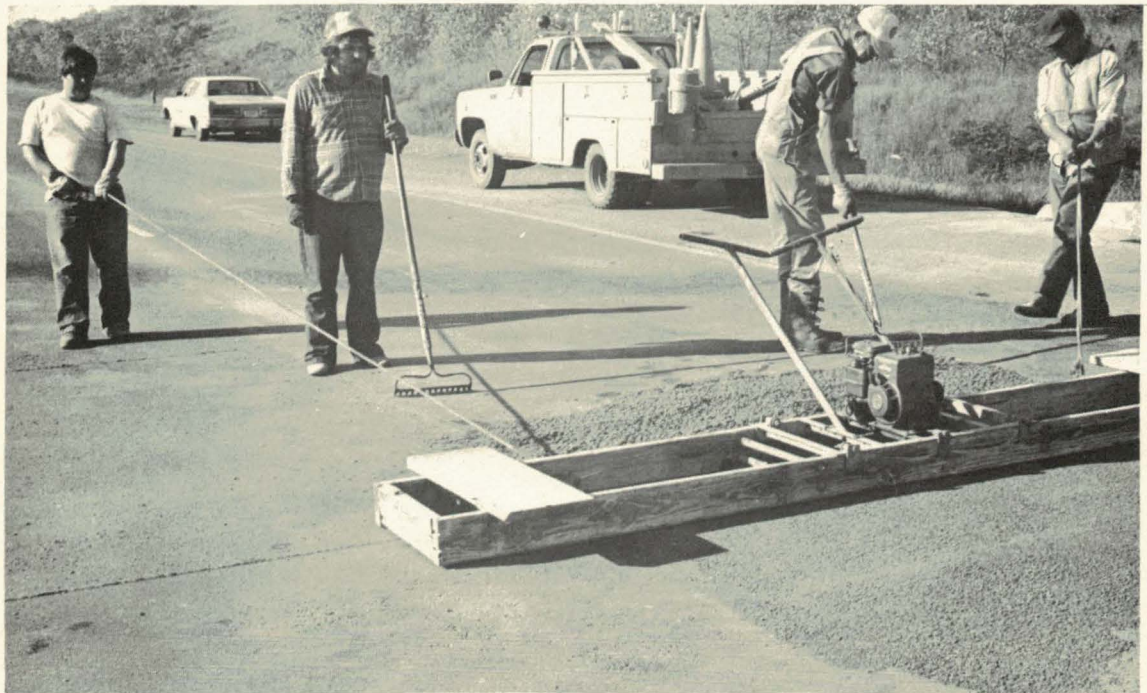
Figure 24. A shopbuilt screed compacted the patches.
