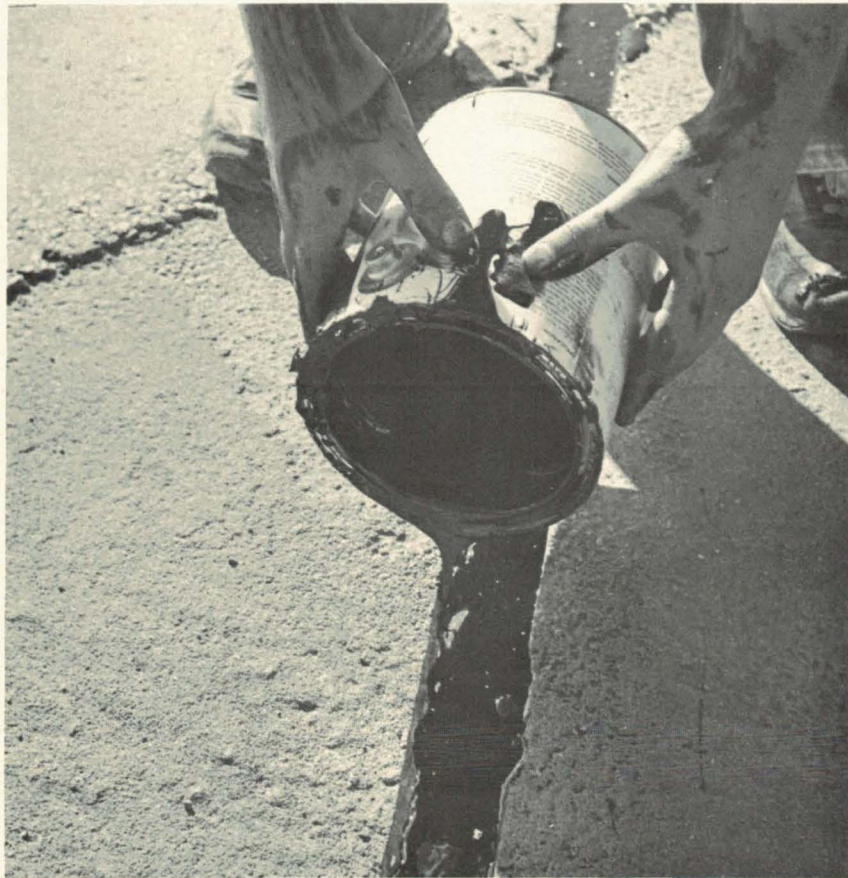
Figure 20. Expansion joints were filled with a rubber-like material.
