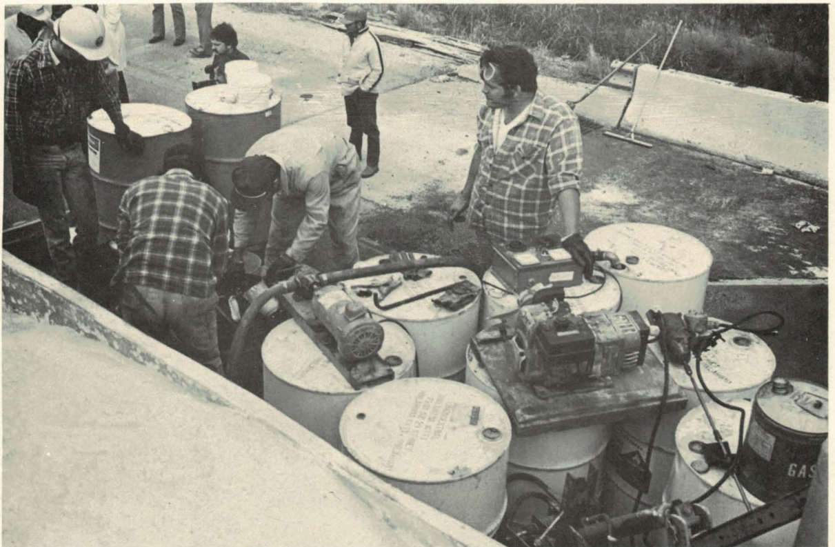
Figure 10. The chemical truck held the resin, catalyst and pumps.
