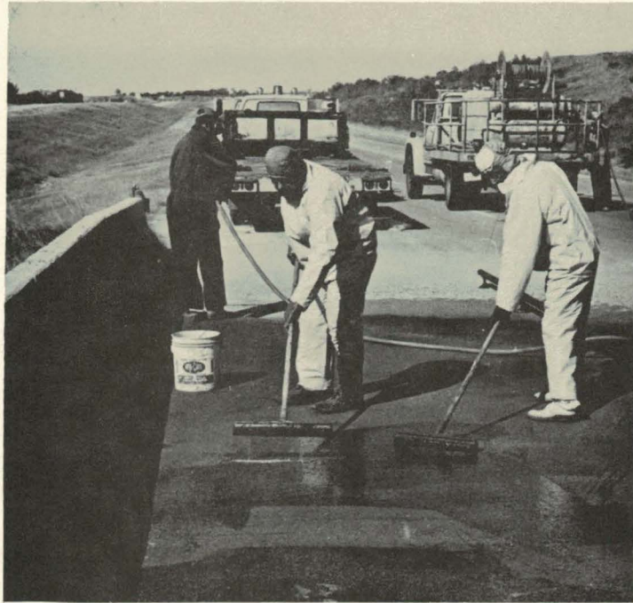
Figure 15. Areas having lean resin content were squeegeed with additional resin.
