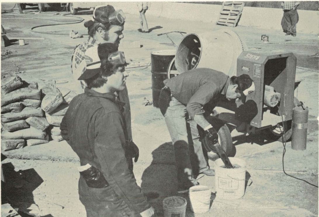
Figure 22. For patching, polymer concrete was mixed with a portable mixer and placed by hand.
