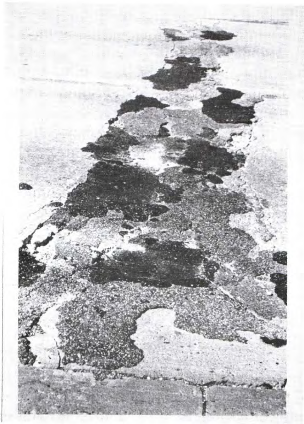
Figure 1. Deteriorated Joints
