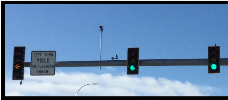
Figure 6 Video and Optical Detector for Preemption
