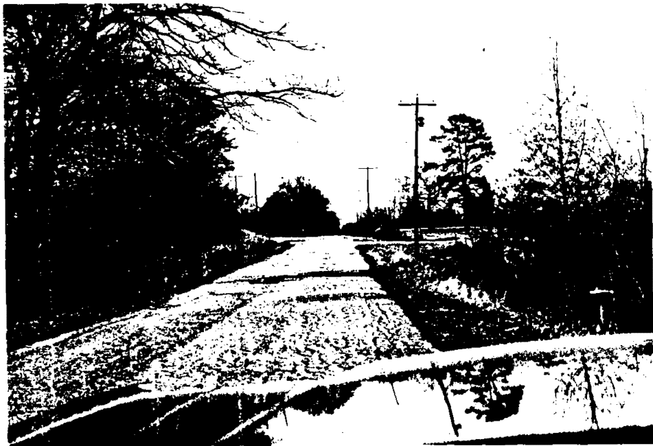
Figure 13. Information-deficient horizontal curve with a tangentially intersecting side road.
