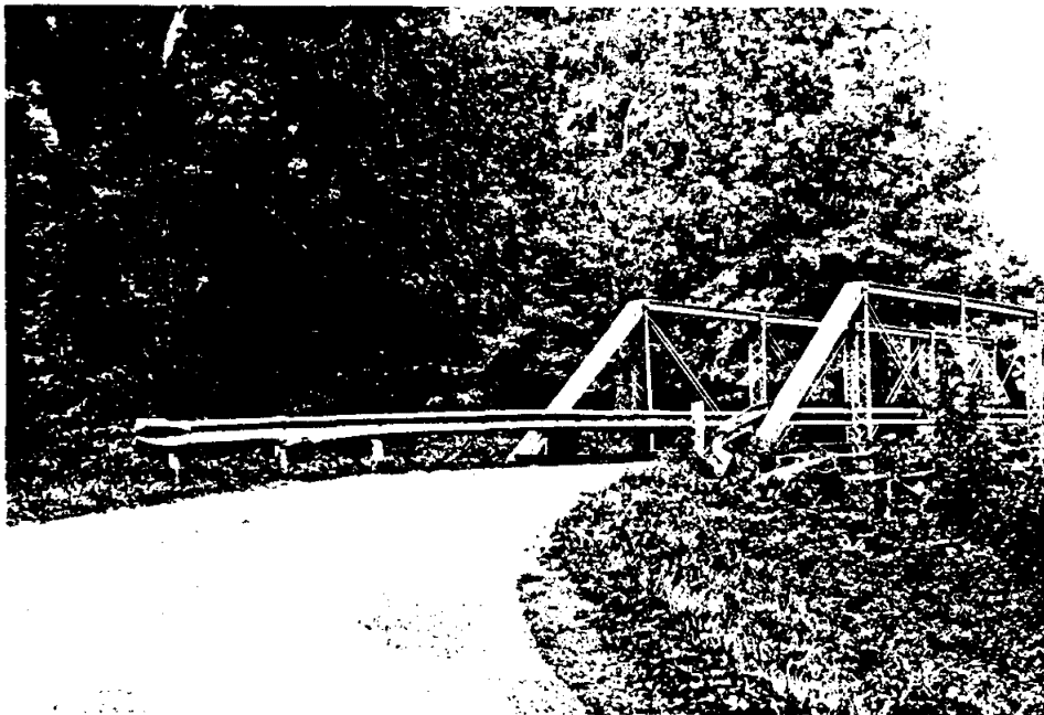
Figure 9. View of the 12-foot-wide bridge from a distance of 50 feet.
