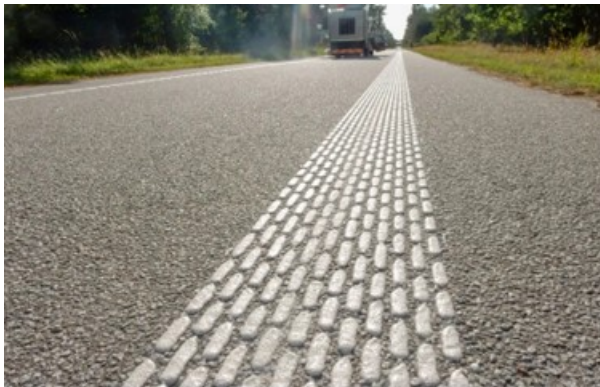
Figure 4.19 Geveko Markings new road marking profile (Geveko, 2018)
