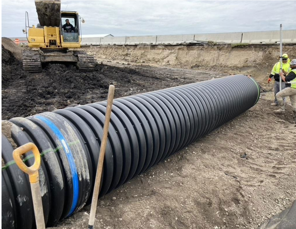
Figure 2.13 Joining of second stick of pipe (M 294 R) to first stick (M 294 V) via bell-and-spigot watertight joint
