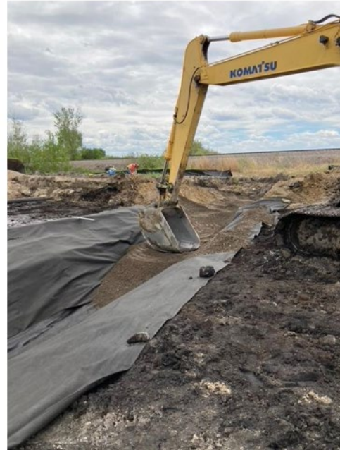
Figure 2.9 Wrapping the trench in geotextile to prevent mitigation of fines into backfill
