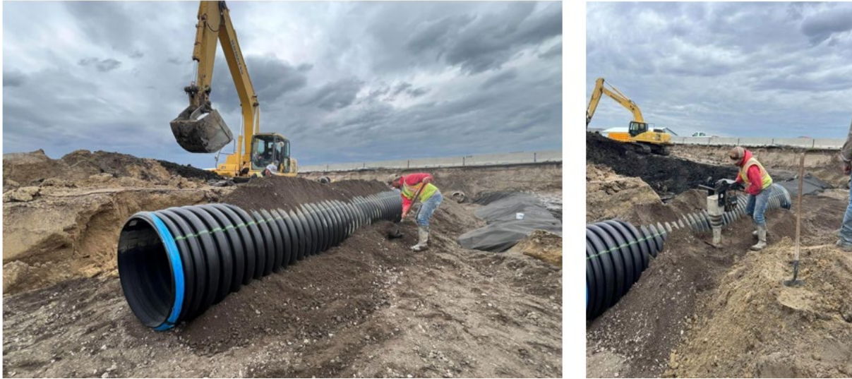
Figure 2.20 Installation of backfill materials around culvert pipes; a shovel was used to knife backfill materials into the haunch area, and a jumping jack compactor used to compact lifts
