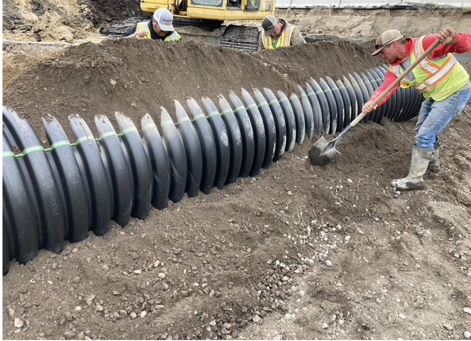
Figure 2.11 Knifing backfill materials into the haunch area to ensure adequate support
