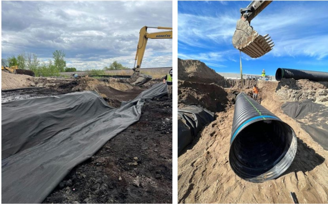
Figure 2.18 Placement of bedding material and initial pipe for installation underneath westbound lanes
