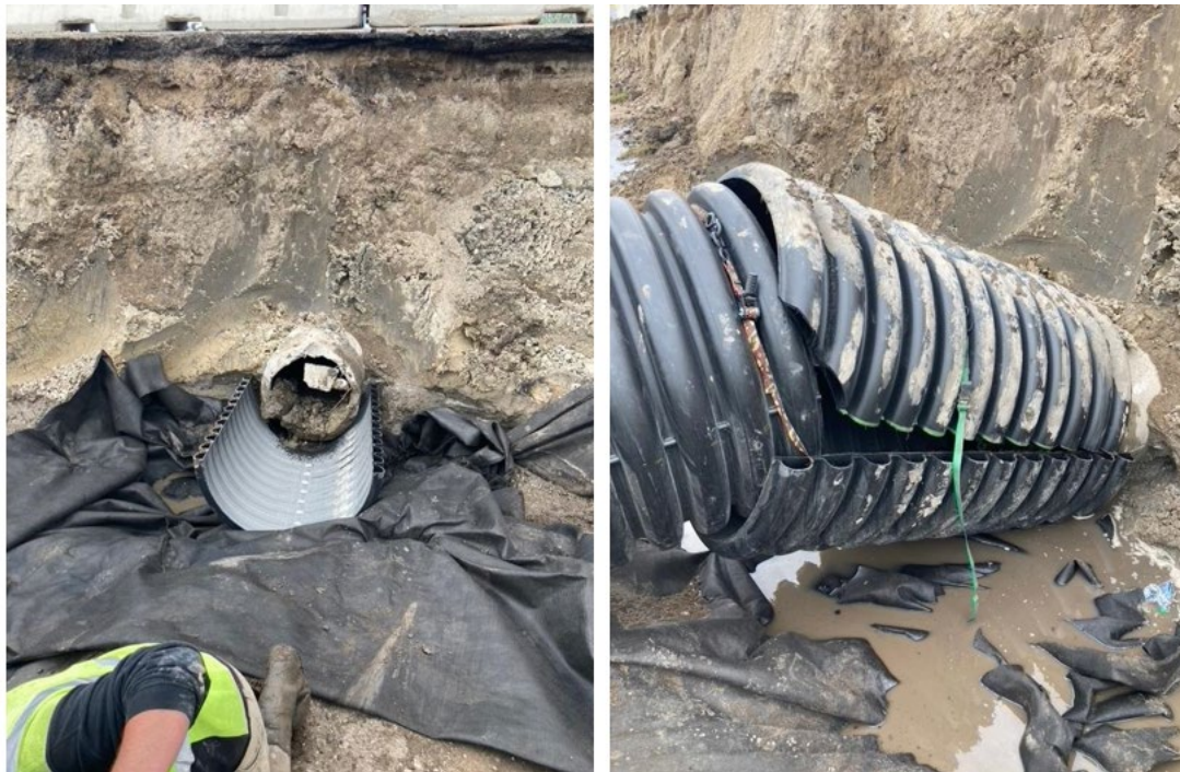
Figure 2.15 Installation of temporary connector of M 294 R pipe to existing 24-in. RCP culvert until westbound lanes are constructed
