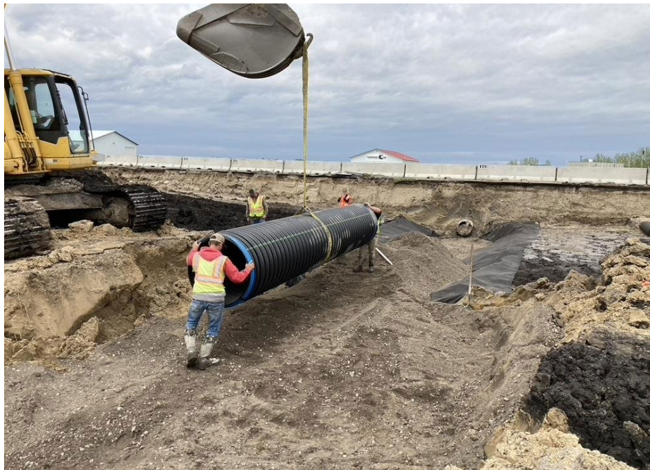
Figure 2.10 Installation of first stick of pipe (M 294 V) onto uncompacted bedding
