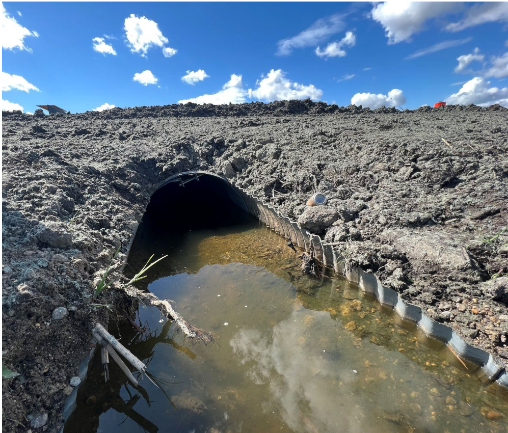
Figure 2.24 Photograph of culvert taken 30 days after installation
