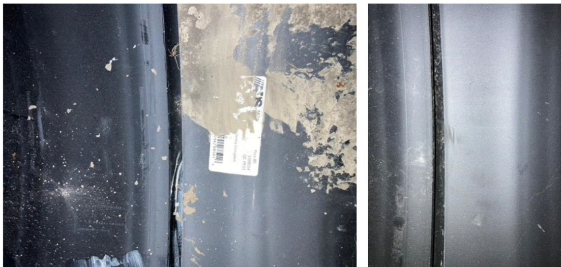
Figure 2.16 Inspection of joint gaps to ensure proper seating of joints
