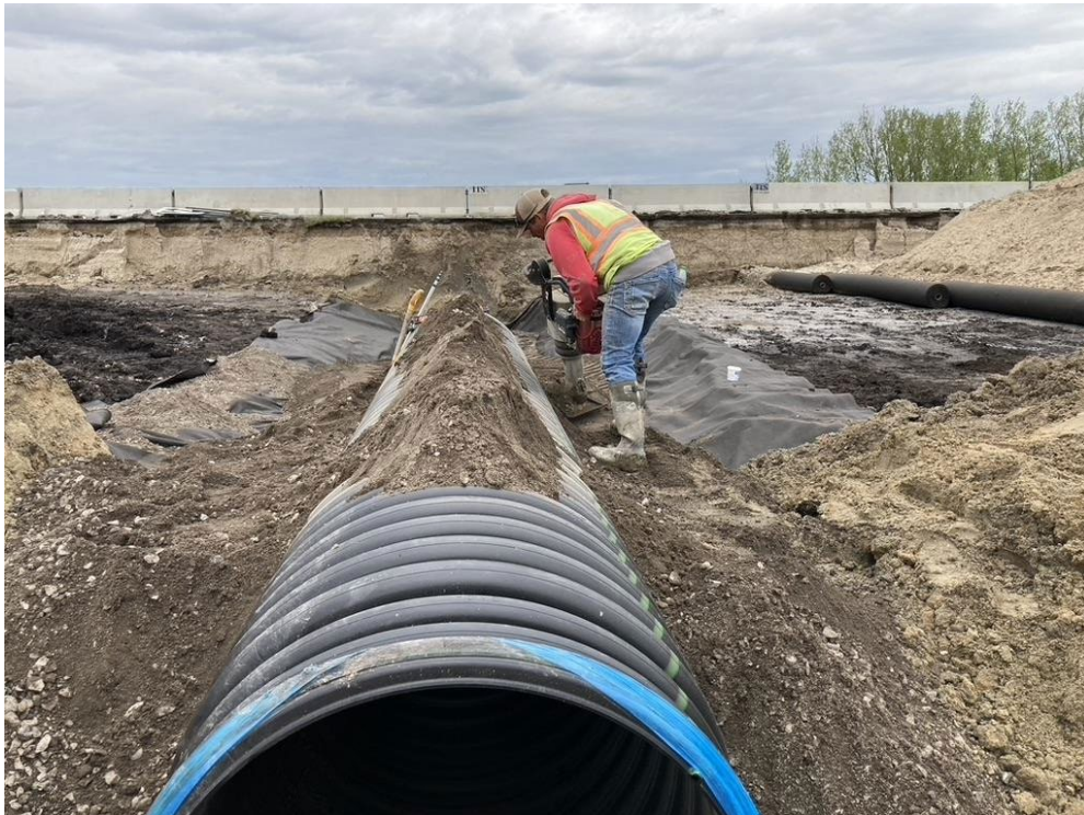
Figure 2.12 Compaction of backfill materials in lifts with vibratory compactor
