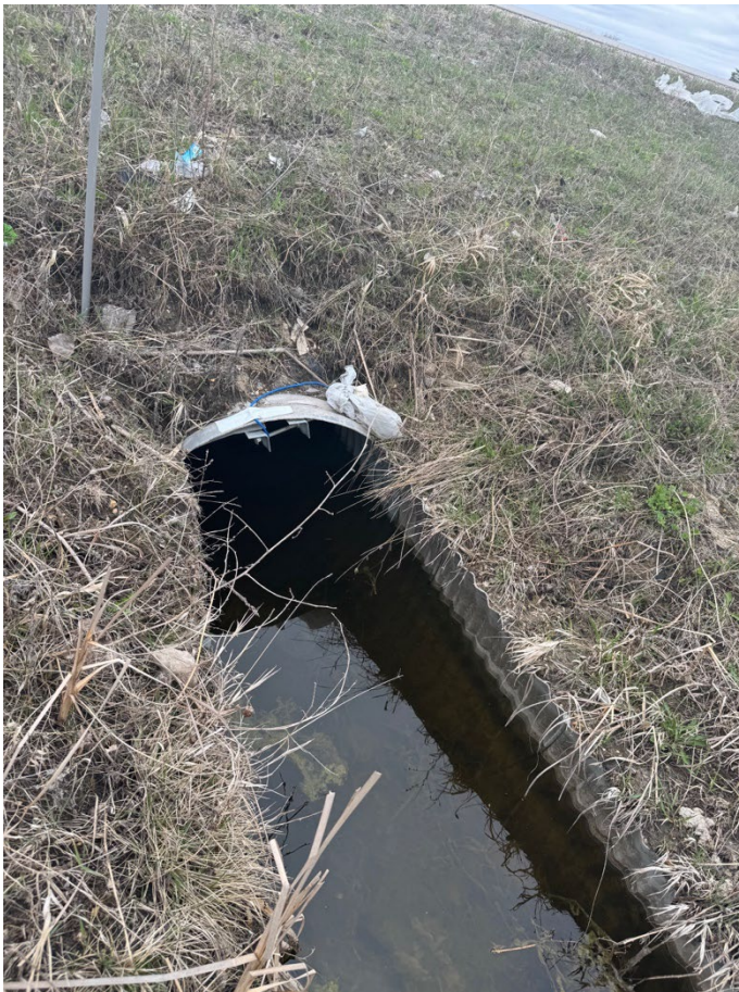
Figure 3.13 April 28, 2024, site visit - water level was over 60% full, and the pipes were deemed unsafe to enter
