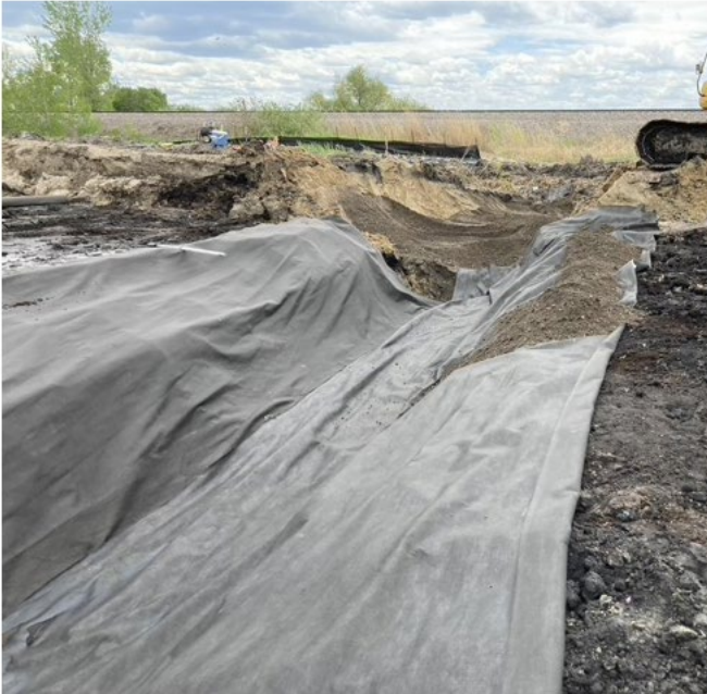
Figure 2.9 Wrapping the trench in geotextile to prevent mitigation of fines into backfill
