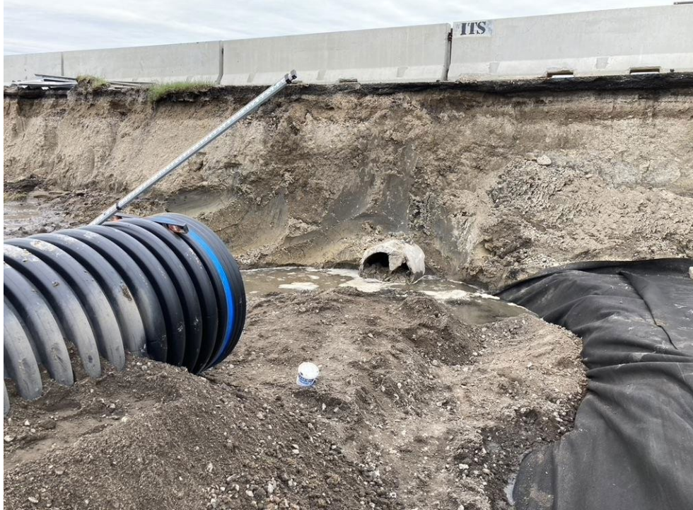
Figure 2.14 Installing a third stick of pipe
