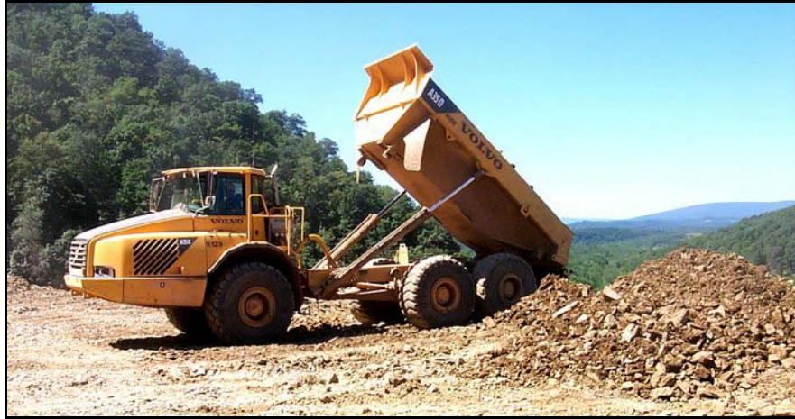
Figure 5.33 Construction vehicle involved in cyclical operation (Photo #1005)
