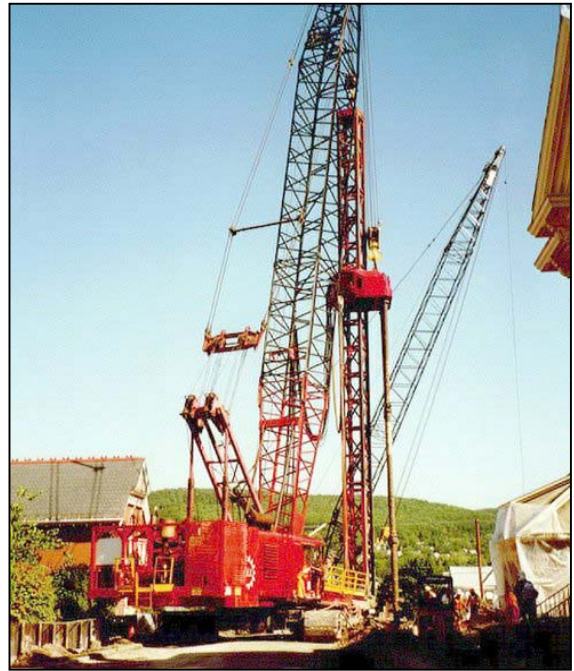
Figure 5.24 Pile driving operation (Photo #856)
