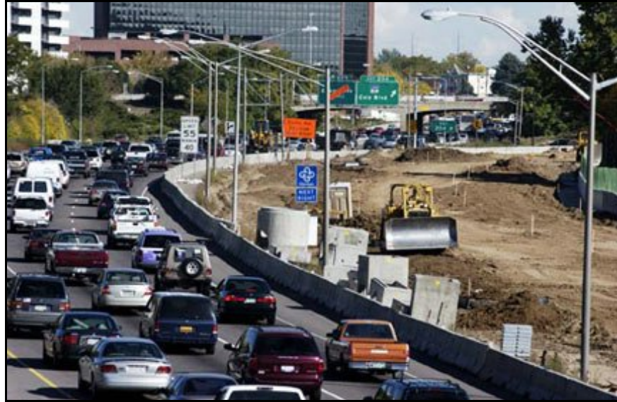
Figure 5.30 Communities can be affected by traffic diverted by construction activities (Photo #1046)
