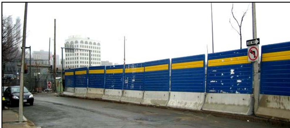
Figure 7.31 Temporary barrier of plastic material (Photo #194)
