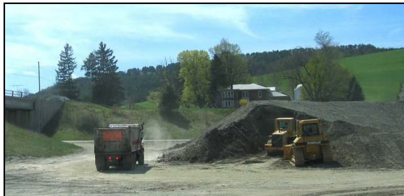
Figure 5.29 Stock pile operation in vicinity of residence (Photo #1258)
