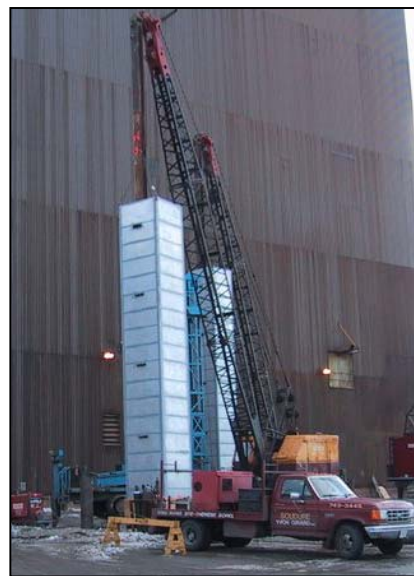
Figure 7.16 Examples of pile driver shielding and damping (Photos #1277, #1281 & #1308)
