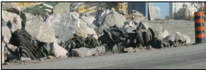
Figure 7.21 Blasting mats constructed with black tires (in foreground of photo) (Photo #261)
