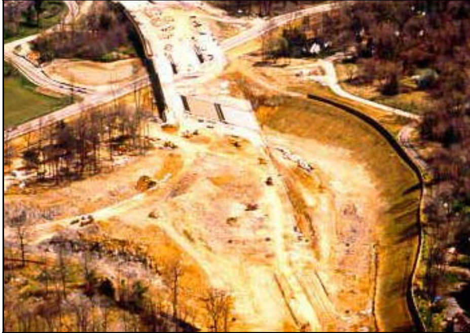
Figure 7.33 Early construction of permanent noise barriers (Photo #472)
