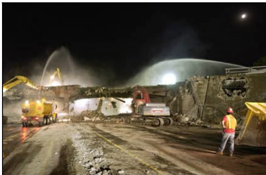
Figure 7.11 Nighttime demolition operation (Photo #1049)
