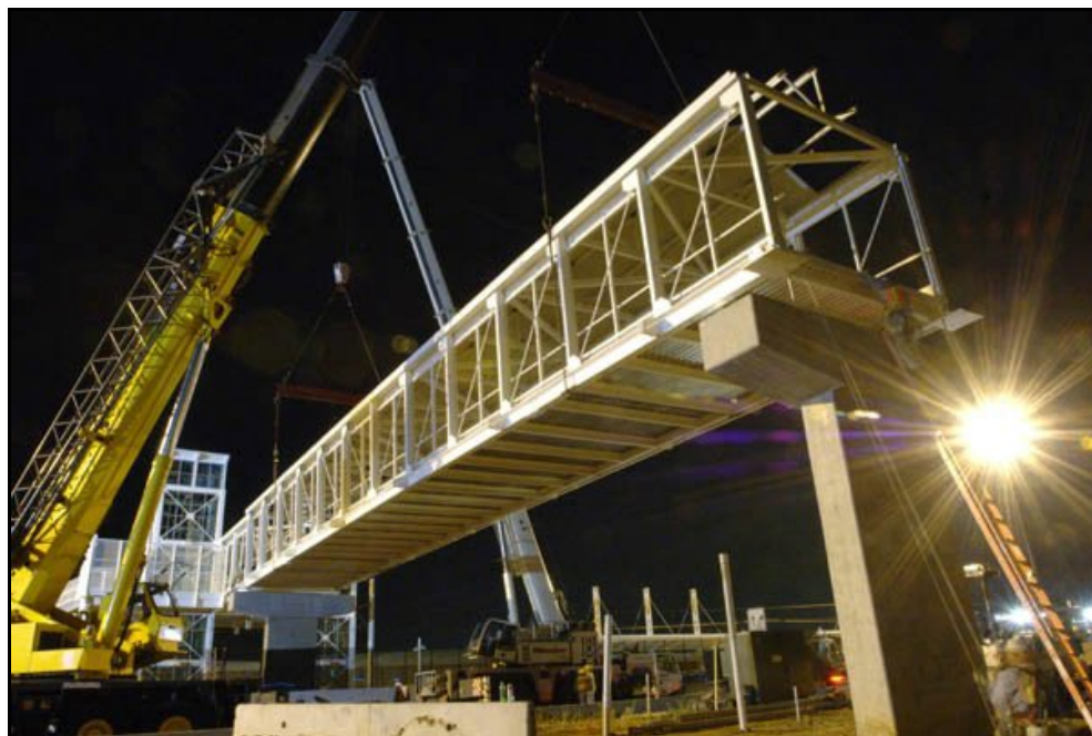
Figure 7.10 Nighttime bridge construction (Photo #661)
