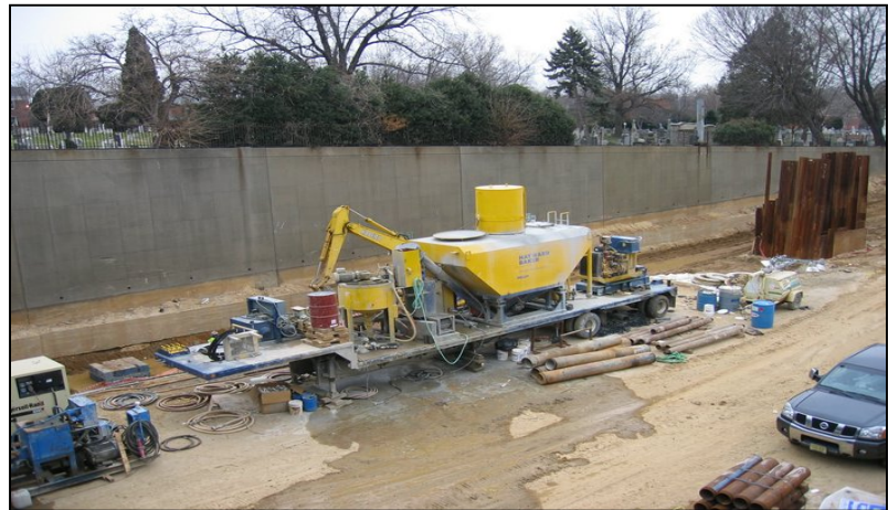
Figure 7.6 Existing retaining wall acting as noise barrier during construction (Photo #543)
