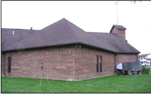
Figure 5.13 Measurements at church; consider also influences of air conditioning units (Photo #1302)
