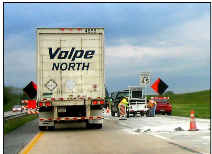
Figure 5.10 Pavement rehabilitation project (Photos #1407 & #1397)
