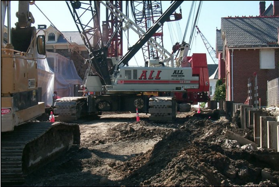
Figure 8.1 Construction in the community (Photo #925)
