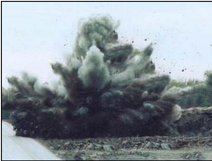
Figure 5.23 Blasting operation (Photo #1309)
