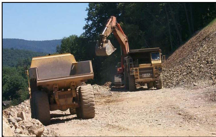
Figure 5.25 Rock excavation operation (Photo #981)
