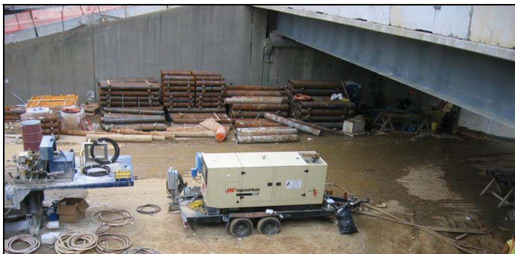
Figure 7.29 Equipment and storage area shielded by existing structures (Photo #558)
