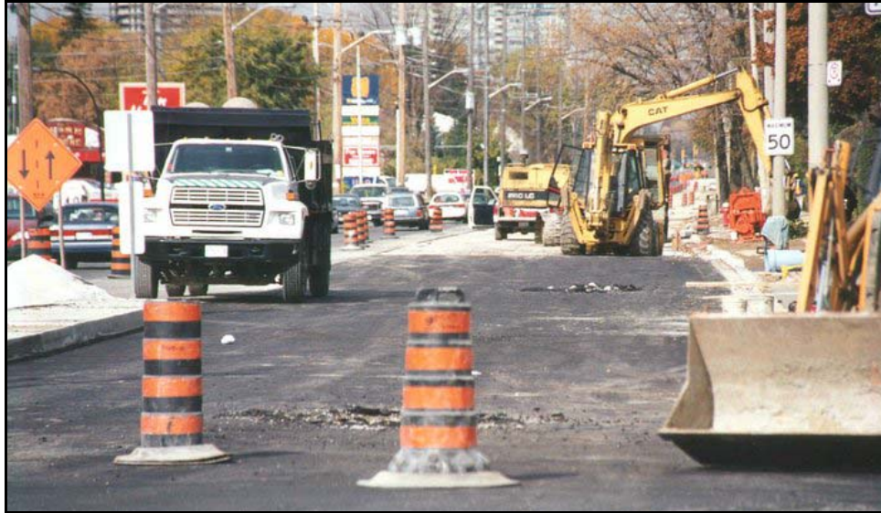
Figure 7.5. Shifting of traffic to accommodate construction. (Photo #1261)
