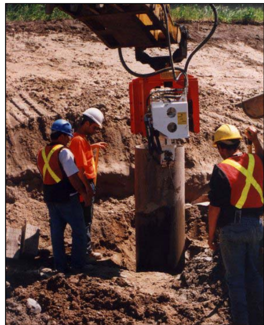
Figure 7.8 Alternative to pile driving (Photo #509)
