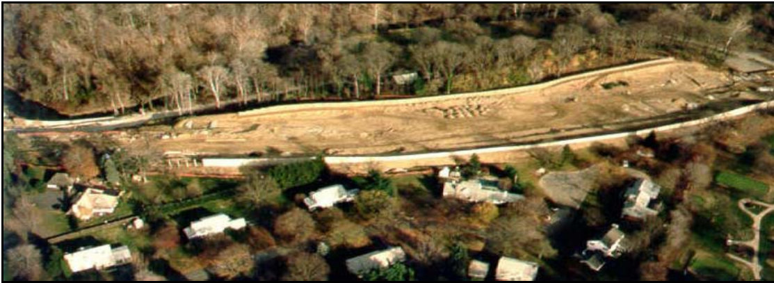
Figure 7.7 Early construction of noise barriers (Photo #447)
