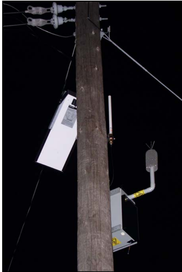
Figure 5.36 Permanent automated wireless noise monitoring system; note solar cell, antenna, transmitter, and microphone (Photo #48)
