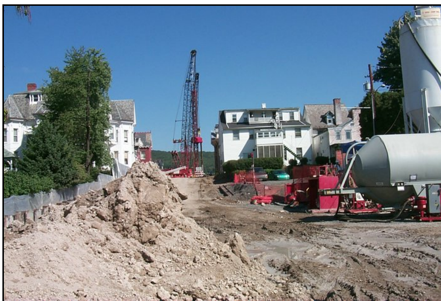
Figure 5.5 Several construction operations affecting noise levels at nearby residences (Photo #929)
