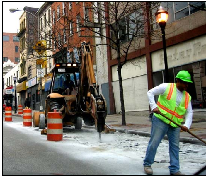
Figure 3.2 Construction in business district (Photo #714)
