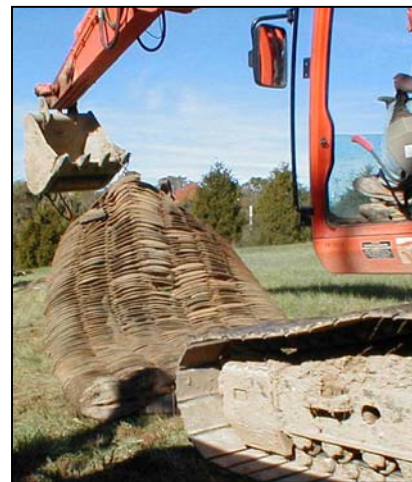
Figure 7.22 Blasting mats being placed into position (Photo #1341)
