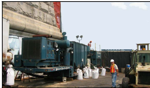
Figure 7.30 Use of existing structure and temporary plywood on chain link fence plus absorptive mats to shield recycling equipment (Photos #690, #390, #395 & #679)
