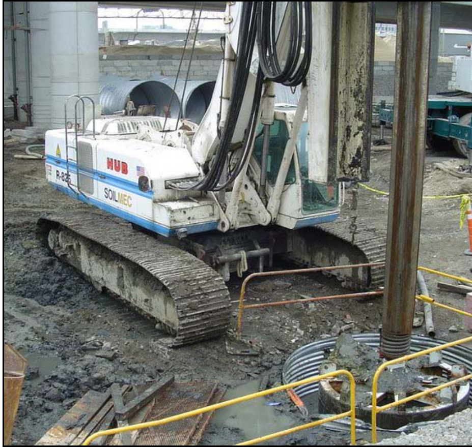
Figure 5.31 Stationary construction operation (Photo #123)
