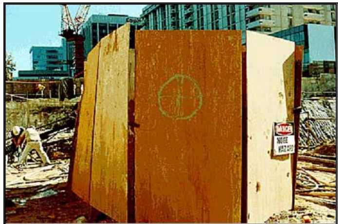
Figure 7.26 Temporary shielding of stationary equipment (Photo #1340)
