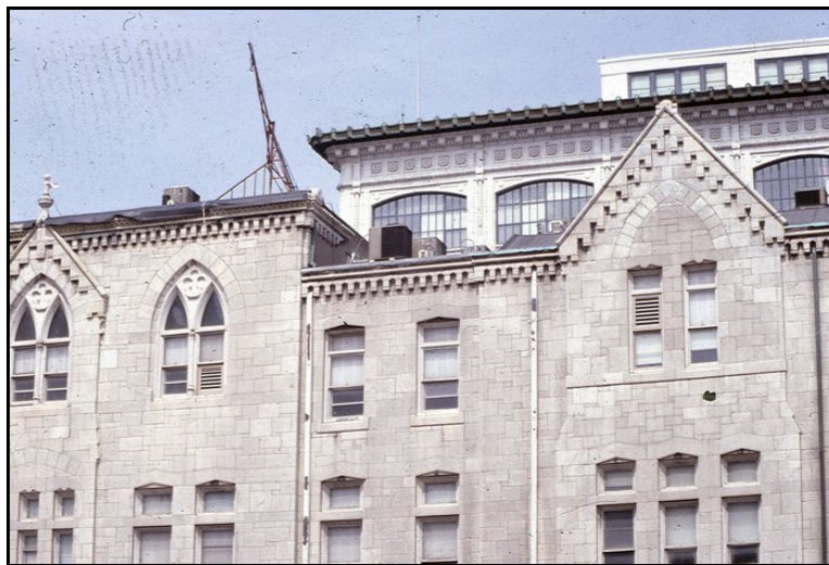
Figure 7.34 Installation of a complete air handling system and window treatments at urban school solely to abate construction noise due to future conversion of arterial to depressed expressway (Photos #1300, #1303 & #1304)
