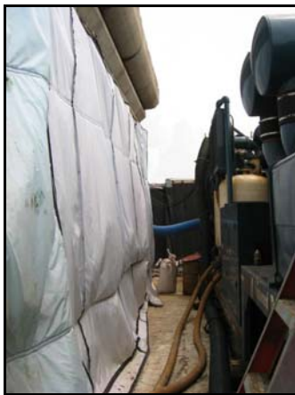
Figure 7.30 Use of existing structure and temporary plywood on chain link fence plus absorptive mats to shield recycling equipment (Photos #690, #390, #395 & #679)
