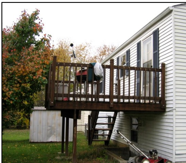
Figure 5.18 Measurement on a raised deck (Photo #1285)
