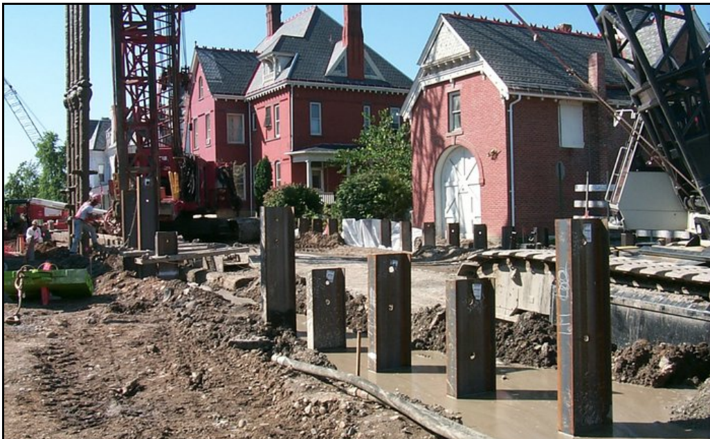
Figure 3.1 Construction in residential area (Photo #924)
