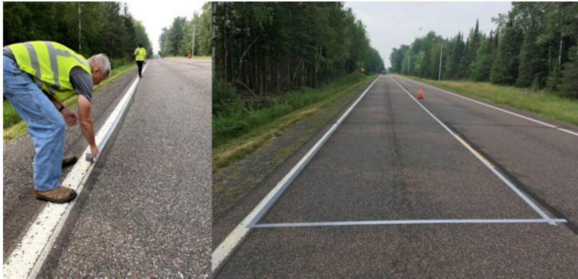
Figure 5.7. Taping of fog line prior to HFST installation (left); fully-taped lines (right)
