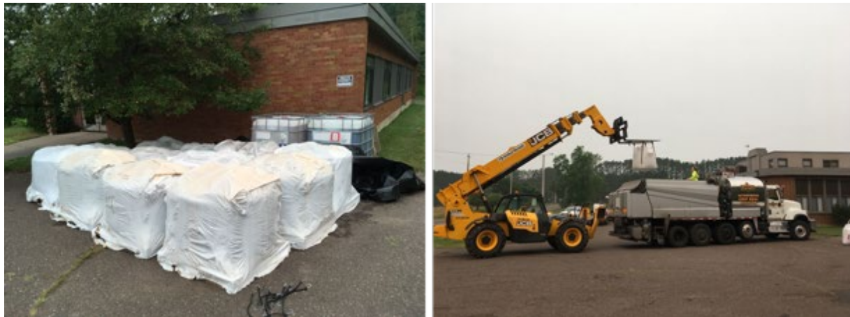
Figure 5.3. Staging area, showing super sacks of aggregate and totes containing two-part epoxy resin (left), and loading of aggregate for GSB-based pavement treatment (right).
