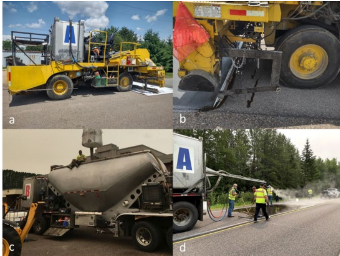
Figure 5.8. HFST equipment options: (a) automated HFST rig; (b) close up of resin and aggregate delivery end of automated HFST rig; (c) non-automated HFST rig showing loading of aggregate to hopper at project staging location; and (d) non-automated method for delivery and application of resin and aggregate from the non-automated HFST rig, showing installation of taconite HFST aggregate to Test Section 3. Images a and b courtesy of Fahrner Asphalt Sealers
