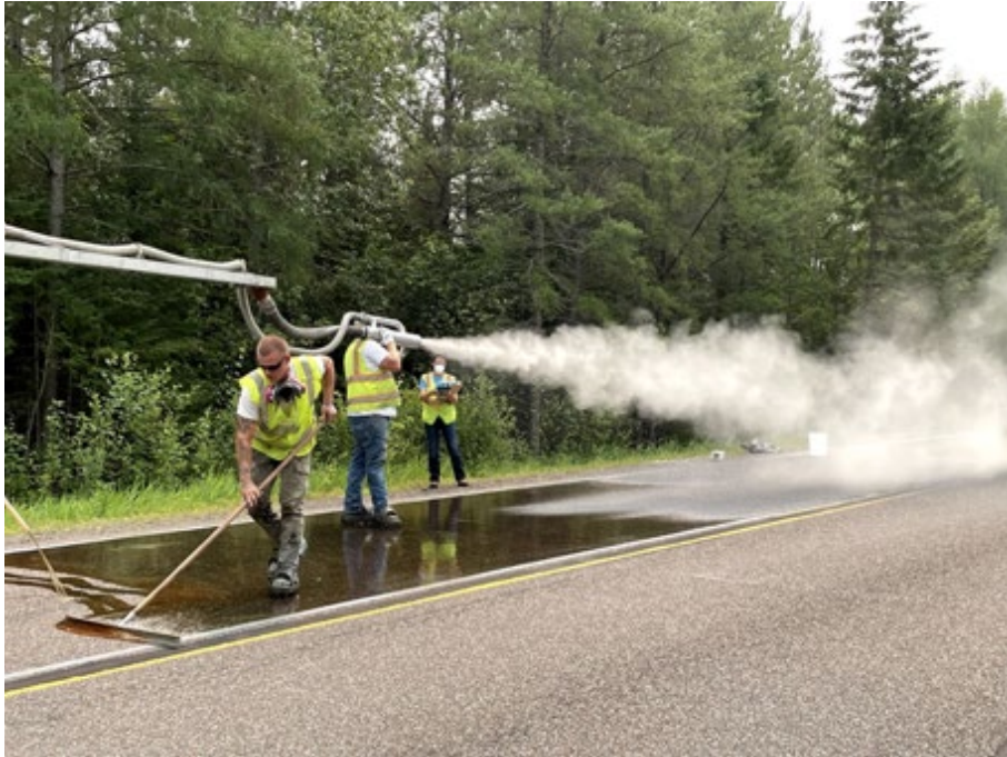
Figure 6.4. Dust monitoring by industrial hygienist upwind of HFST aggregate deployment.
