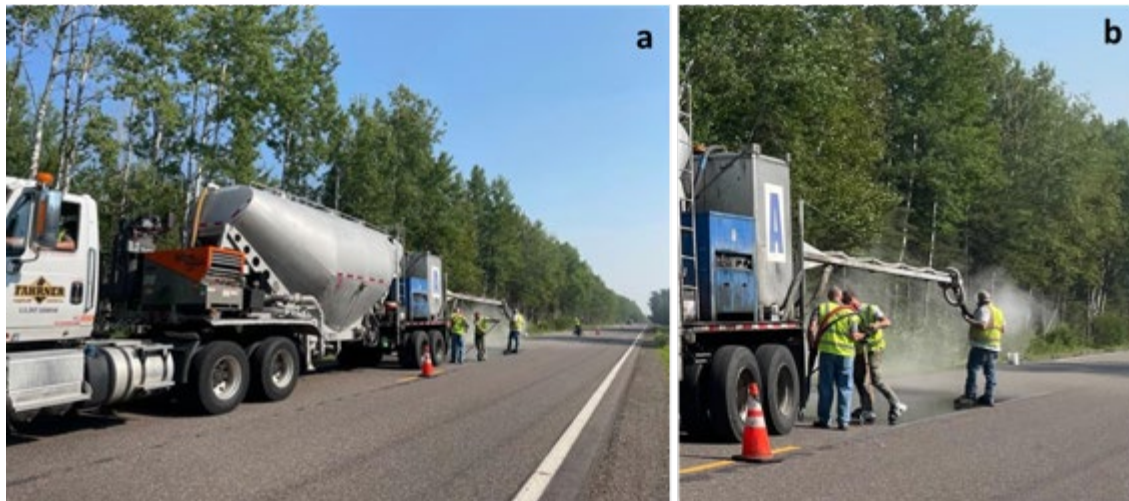
Figure 6.2. High friction rig (a); closeup of application hose (b) application process
