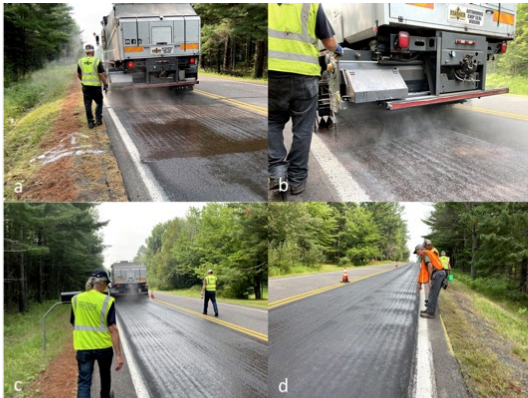
Figure 5.5. Installation of minus #8 Friction Seal: (a) start of installation; (b) close-up of spreader and deployment of GSB and aggregate; (c) freshly-installed; and (d) post-installation
