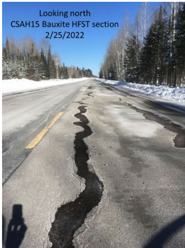
Figure 7.13. Photo showing potential relationship of pre-existing pavement cracking in “Control” pavement (left) to the losses in the HFST test section (right)
