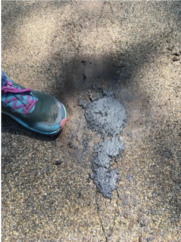
Figure 7.18. Core hole filled with the NRRI's rapid-setting repair compound
