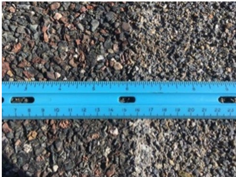
Figure 3.3. Closeup of existing pavement (left) and calcined bauxite treatment (right)
