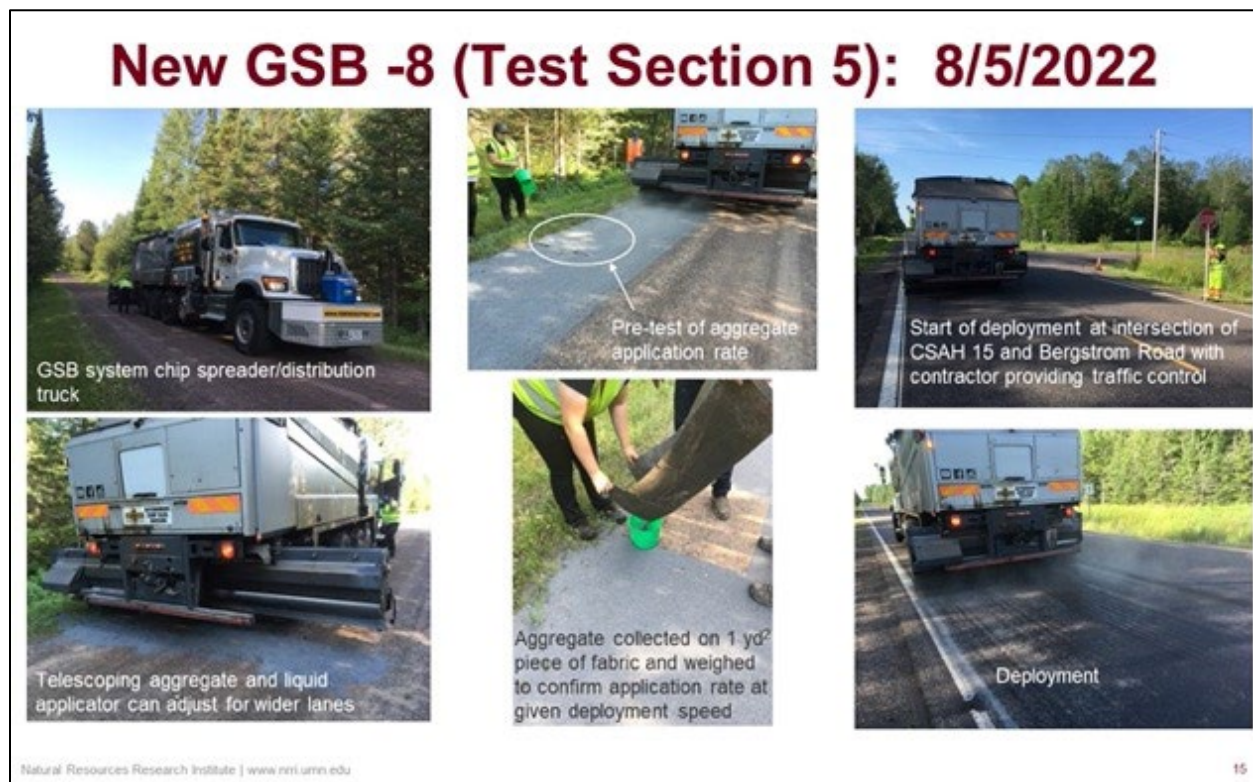
Figure 7.24. Installation of new GSB -8 (Test Section 5) on August 5, 2022
