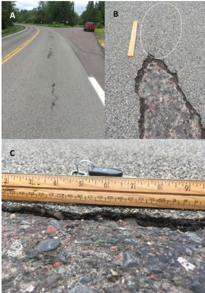
Figure 7.21. July 5, 2022, photos of losses in bauxite HFST installed in 2020: Looking south toward horizontal curve (A); closer view of HFST loss and visible faint cracks (B, circled); and close-up of underlying exposed asphalt pavement (C)
