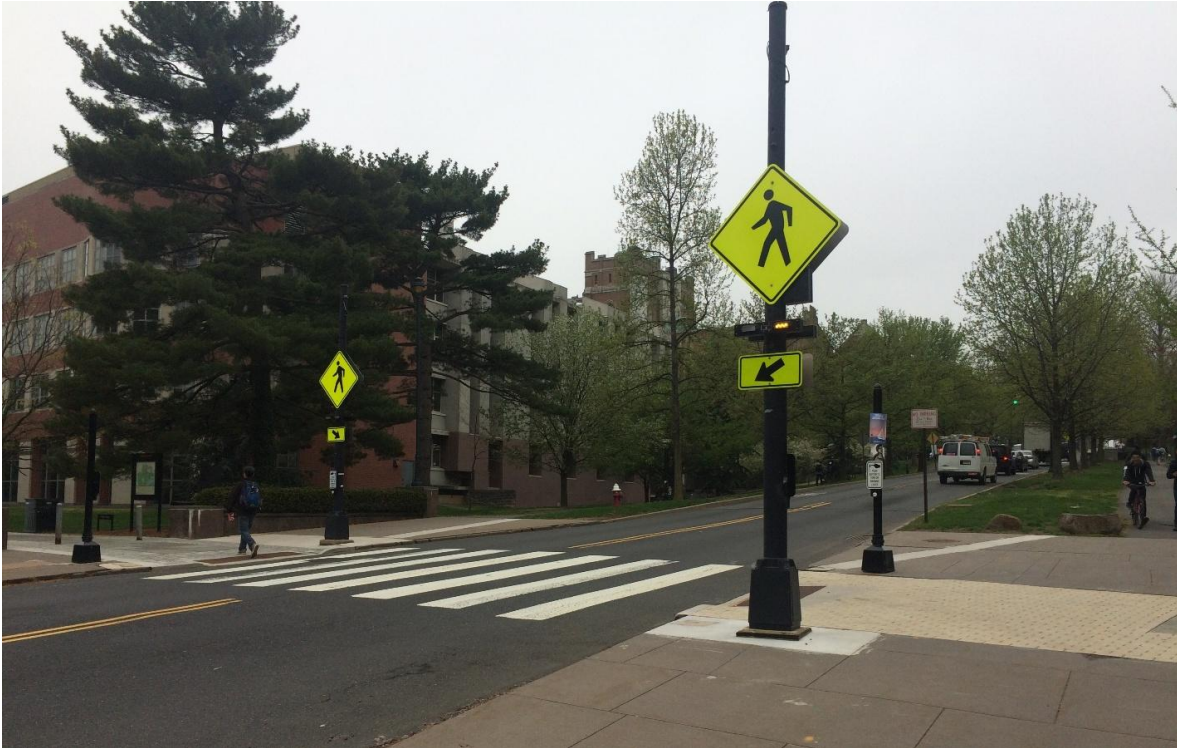
Figure 6.43. RRFB Installed at a Short Crosswalk
