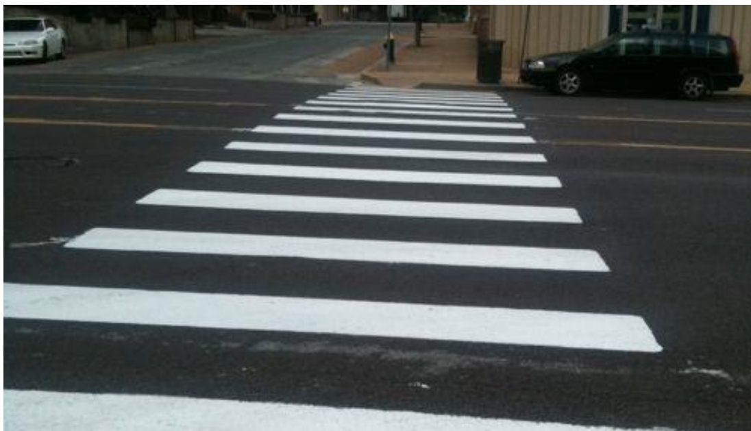
Figure 6.17 High Visibility Crosswalk (Continental/Zebra Design)
