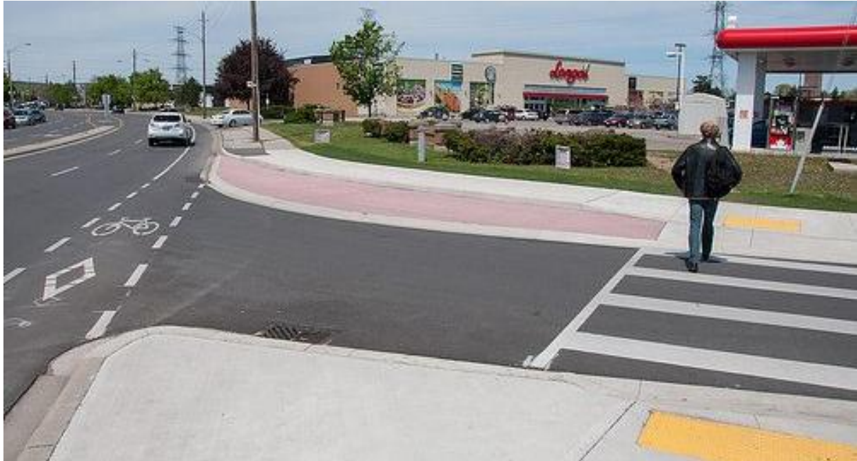
Figure 6.7 Curb Extension with Truck Apron – Right-Turn Curve
