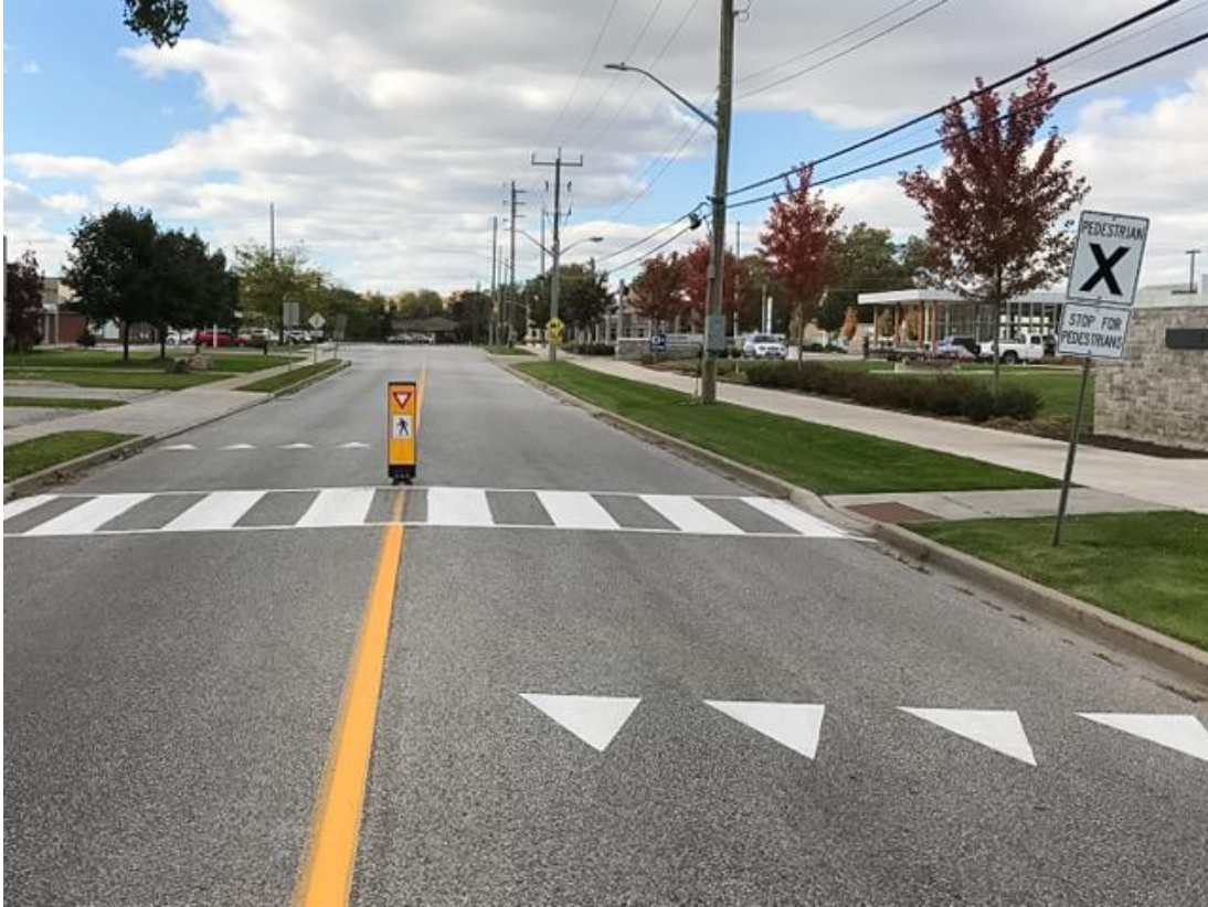
Figure 6.18 High-Visibility Crosswalk (Ladder-Style Design with Sharks Teeth)
