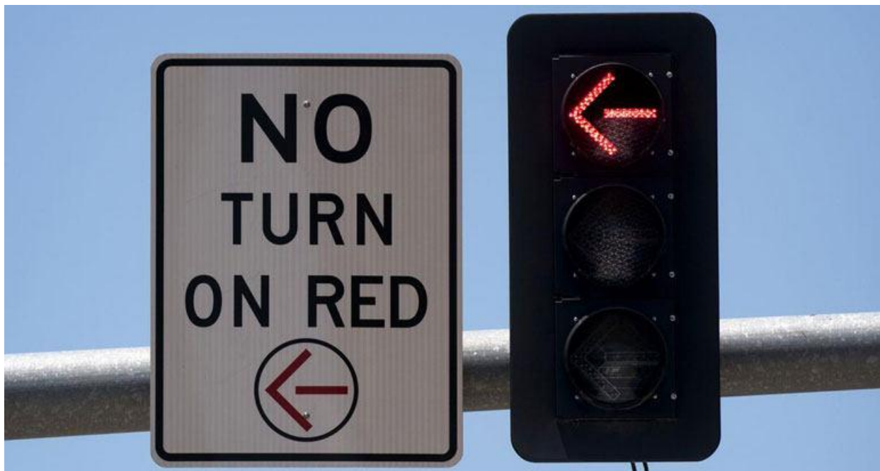
Figure 6.12 Left-Turn Signal Head and Sign for Control Over Left-Turn Phasing
