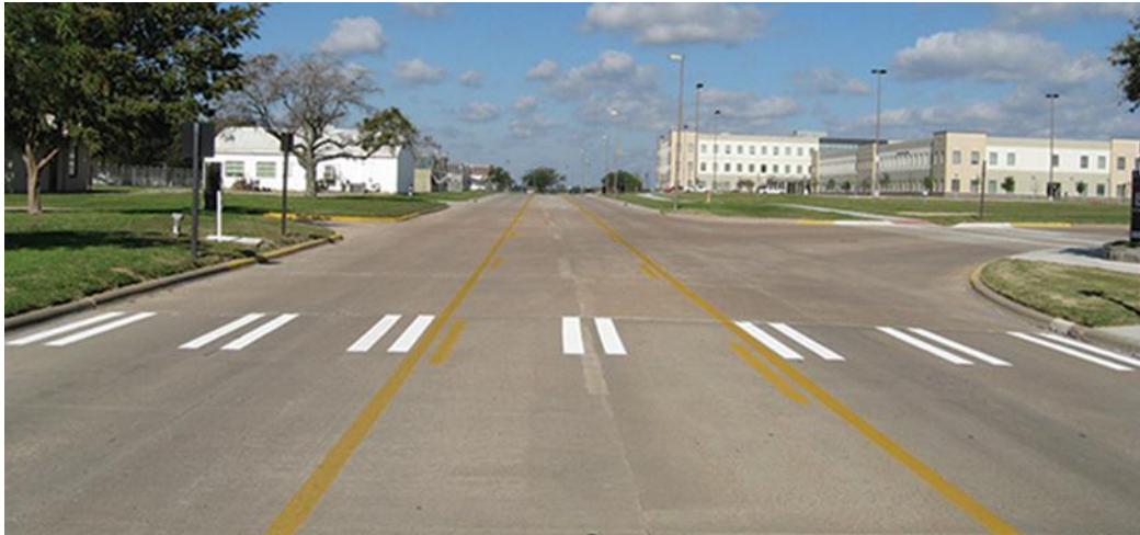
Figure 6.16 High-Visibility Crosswalk (Bar Pair/Piano Key Design)
