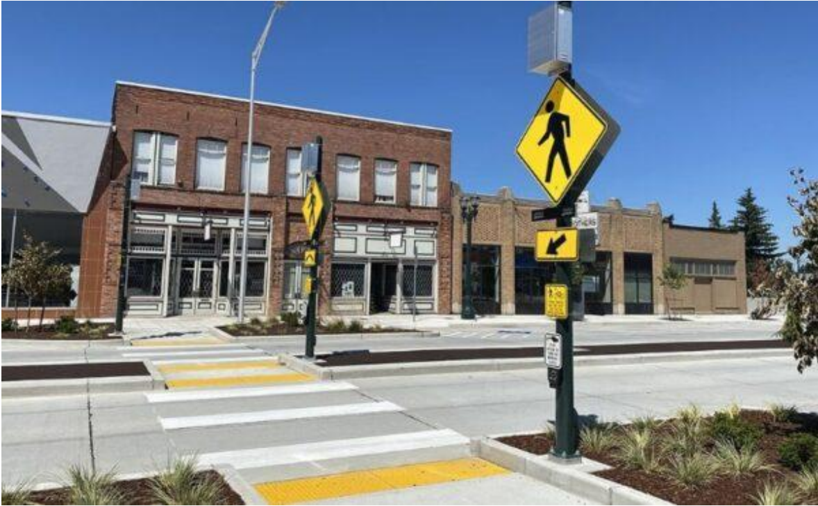
Figure 6.44. RRFB Installed with a Median Island
