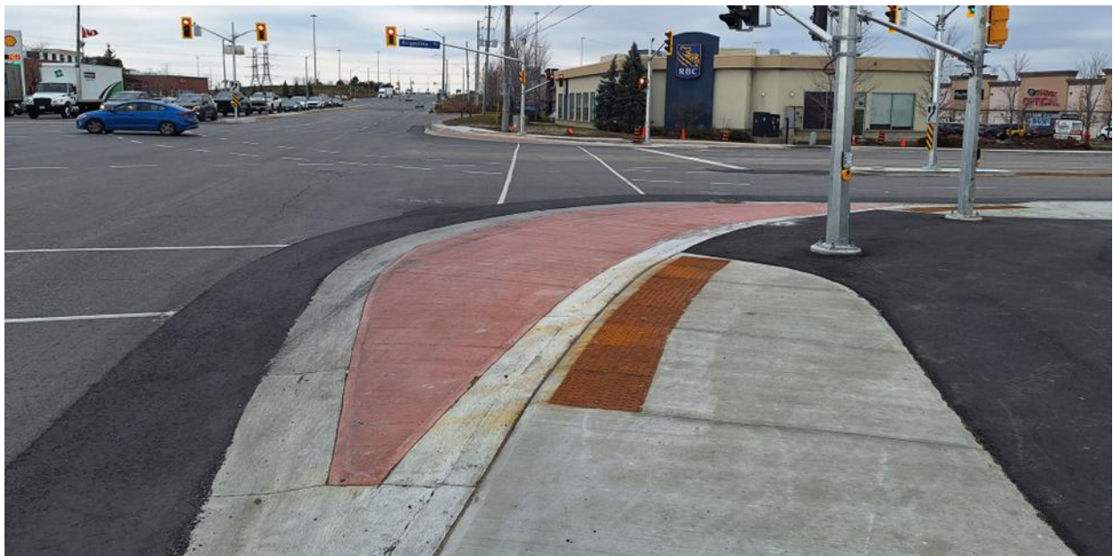
Figure 6.5 Curb Extension with Truck Apron
