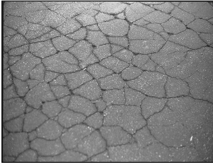
Figure C5 Illustration for Severe and Extensive Cracking on Asphalt Pavements
