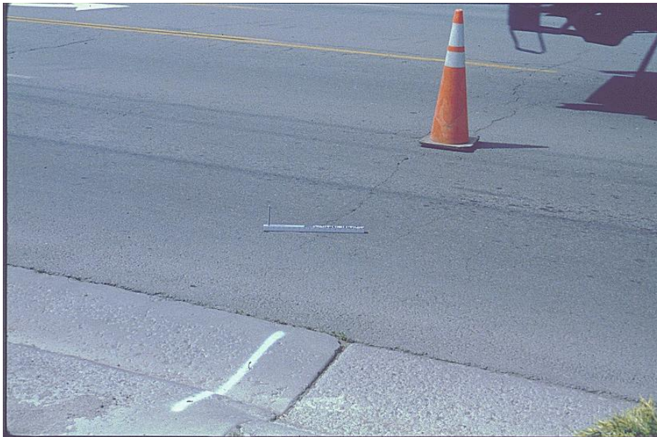
Figure C4 Illustration for Moderate Cracking on Asphalt Pavements
