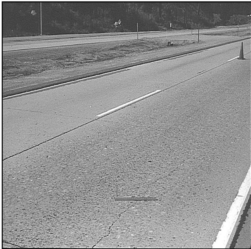
Figure C6 Illustration for Light Cracking on PCC Pavements
