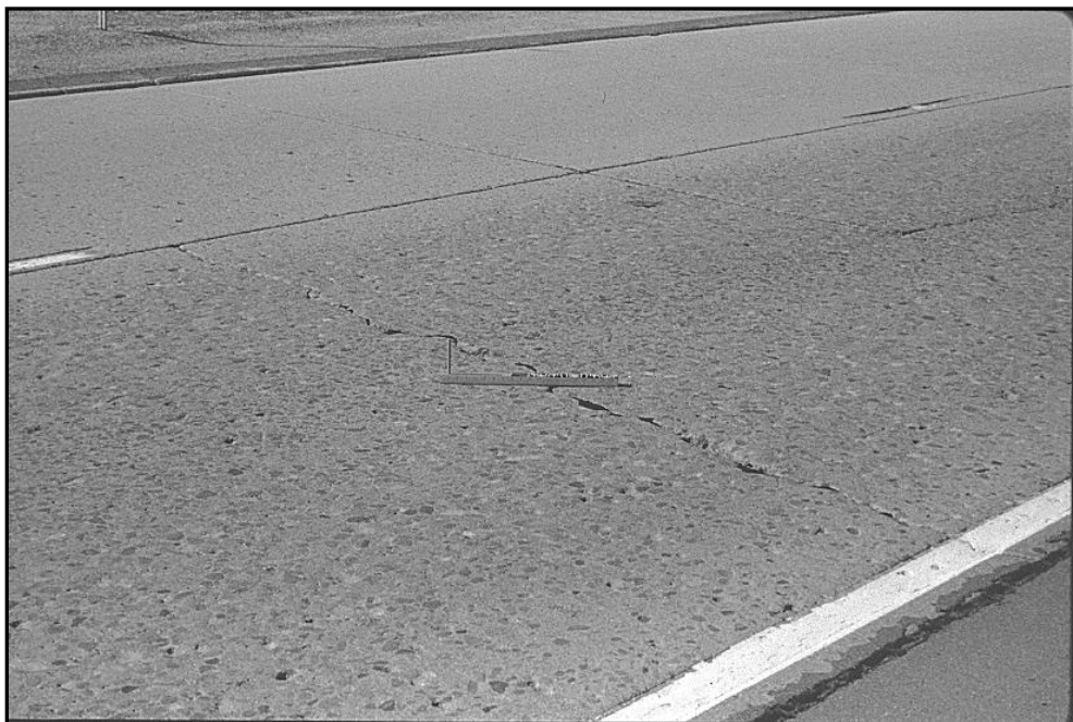
Figure C7 Illustration for Moderate Cracking on PCC Pavements
