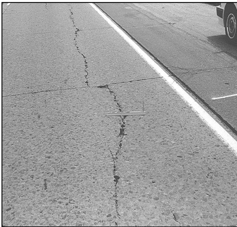
Figure C8 Illustration for Severe Cracking on PCC Pavements
