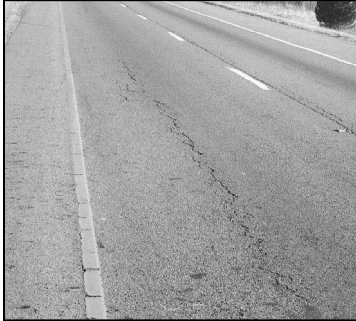
Figure C3 Illustration for Light Cracking on Asphalt Pavements
