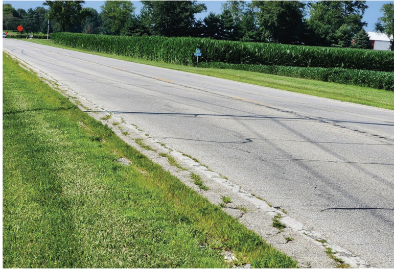
Figure 4.6 Vegetation growing in between rumble strips: US 231.
