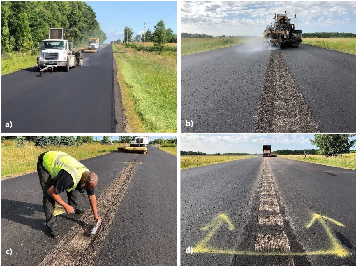
Figure 5.9: Installation of CLRS Including Milling Operation (a and b), Checking Dimensions (c), and Cleaned Surface. WisDOT Sinusoidal CLRS are Shown (d).
