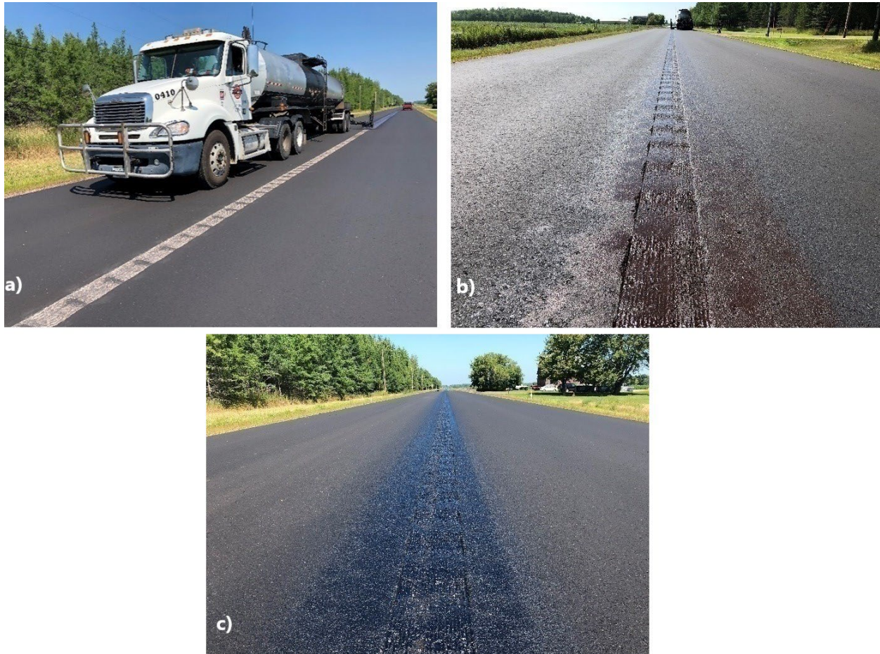
Figure 5.10: RPE Application Over CLRS, Centerline Application Alternative (a), Freshly Applied RPE (b), and Fully Dried Ready for Striping (c).
