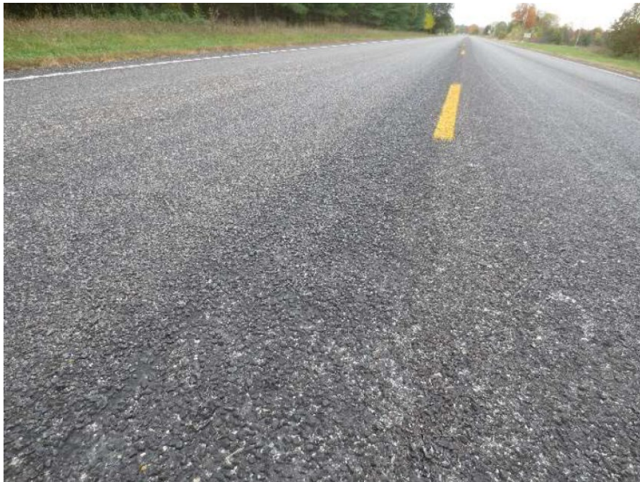
Figure 2.19: Example of a Sinusoidal CLRS With Chip Seal Application. From (Donavan, Janello, Rochat, & McKenna, 2024).
