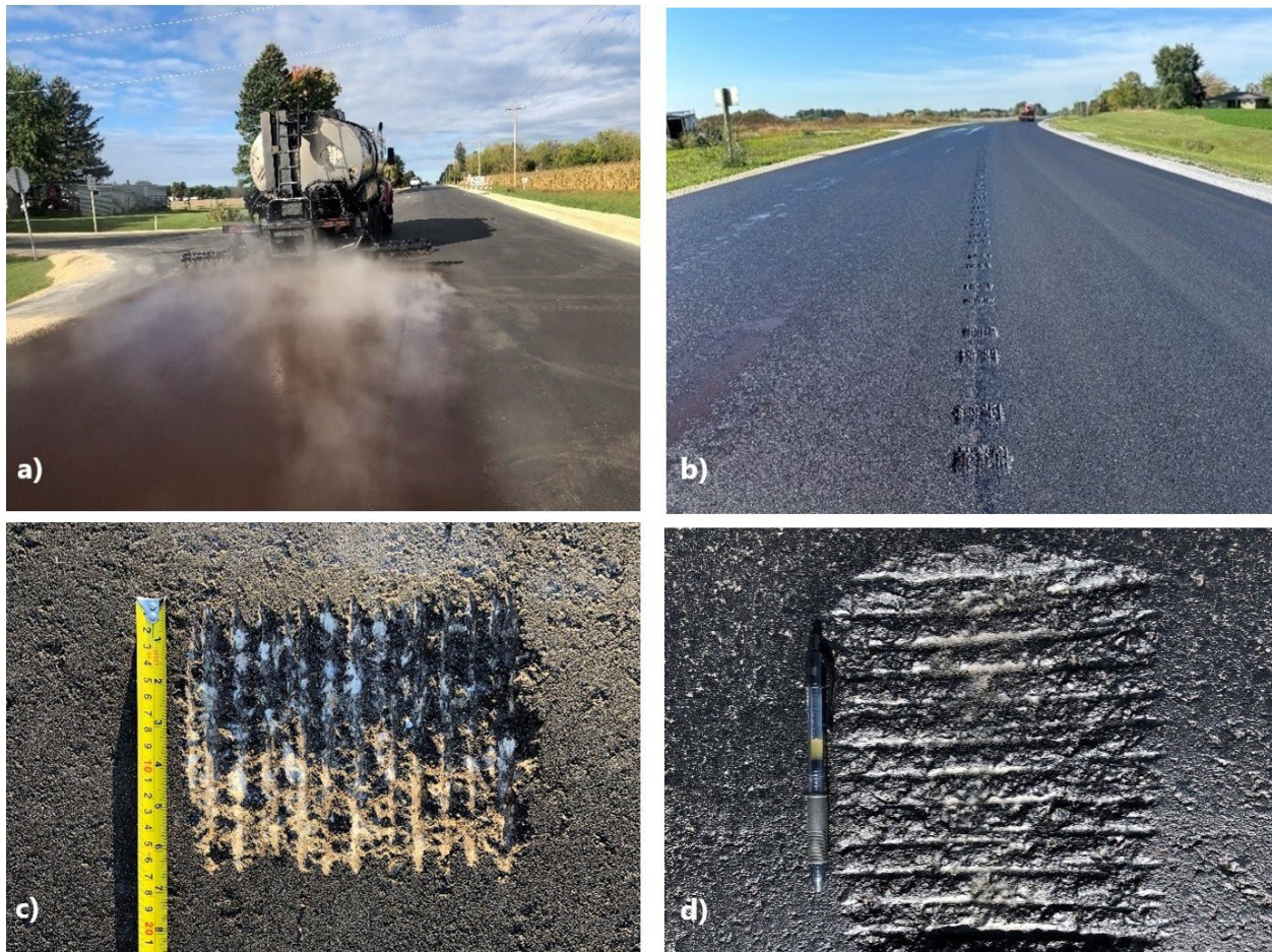
Figure 5.11: RPE Application Utilizing Full Lane Width Alternative (a). Photo (b) is After Final Pass Before RPE has Fully Dried. Photo (c) is CLRS Before RPE, Photo (d) is CLRS Following RPE, Note the Macro-Texture of the Underlying Surfacing, Characteristic of a Penetrating Emulsion Treatment.
