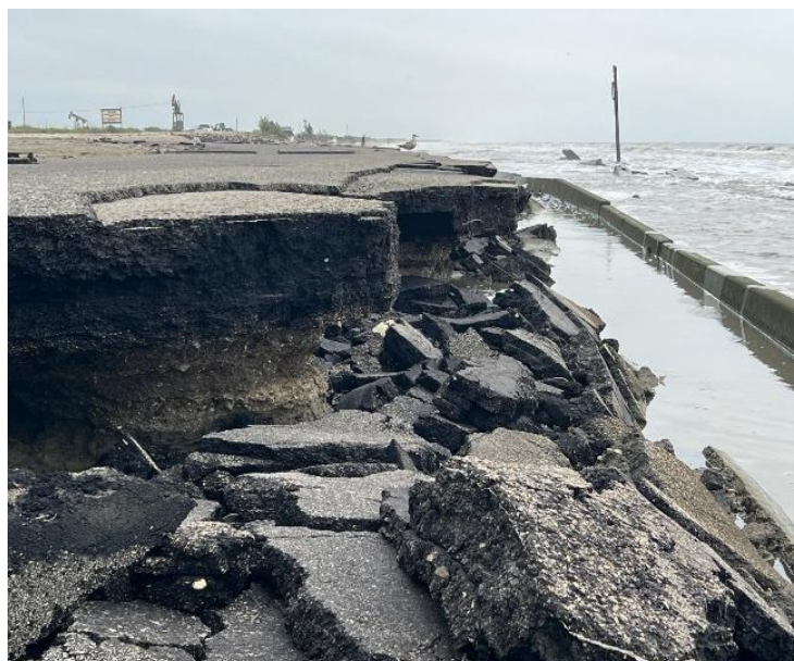
Figure 1. Highway embankment slope failure in a coastal area
