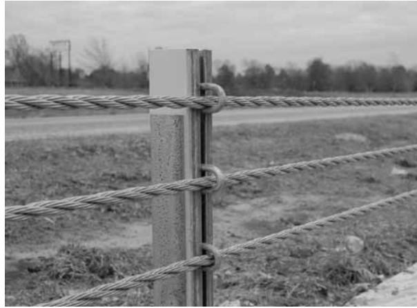
Figure 7. Cable barrier guardrail
