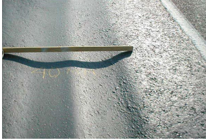
Figure 3. Rutting failure in flexible pavements
