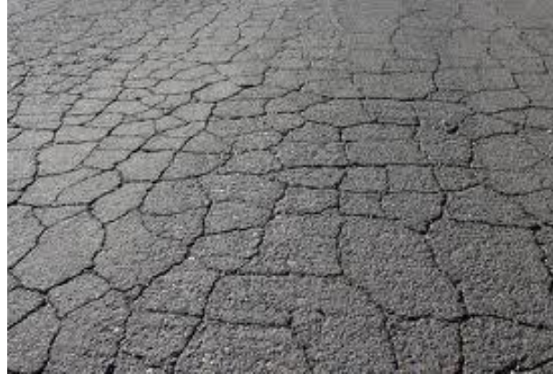
Figure 2. Fatigue cracking in flexible pavement [17]
