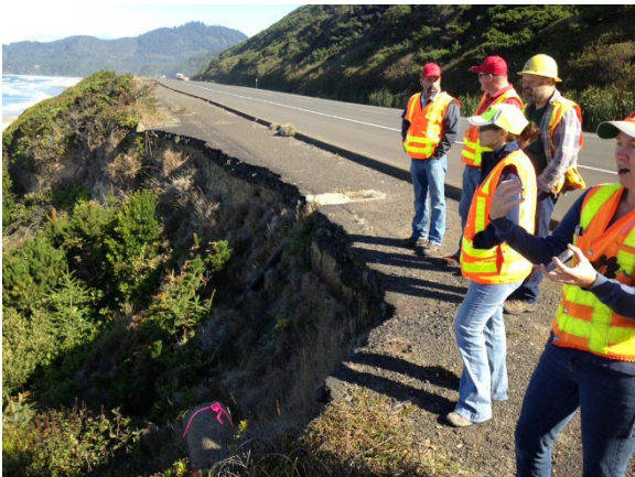
Figure 2. Evidence of road erosion (Source: Oregon DOT).
