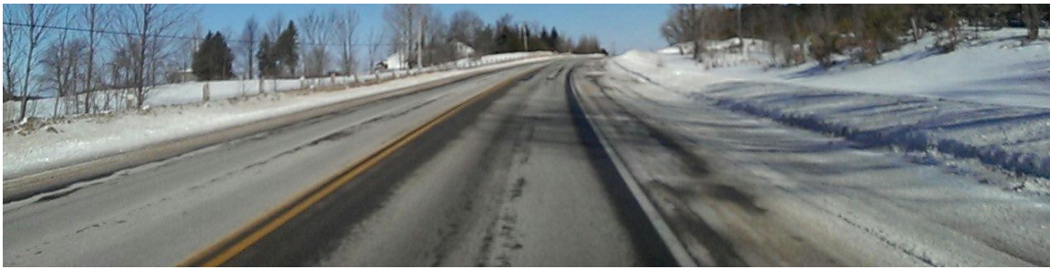
Figure 21 - Bare RSC Covered with Dried Residual Salt
