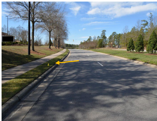
Figure 3. Facing west trajectory view, looking at roadway departure point as indicated by the yellow cone
