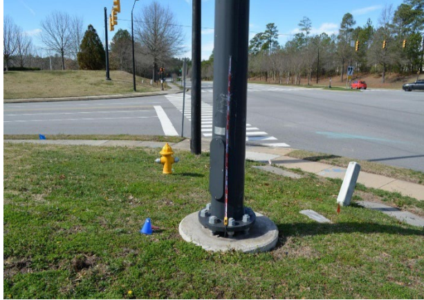
Figure 10. Facing west, viewing the traffic control post and Event 7
