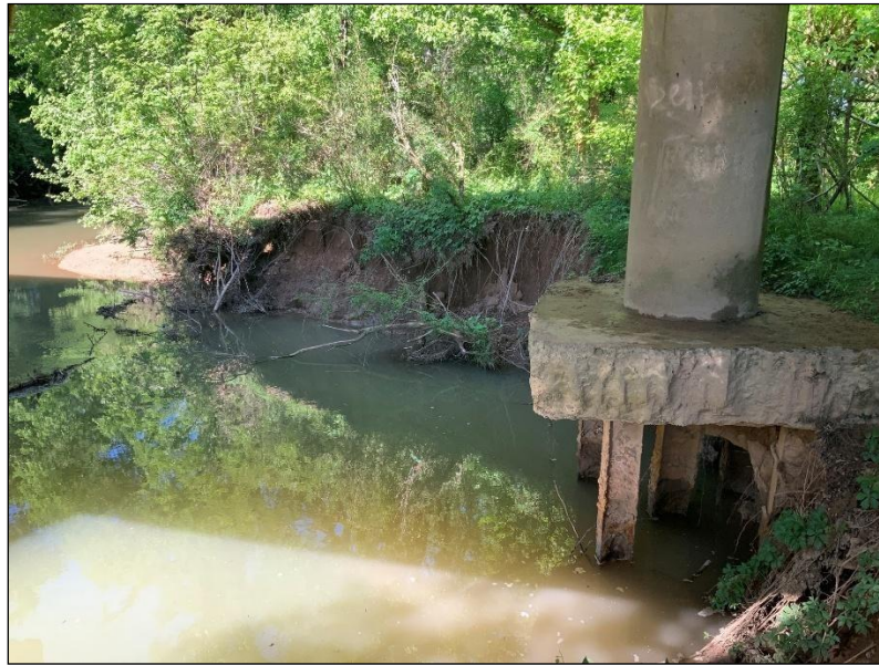
Figure 1. Photo. Natural loss of sediment from base of bridge bent or pier due to scouring.
