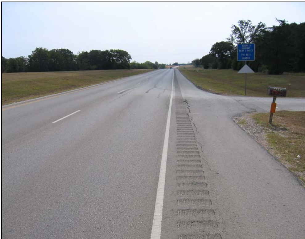
Figure 1.15. Cracking in SH 47 SB from STA 2155.94 to 2156.92.
