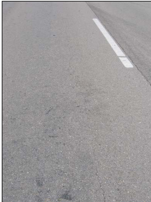
Figure 1.9. Cracking in SH 47 OL from STA 2145.23 to 2145.43 (Joint crack from 2144.80 to 2145.70 also visible).
