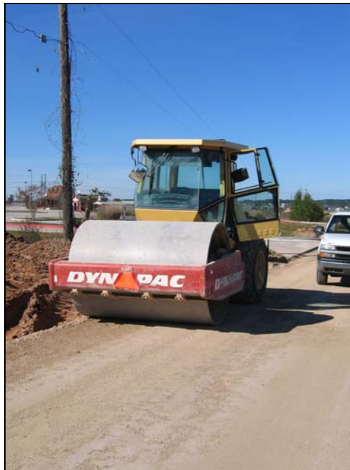
Figure 3.5. Microcracking IH 45 SB OL on December 7, 2005.
