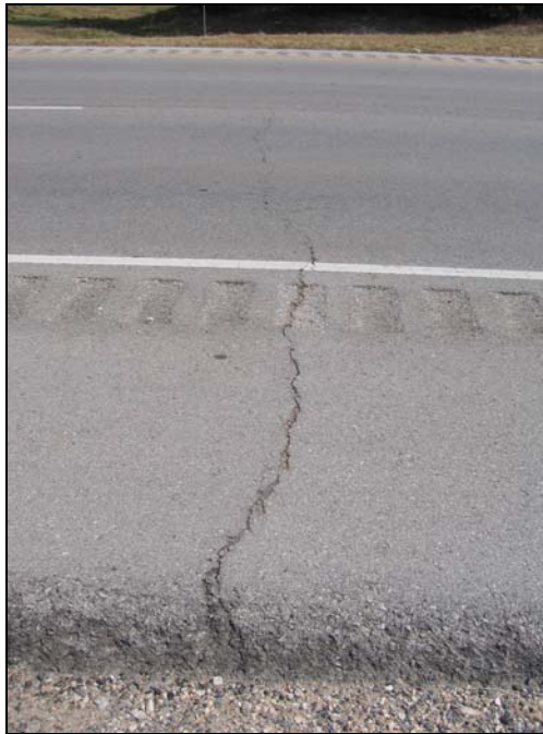
Figure 1.13. Transverse Cracking in SH 47 SB at STA 2153.87.
