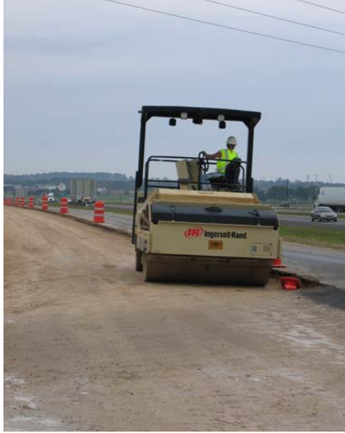
Figure 3.4. Microcracking IH 45 SB OL on December 6, 2004.
