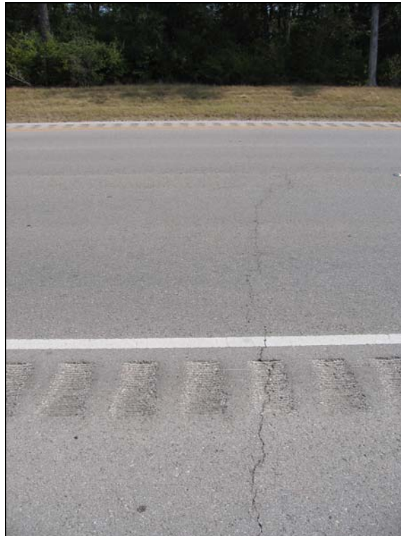
Figure 1.7. Transverse Crack on SH 47 SB at STA 2143.50.
