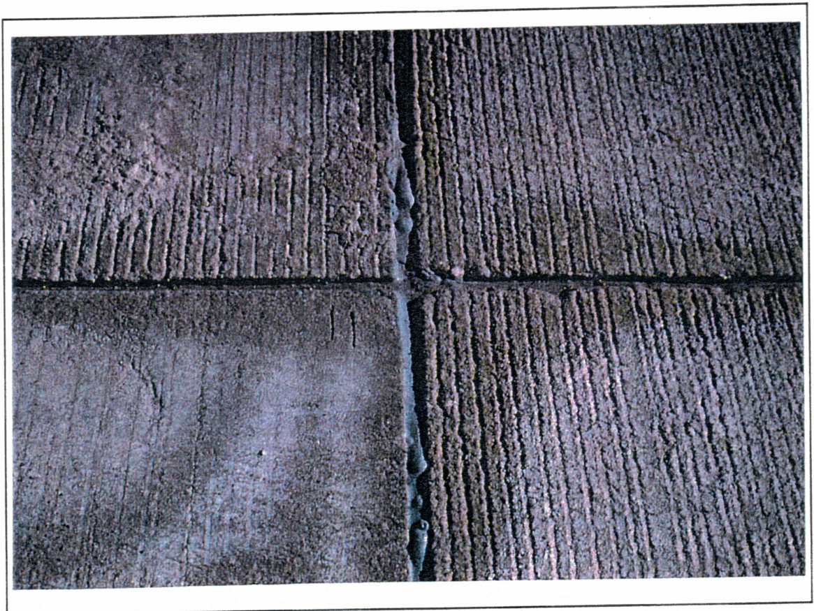
Figure 7. Bubbles in sealant
