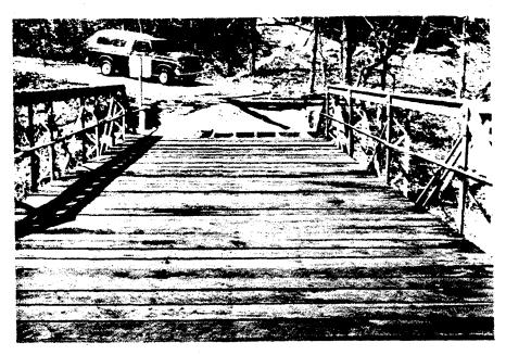
Figure 7-2 Plank Deck
