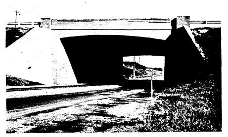
Figure 9-20 Typical Single Span Rigid Frame Bridge
