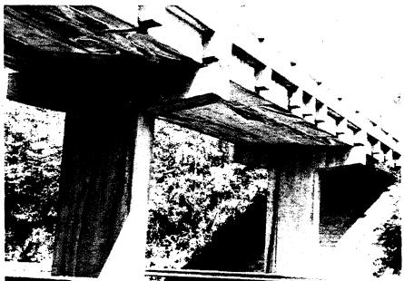
Figure 9-28 Leaking Joints Between Adjacent Boxes
