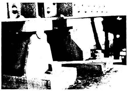
Figure 11-2 Fixed and Expansion Bearings
