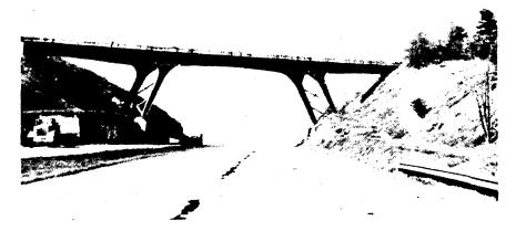
Figure 10-21 Rigid Frame Bridge with Only Two Frames
