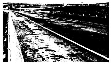
Figure 7-1 Environmental Damage to a Bridge Deck
