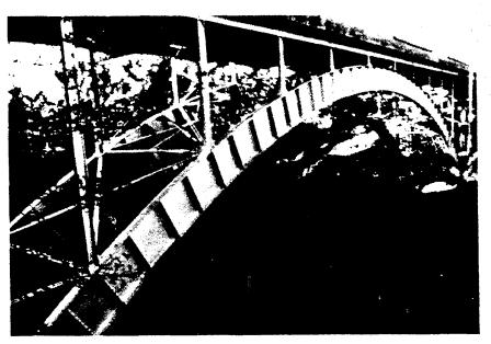
Figure 10-16 Solid Ribbed Deck Arch
