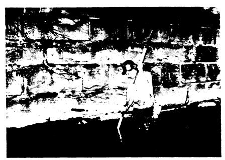
Figure 17-2 Wading Inspection
