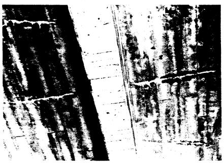
Figure 4-16 Cracking in Concrete (Note Efflorescence)
