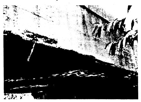
Figure 9-10 Exposed Reinforcement in a Through Girder
