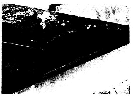
Figure 16-6 Exposed Reinforcing Bars on Bottom Surface of Concrete Pier Cap Beneath Expansion Dam (Note Also Corrosion and Paint Failure on Steel Girder and Cross Frame)
