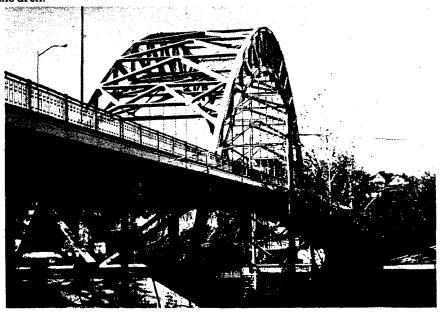
Figure 10-17 Braced Ribbed Through Arch
