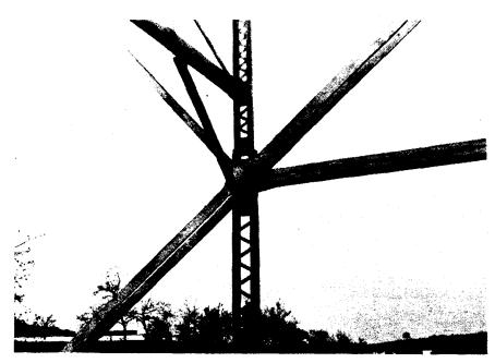
Figure 6-23 Pin-Connected Truss Members
