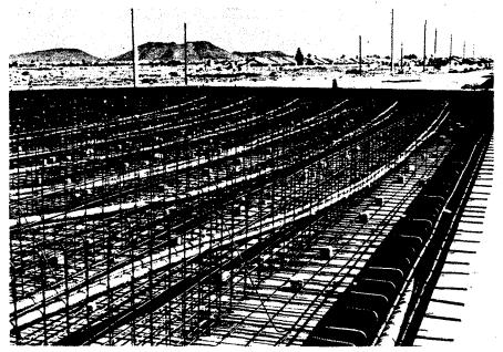
Figure 9-38 At-Grade Formwork With Posttensioning Ducts
