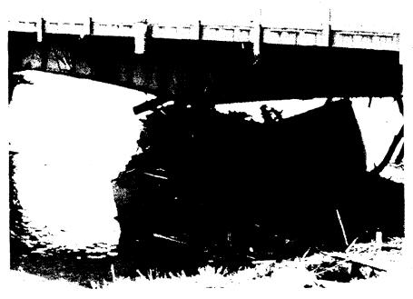
Figure 17-6 Movement of a Substructure Unit
