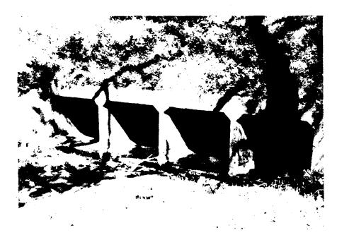
Figure 19-4 Cast-in-Place Concrete Multicell Box Culvert
