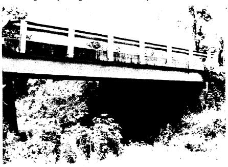
Figure 10-1 Simple Span Rolled Multi-Beam Bridge
