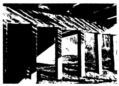
Figure 6-14 Concrete Pile Bent
