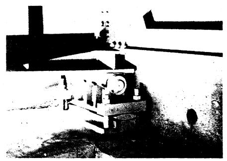
Figure 11-13 Restraining Bearing
