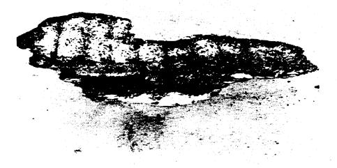
Figure 4-22 Spall (Pothole)
