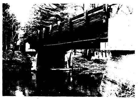
Figure 8-1 Elevation View of a Glulam Multi-Beam Bridge
