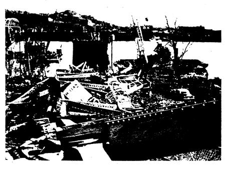
Figure 1-1 Collapse of the Silver Bridge
