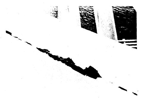
Figure 16-8 Edge Failure on Painted Steel Beam
