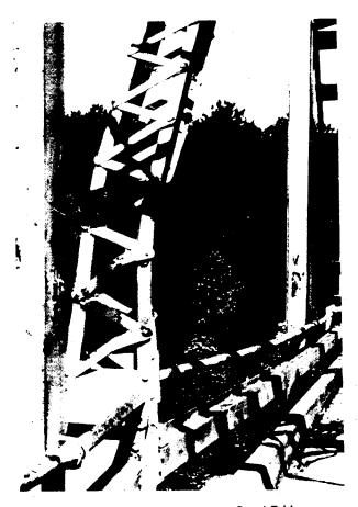
Figure 4-27 Collision Damage on a Steel Bridge
