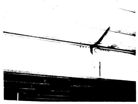
Figure 11-9 Pin and Link Bearing
