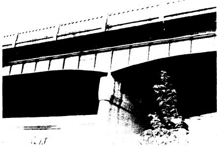
Figure 10-3 Web Stiffeners on a Fabricated Multi-Girder Bridge
