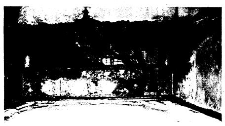
Figure 10-2 Corroded Shear Zone on a Rolled Multi-Beam Bridge
