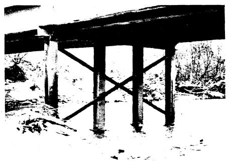
Figure 12-14 Corrosion and Debris at a Steel Pile Bent
