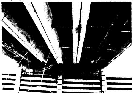
Figure 9-11 Typical Channel Beam Bridge
