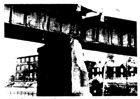
Figure 12-12 Pier Movement and Superstructure Damage Due to Scour
