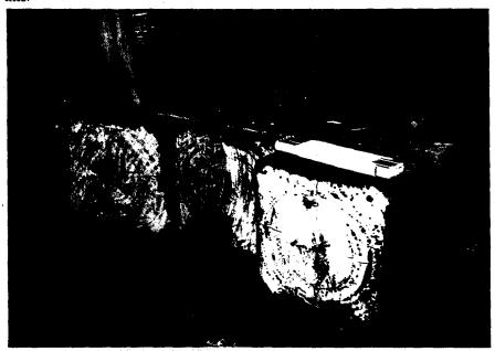
Figure 16-1 Bridge Timber Member Showing Penetration Depth of Preservative Treatment
