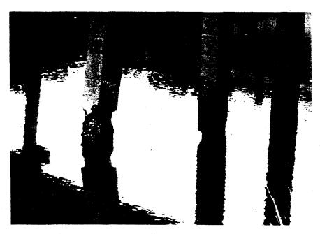
Figure 17-7 Spalled Concrete Piles at Low Water Level
