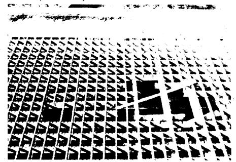
Figure 7-6 Broken Members on an Open Steel Grid Deck
