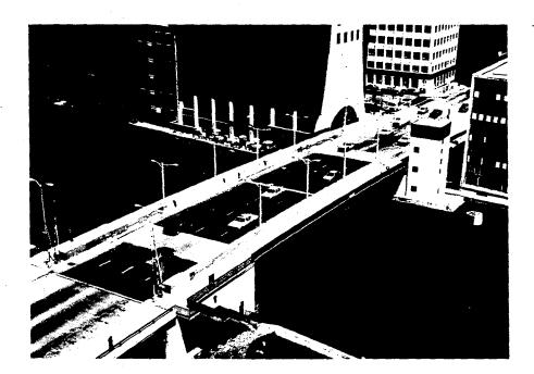
**Figure 20-9** A Simple Trunnion (Chicago Type) Double-Leaf Bascule Bridge Over the Chicago River
