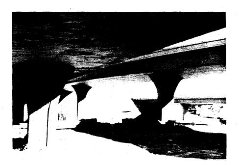
Figure 9-39 Box Girder Bridge Constructed Using At-Grade Forming
