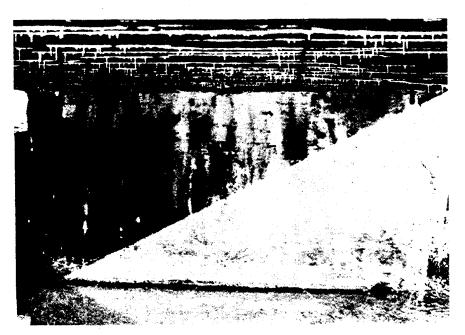
Figure 4-23 Efflorescence
