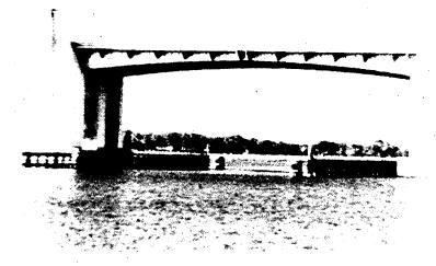
Figure 20-6 Double-Leaf Bascule Bridge; There is a "Center Break in Floor" at the Centerline of Bascule Span
