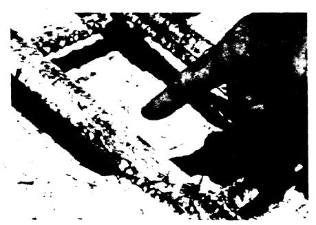
Figure 16-5 Corroding Concrete Reinforcing Bar
