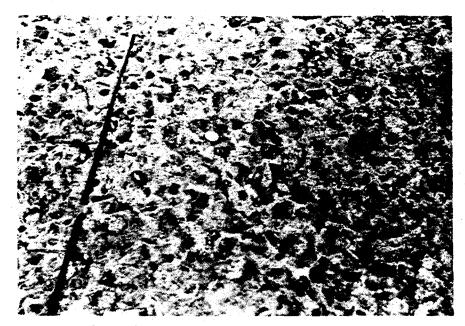
Figure 4-20 Severe Scaling
