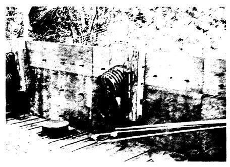
Figure 9-35 Formwork with Posttensioning Ducts Located
