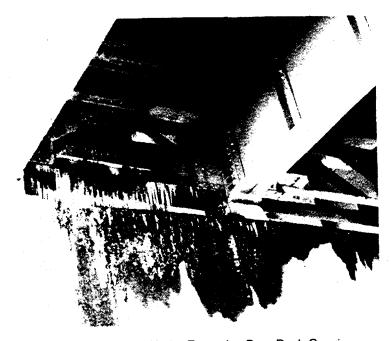
Figure 16-9 Water and Salt Runoff Under Expansion Dam Deck Opening
