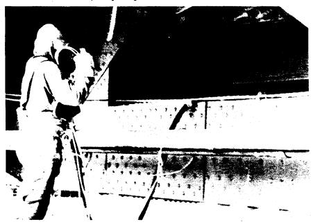
Figure 16-7 Open Nozzle Dry Abrasive Blast Cleaning
