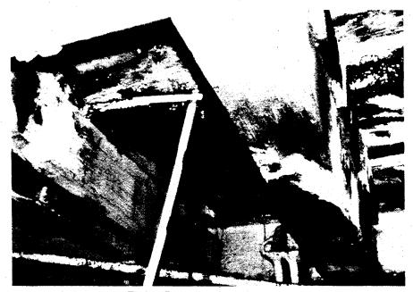
Figure 8-4 Decay in a Timber Beam
