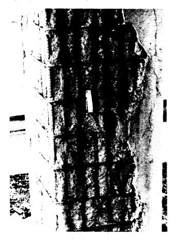
Figure 4-21 Delamination and Spall
