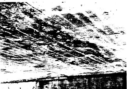
**Figure 9-3** Delamination and Efflorescence With Rust Stains on Slab Underside
