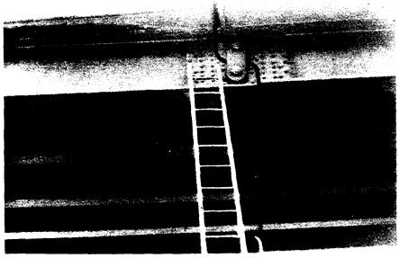
Figure 6-27 Pin and Hanger Connection
