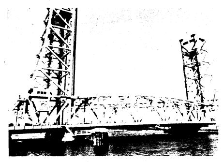
Figure 20-16 Vertical Lift Bridge with Power and Drive System on Towers
