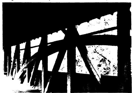
Figure 8-8 Inside View of a Covered Bridge with a Burr Arch-Truss
