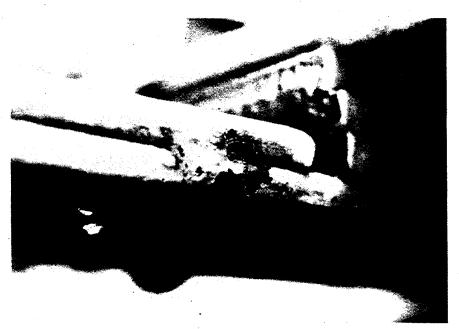
Figure 6-26 Close-Up of Tack Weld on a Riveted Built-Up Truss Member
