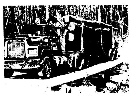
Figure 8-10 Stressed Deck Bridge Carrying a 90,000 Pound Logging Truck (Source: Barry Dickson, West Virginia University)
