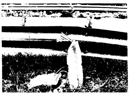
Figure 7-18 Approach Guardrail Collision Damage
