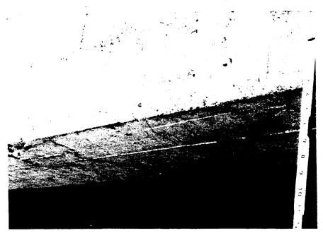
Figure 9-6 Flexure Cracks on a Tee Beam
