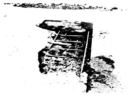
Figure 7-5 Pothole Showing Primary Deck Reinforcing Steel Perpendicular to Traffic
