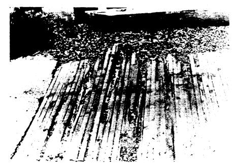
Figure 7-4 Wear and Weathering on a Timber Deck
