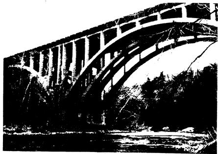
Figure 6-5 Concrete Arch Bridge
