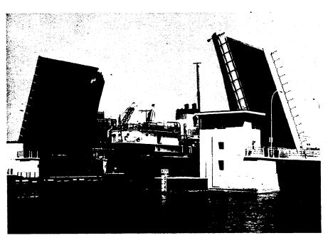
Figure 20-8 Double-Leaf Rolling Lift; the Leaves Roll Away from the Channel While the Moving Leaves Rotate Open
