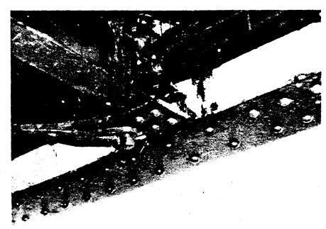
Figure 10-8 Lateral Bracing Connection on a Through Girder Bridge
