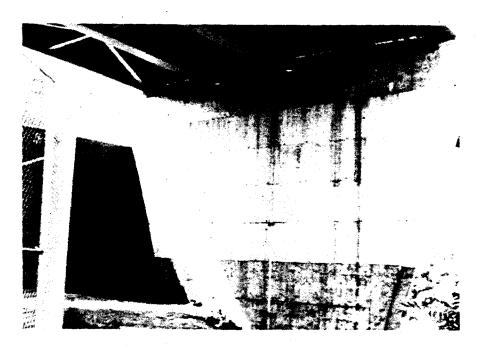
Figure 16-4 Anti-Graffiti Coating on Lower Area of Bridge Piers
