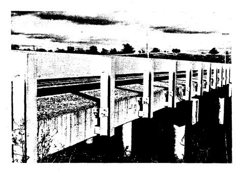
Figure 9-23 Typical Prestressed Slab Beam Bridge
