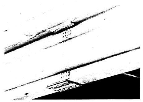
Figure 6-28 Bolted Field Splice
