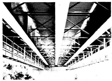
Figure 5-15 Inspection Catwalk
