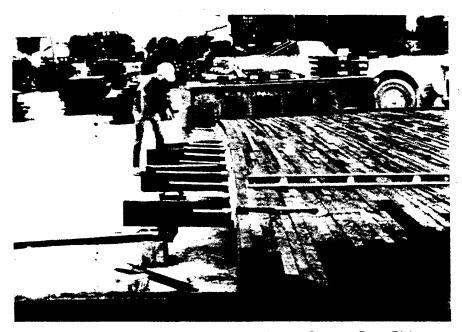
Figure 8-9 Stressed Deck Section Being Fabricated (Source: Barry Dickson, West Virginia University)
