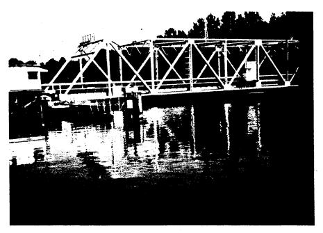
Figure 20-4 Swing Span with Operator's House on Approach at Left and Control Cabinet on Swing Span at Right
