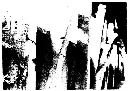
Figure 8-7 Collision Damage on a Timber Truss
