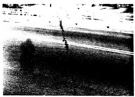
Figure 7-13 Asphalt Wearing Surface Over an Expansion Joint
