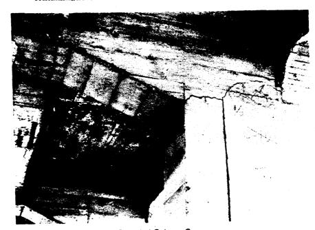
Figure 9-16 Diagonal Crack in Spandrel Column Cap
