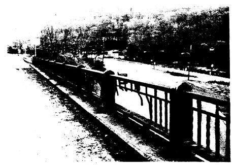
Figure 7-17 Damaged Steel Post Bridge Railing
