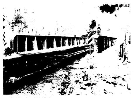
Figure 10-7 Through Girder Bridge
