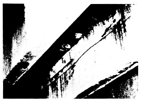
Figure 8-3 Horizontal Shear Crack in a Timber Beam
