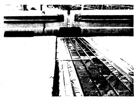
Figure 7-19 Heaving of the Approach Pavement
