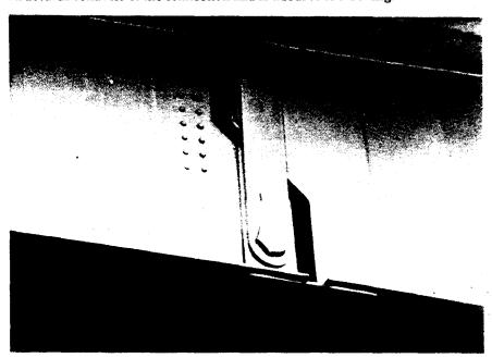
Figure 10-6 Two-Girder Bridge With a Pin and Hanger Connection
