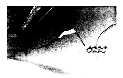
Figure 18-5 Girder Fracture Initiated at Plug Welded Bolt Hole
