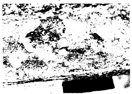
Figure 16-18 Color of Oxide Film is Critical in the Inspection of Weathering Steel; Dark Black Color is an Indication of Non-Protective Oxide
