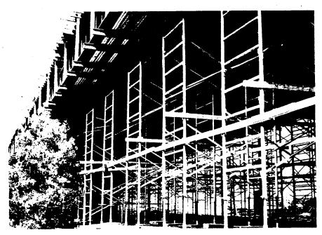
Figure 9-37 High Level Formwork Support Scaffolding
