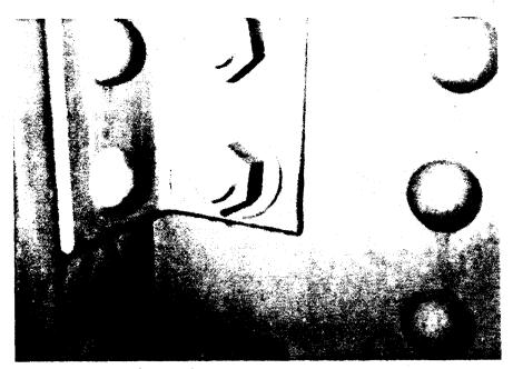
Figure 18-11 Cracked Stringer Connection Angle
