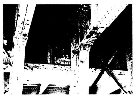
Figure 16-15 Paint Peeling from Steel Bridge Members
