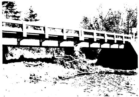
Figure 9-4 Multi-Span Tee Beam Bridge
