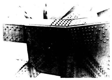
Figure 6-25 Shop Rivets and Field Bolts
