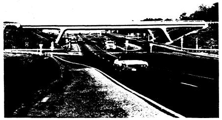
Figure 10-19 Typical Rigid Frame Bridge
