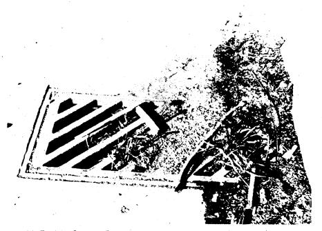
Figure 7-14 Partially Clogged Drainage Inlet
