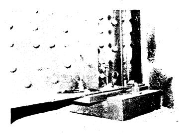
Figure 11-4 Lubricated Steel Plate Bearing
