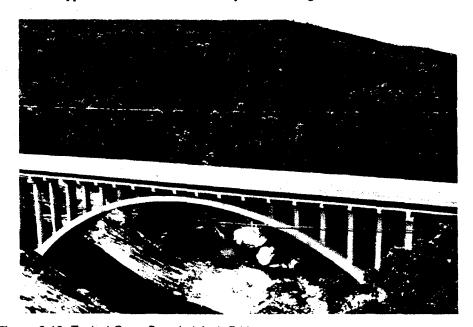
Figure 9-13 Typical Open Spandrel Arch Bridge
