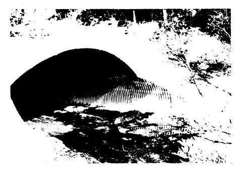
Figure 19-1 Steel Arch Culvert
