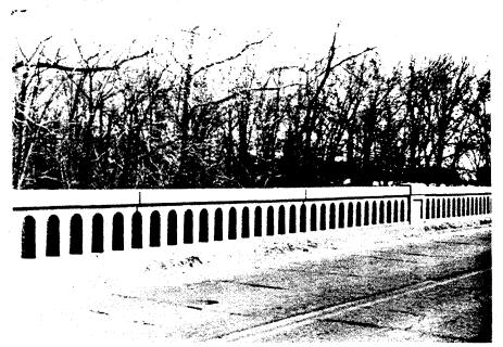
Figure 7-15 Pigeonhole Parapet
