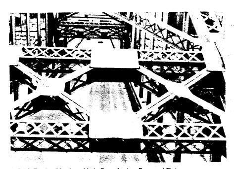
Figure 6-16 Bracing Members Made From Angles, Bars, and Plates
