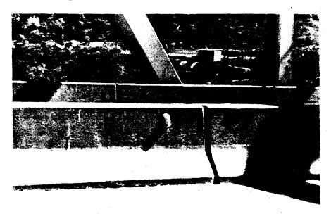
Figure 7-16 New Jersey Type Barrier
