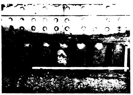
Figure 11-8 Rocker Nest Bearing
