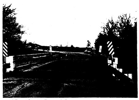
Figure 9-8 Typical Concrete Through Girder Bridge
