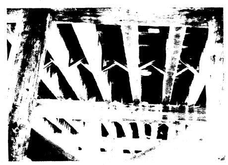
Figure 8-2 Underside View of a Solid Sawn Multi-Beam Bridge
