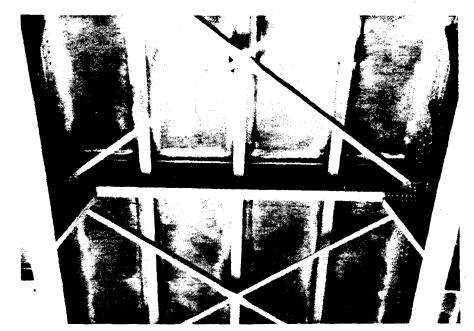
Figure 10-5 Two-Girder Bridge With a Girder-Floorbeam-Stringer System
