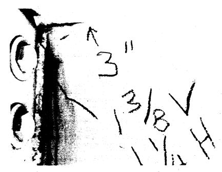
Figure 18-9 Cracks at Top of Floorbeam Connection to Girder
