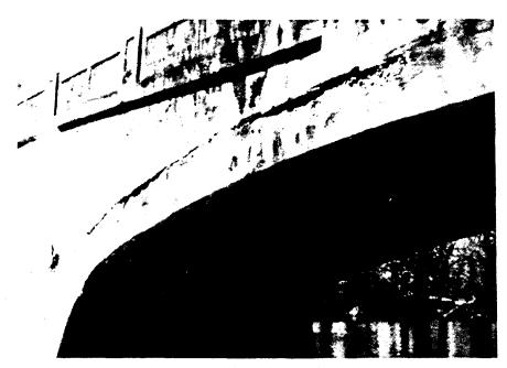
Figure 9-19 Deteriorated Arch/Spandrel Wall Interface
