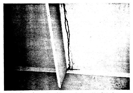
Figure 10-4 Fatigue Crack at Toe of Weld on a Fabricated Multi-Girder Bridge
