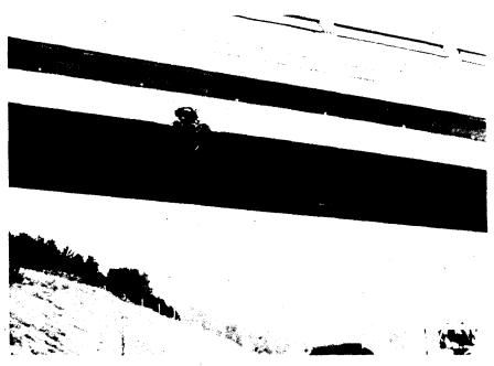
Figure 9-29 Collision Damage on a Prestressed Box Beam
