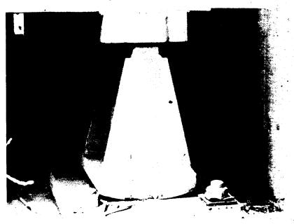
Figure 11-7 Rocker Bearing
