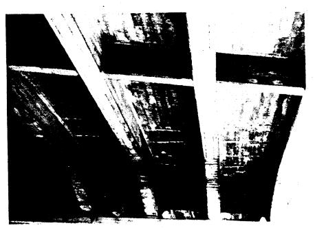
Figure 9-7 Flexure Cracks in Tee Beam Top Flanges
