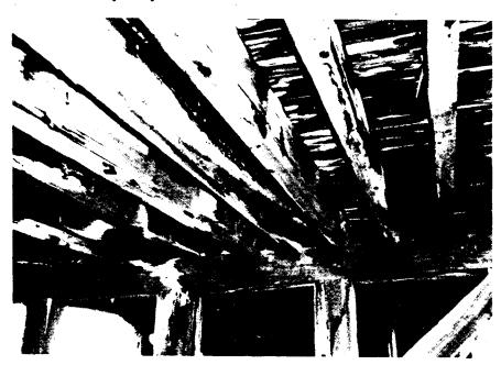
Figure 4-9 Advanced Decay in Timber Superstructure
