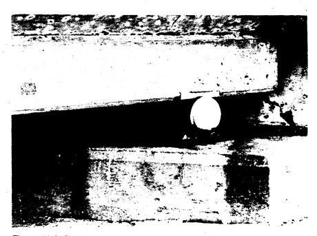
Figure 11-6 Single Roller Bearing
