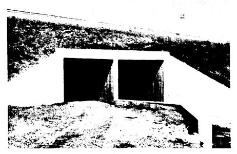
Figure 19-5 Headwall and Wingwall End Treatment
