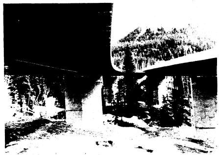
Figure 10-9 Curved Box Girder Bridge
