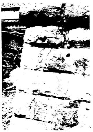
Figure 4-30 Splitting in Stone Masonry
