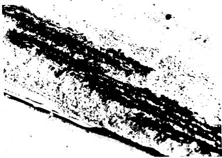
Figure 9-25 Exposed Strands in a Precast Slab Beam
