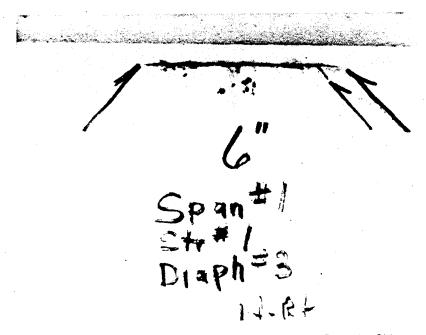
Figure 18-10 Cracked Girder Web Near Top Flange on the Opposite Side From a Diaphragm Connection
