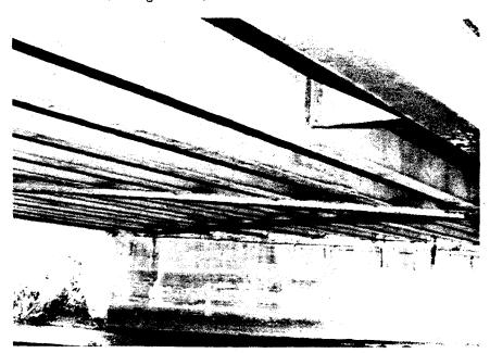
Figure 2-10 Steel Multi-Beam Bridge
