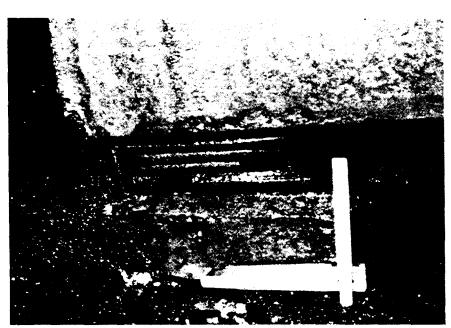
Figure 11-10 Laminated Neoprene Bearing
