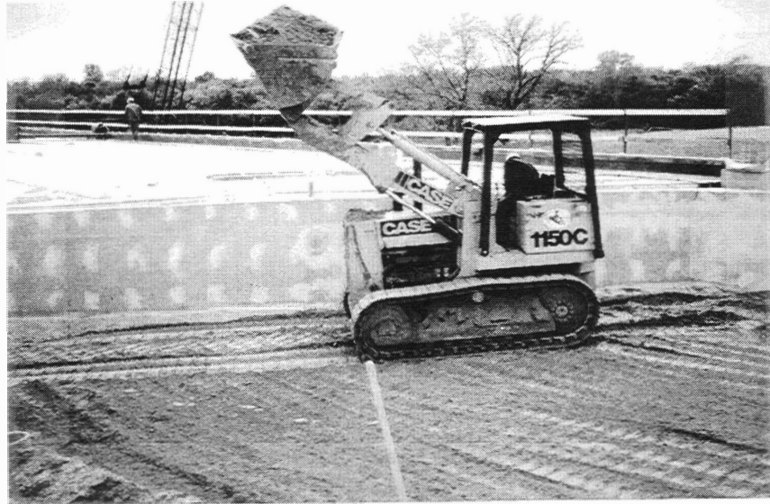
Figure 15. Compaction of Unclassified Borrow for Approach Embankment at North Abutment, Bridge A
