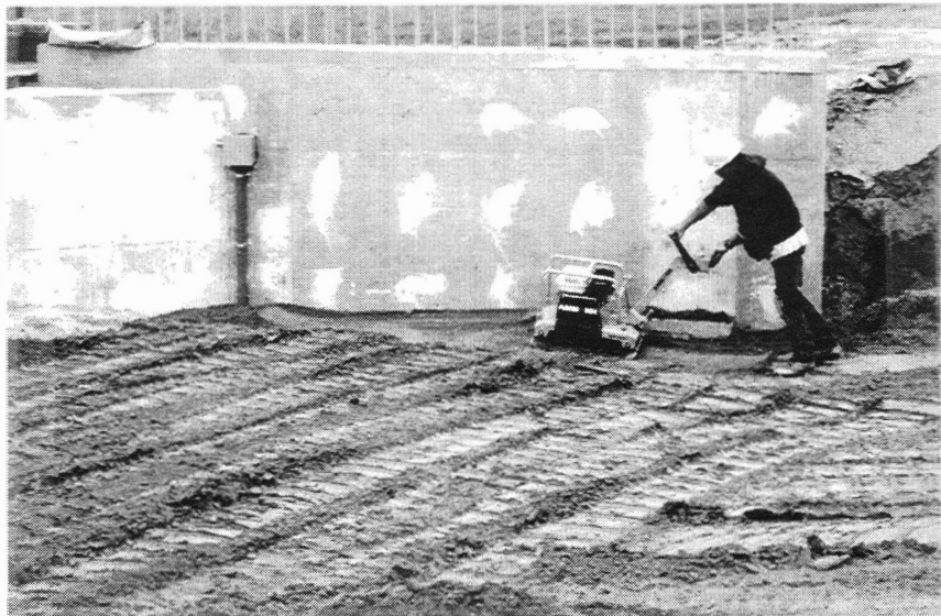
Figure 16. Compaction of Granular Backfill Adjacent to Abutment Wall at North Abutment, Bridge A
