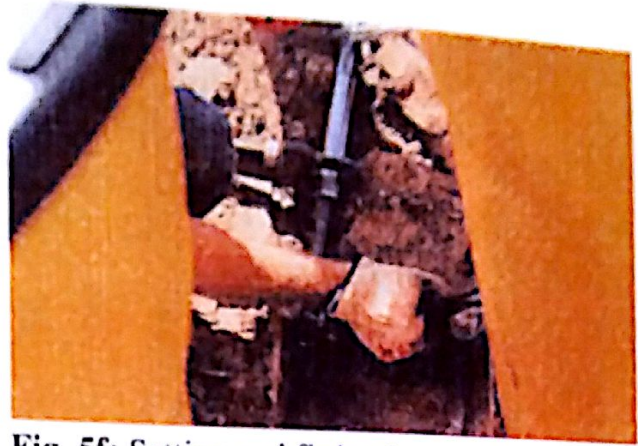
Fig. 5f: Setting end fitting into anchor.
