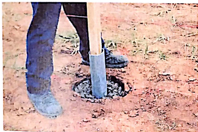
Fig. 4c: Placing post sleeve into concrete base.
