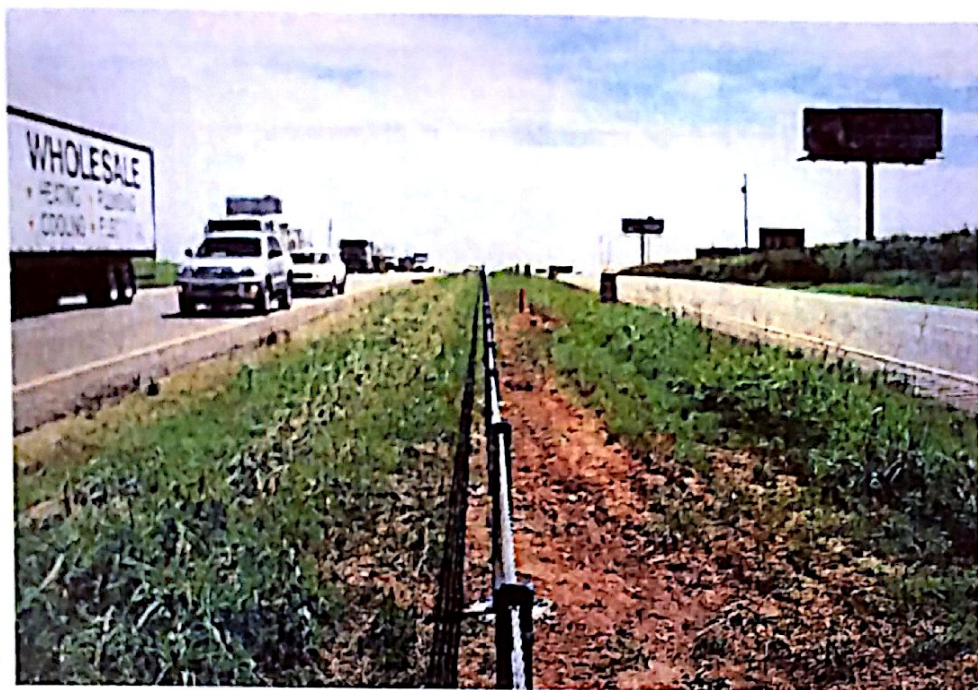
Fig. 5m: Fully assembled and tensioned Safence Cable Barrier System in place on I-35 in Mc Clain County.
