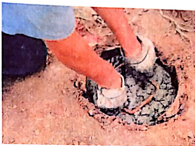
Fig. 4b: Placing reinforcing steel into base.
