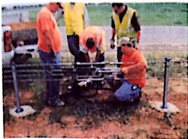
Fig. 5k: Tensioning cable three.
