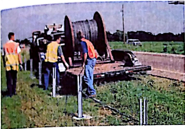
Fig. 5g: Placing bottom cable into posts.
