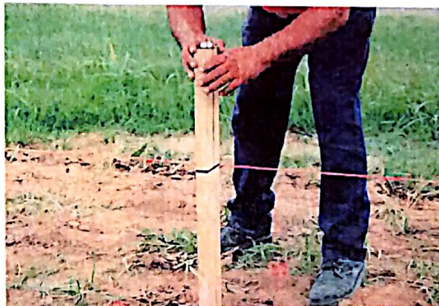
Fig. 4d: Using bubble level and string line to set post position and alignment.
