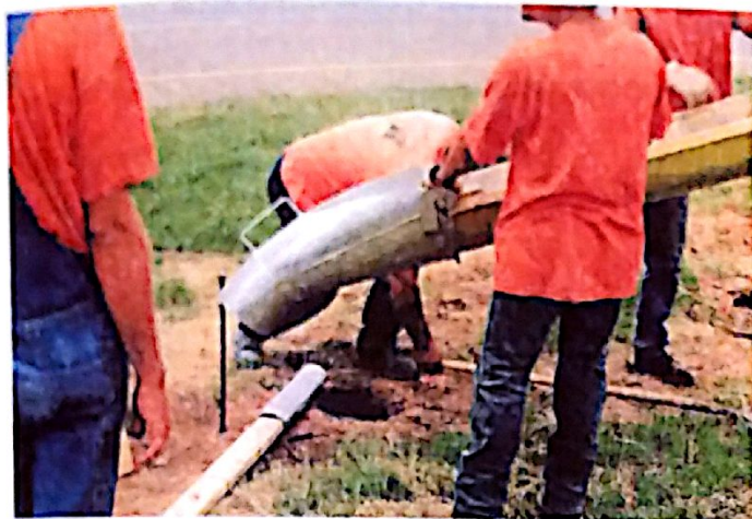
Fig. 4a: Placing concrete for post bases.
