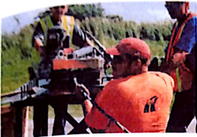
Fig. 5e: Crimping end fitting onto cable.
