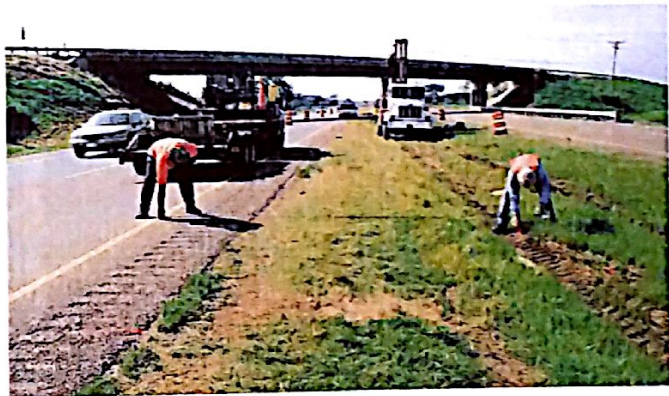
Fig. 3b: Marking post offset from edge of pavement.
