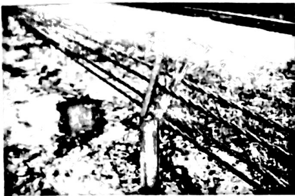
Fig. 6a: Posts have broken away after vehicle collision with fence, but the cable remains intact.
