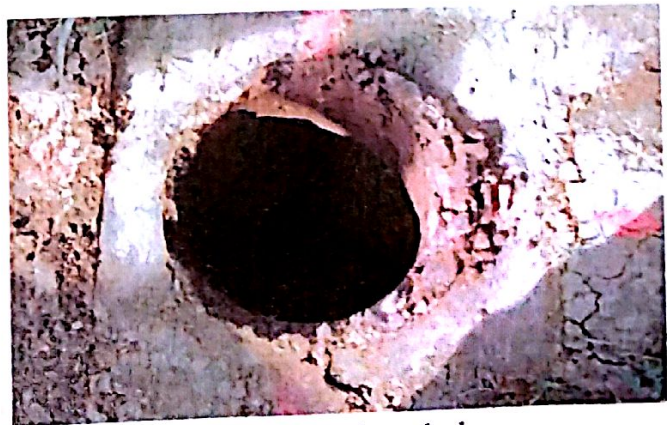
Fig. 3d: Completed post base hole.
