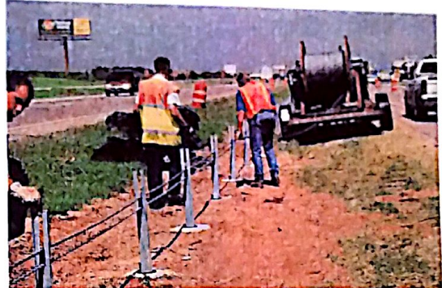
Fig. 5h: Placing second cable and inserting spacers for third cable.
