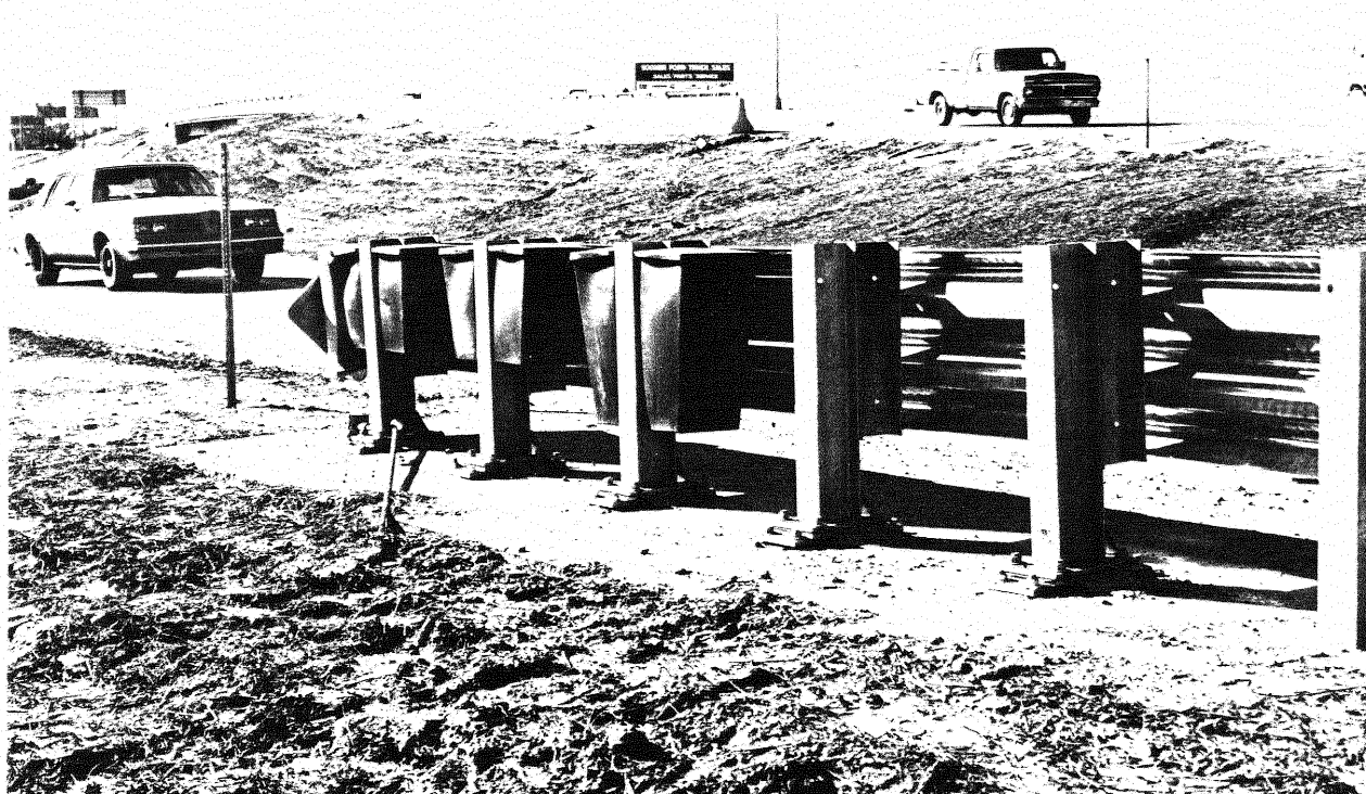
Figure 1. SENTRE unit after installation on guardrail end.
