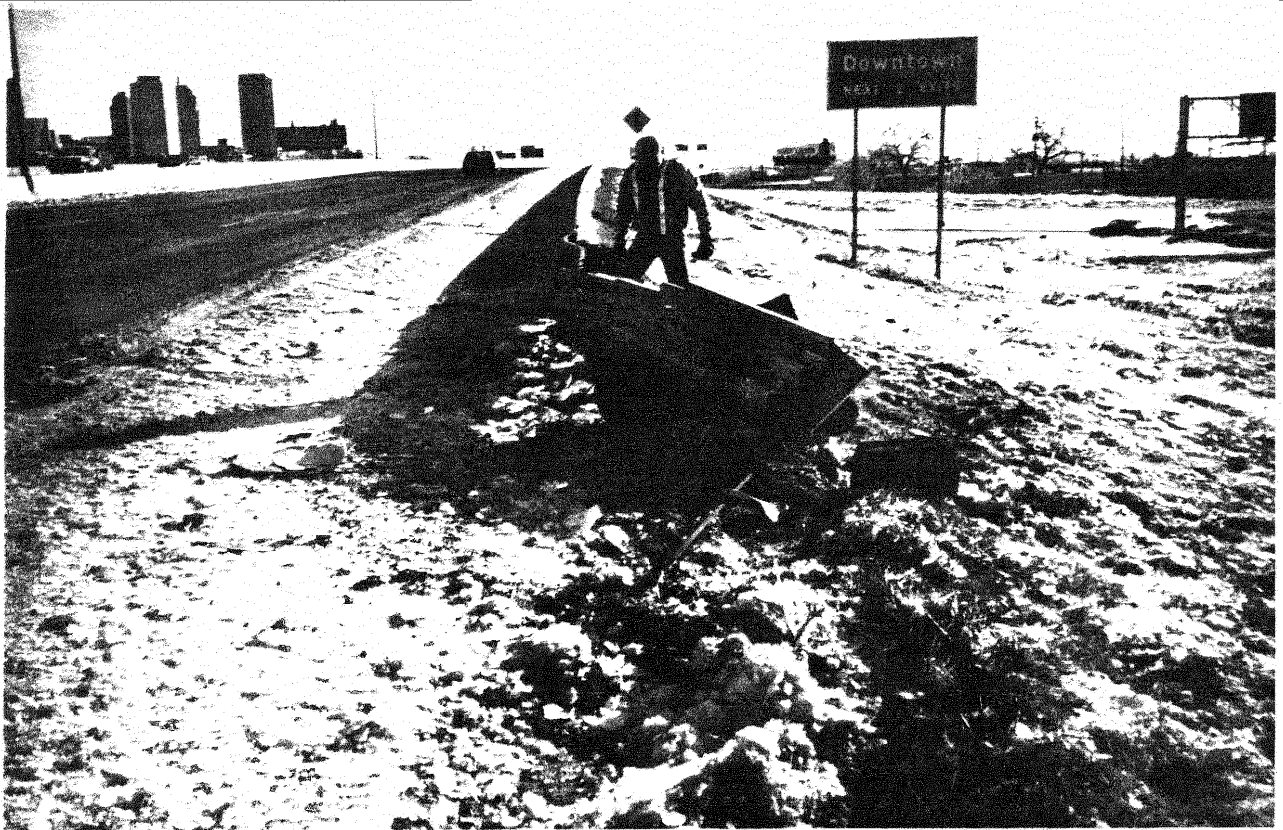
Figure 7. After collision - unit functioned as intended.
