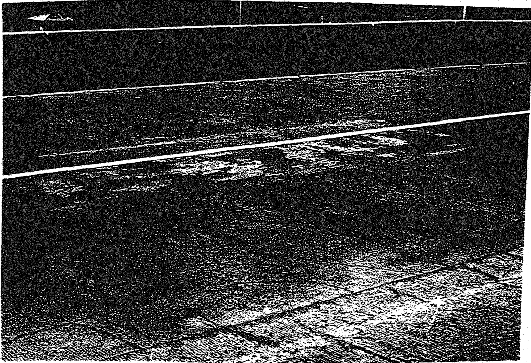
Figure 4. Cracks in Pavement.
