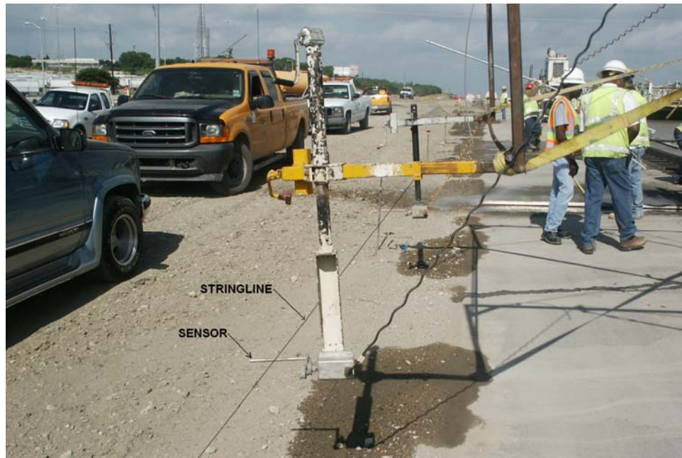
Figure 2-4. Stringline Set-Up on a Concrete Paving Project.
