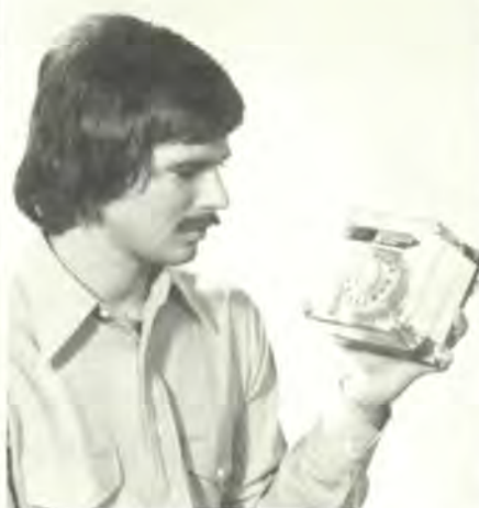
Steve Peirce studies a disc recorder from a GM fleet project. Since the start of this particular project in June 1973, over 100 of the 500 recorders installed in cars have been returned. About 20 of these contain accident data.
