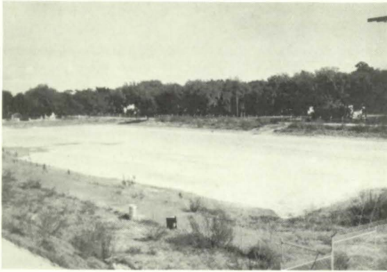
Fenced detention basins can be used to lower flood peaks and reduce costs for outlet structures.
