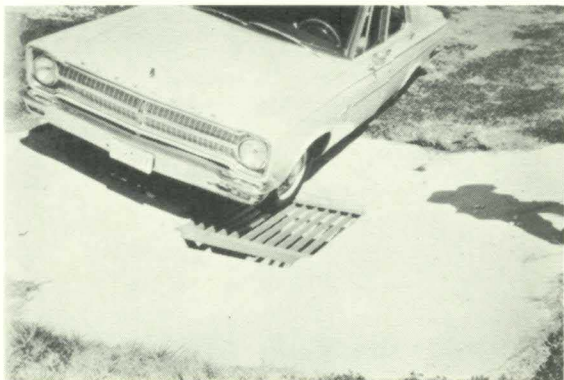
Median inlets which present a safety hazard (left photo) should be avoided. Photo at right shows a flush type grate inlet with slots for small debris.
