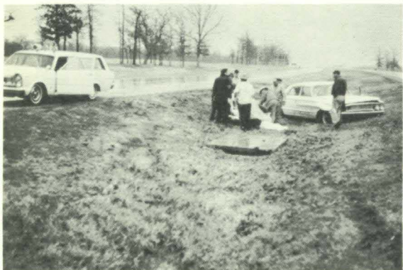
Median inlets which present a safety hazard (left photo) should be avoided. Photo at right shows a flush type grate inlet with slots for small debris.
