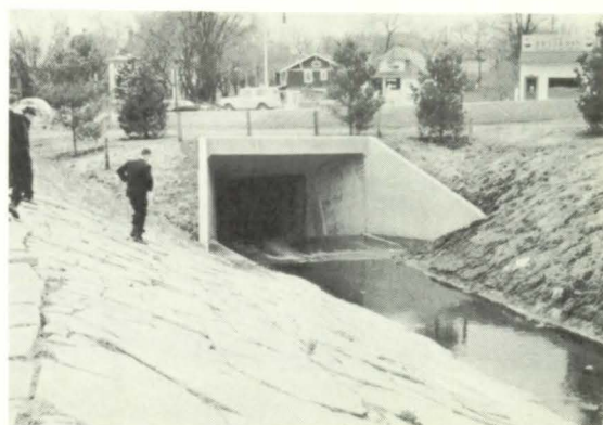
An improved culvert entrance which accelerates flow thus increasing capacity. Especially beneficial on long culverts on steep grades.
