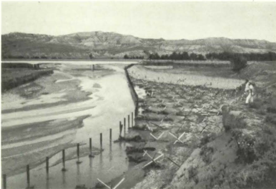
River training works controlling the natural river meanders to fit the bridge location.
