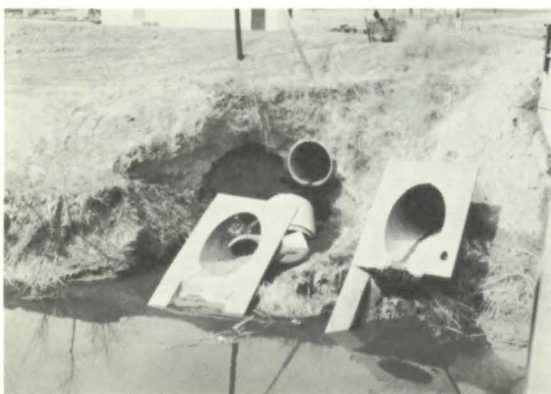
Sectional pipe is particularly vulnerable to scour at culvert outlet.
