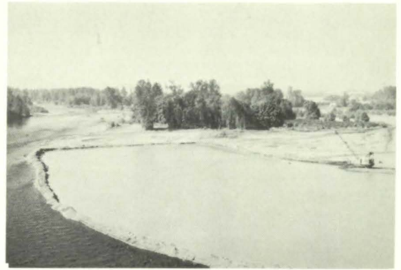
A dike separating the clear river flow from a borrow pit area, thus avoiding damage to fish and their habitat.
