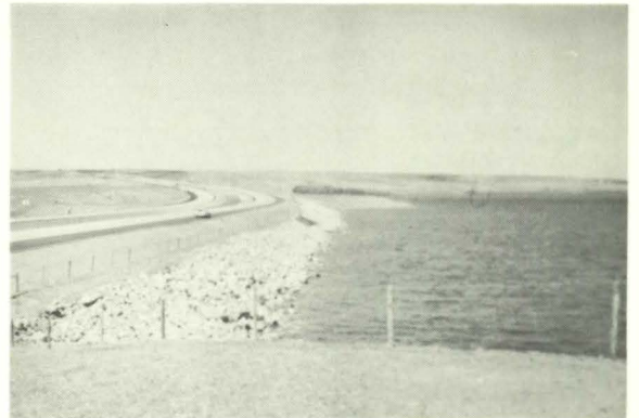
An Interstate highway embankment serves as a dam for a recreation reservoir. Built as a cooperative highway and recreation project.
