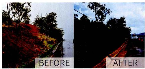
Figure 5 Install hydro mulch and netting to prevent soil erosion along Kawainui Watershed (adopted picture from Hawaii Department of transportation website)
