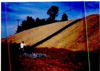
Figure 25 Slope drains, adopted from [30]
