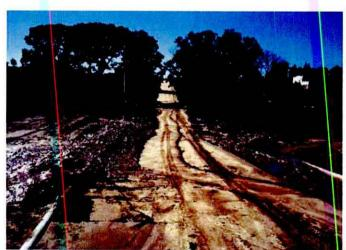
Figure 4 Sediment in Street Due to Inadequate Erosion and Sediment Control During Construction, adopted picture from [6]
