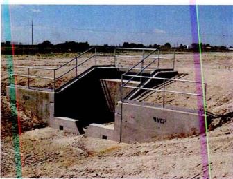
Figure 10 Energy Dissipators, adopted picture from [27].
