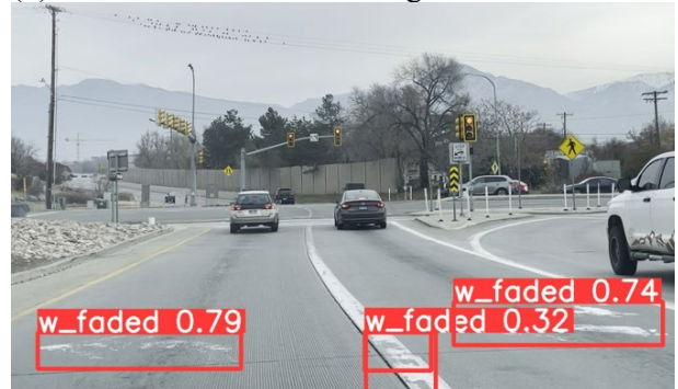
(f) Faded White Arrow and Lane Markings-2
