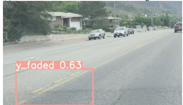
(h) Faded Yellow Double Lane Marking
