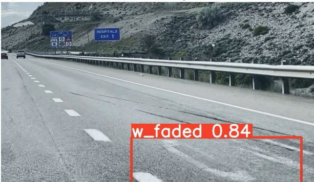
(c) Faded White Word Marking-1
