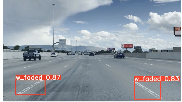
(b) Faded White Lane Marking-2
