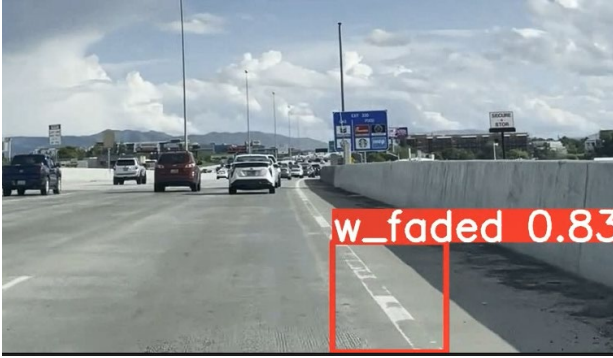
(a) Faded White Lane Marking-1
