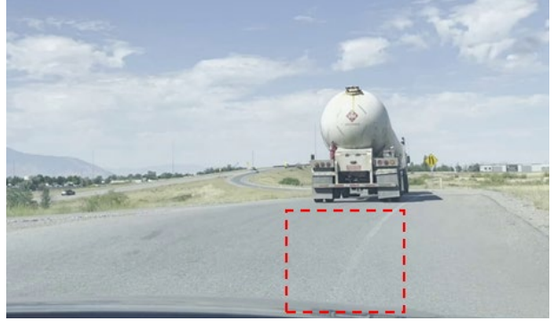
(b) Almost Fully Faded Marking
