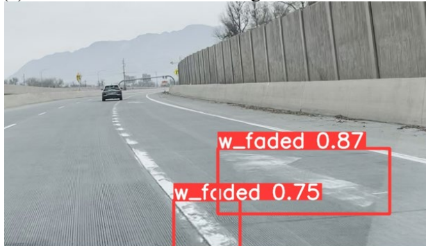
(e) Faded White Arrow and Lane Markings-1
