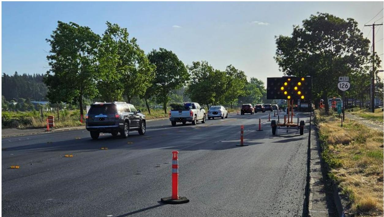
**Figure 6.3: Smart Arrow Board Deployment**
