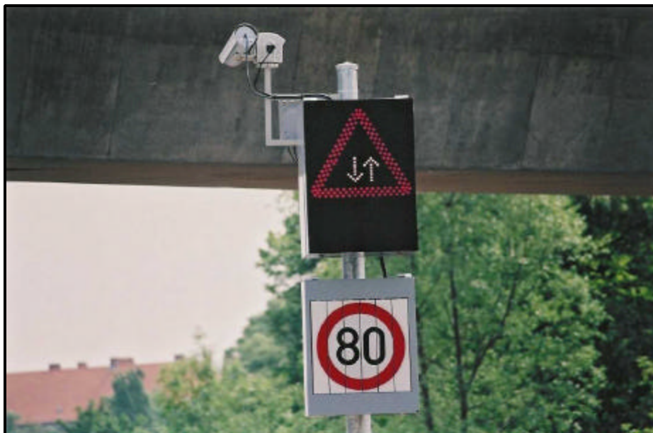
Figure 2-19. Variable Speed Limit Sign on Autobahn 100 in Germany. 39
