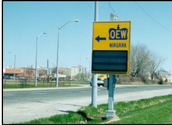
Figure 2-10. Arterial Advisory Sign with VMS Panel. 28
