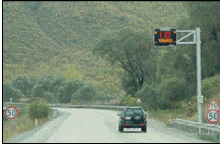
Figure 2-29. Doppler Radar Speed Warning System on Turkish Motorway. 47
