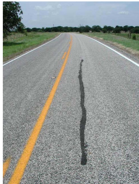
Figure 14. Longitudinal Cracking on Control Section on FM 1915.
