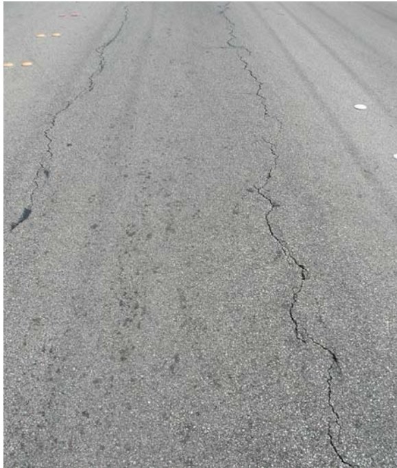
Low Severity Fatigue Cracking
