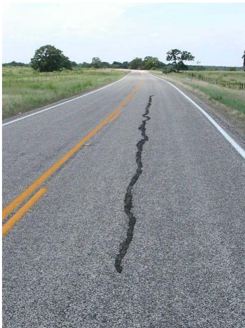
Figure 14. Longitudinal Cracking on Control Section on FM 1915.
