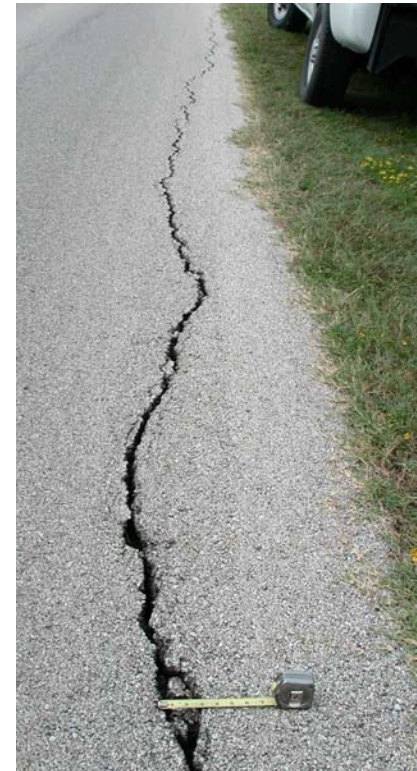
High Severity Longitudinal Cracking
