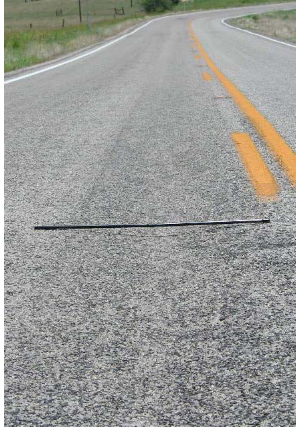
Figure 13. Longitudinal Crack and Rutting on First Geogrid Section on FM 1915.
