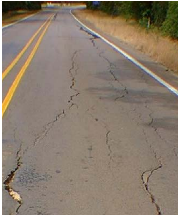
Figure 1. Example of Longitudinal Cracking.
