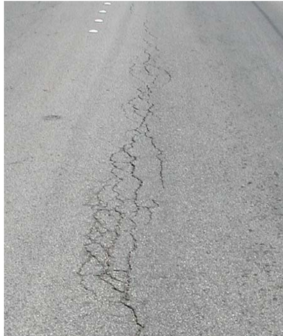
Medium Severity Fatigue Cracking
