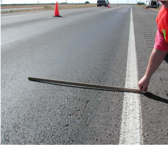
Low Severity Rutting
