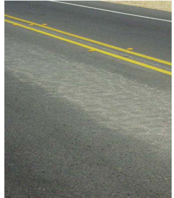
High Severity Fatigue Cracking
