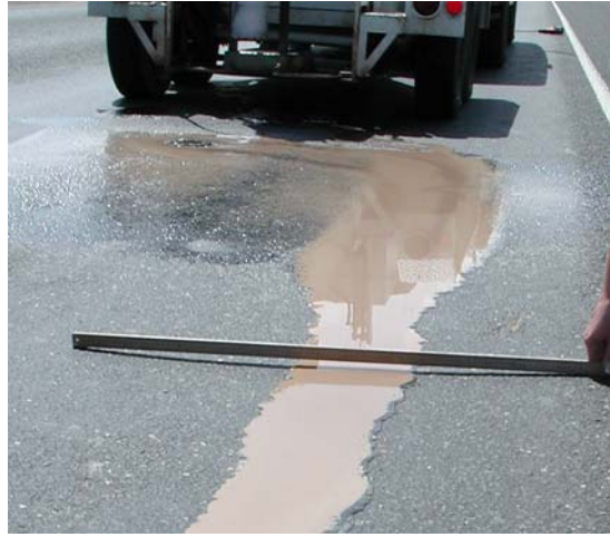
Medium Severity Rutting
