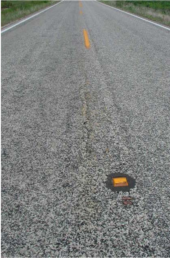
Figure 13. Longitudinal Crack and Rutting on First Geogrid Section on FM 1915.
