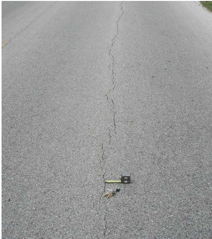
Low Severity Longitudinal Cracking
