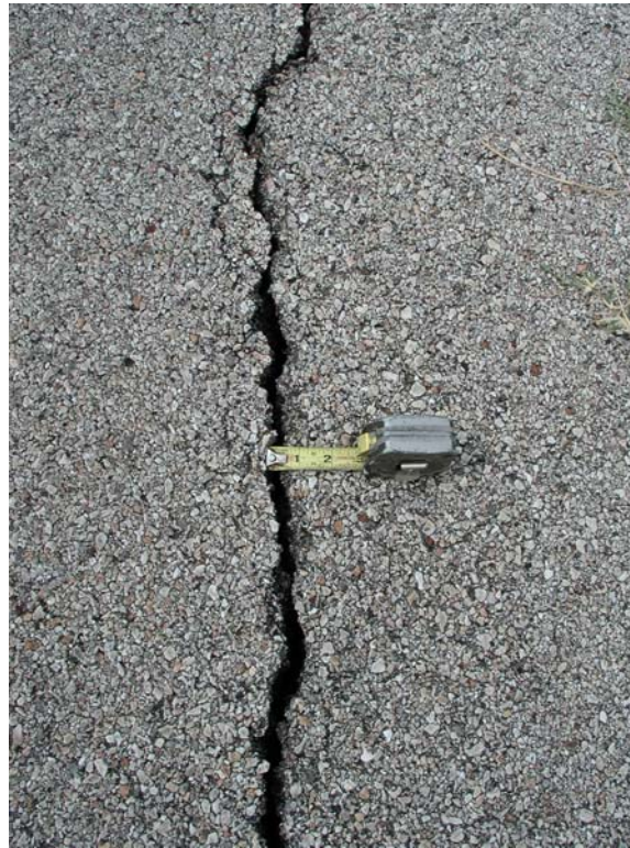
Medium Severity Longitudinal Cracking
