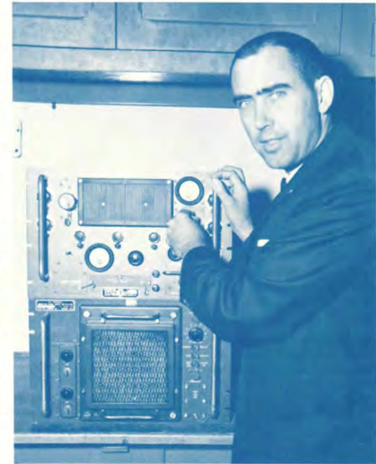
SEMT Austin E. Sterling demonstrates the UHF transmitter for which he suggested modifications. Suggestion won him $500 cash award, based on estimated first-year savings of $10,000 to the Agency.
