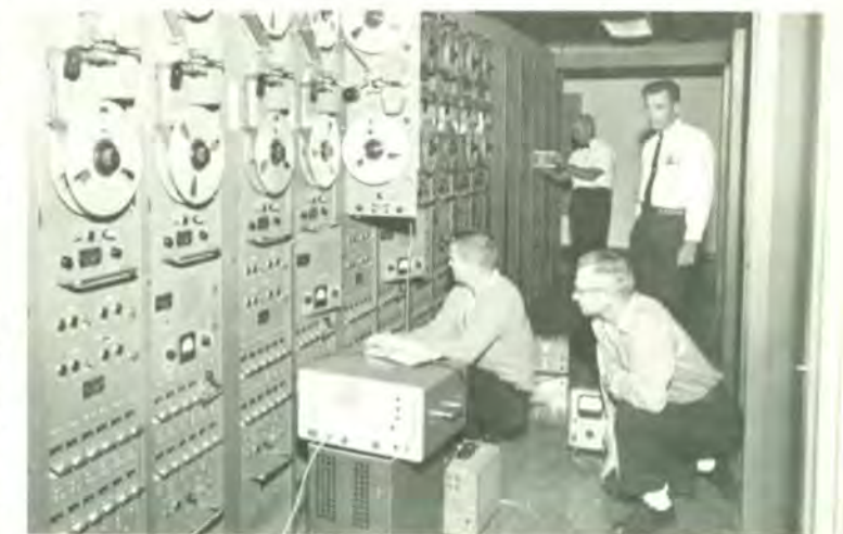
These EMTs are checking the voice recorder system at the Fort Worth Center. Each tape on the reels shown in the foreground is capable of recording 22 simultaneous conversations between aircraft and controllers. From left to right are DOYLE D. GRAVES, LOYD C. LOWRIE, JAMES D. DUCOTE, and FRED W. BOWERS.
