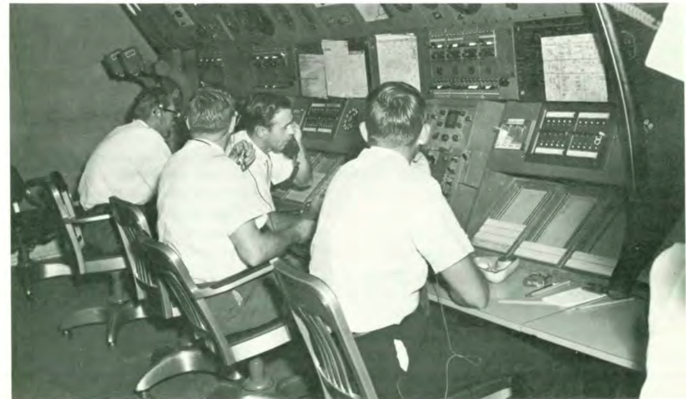
Radar room in an approach control tower. Positions, left to right, are PAR, flight data, approach control, flight data.
