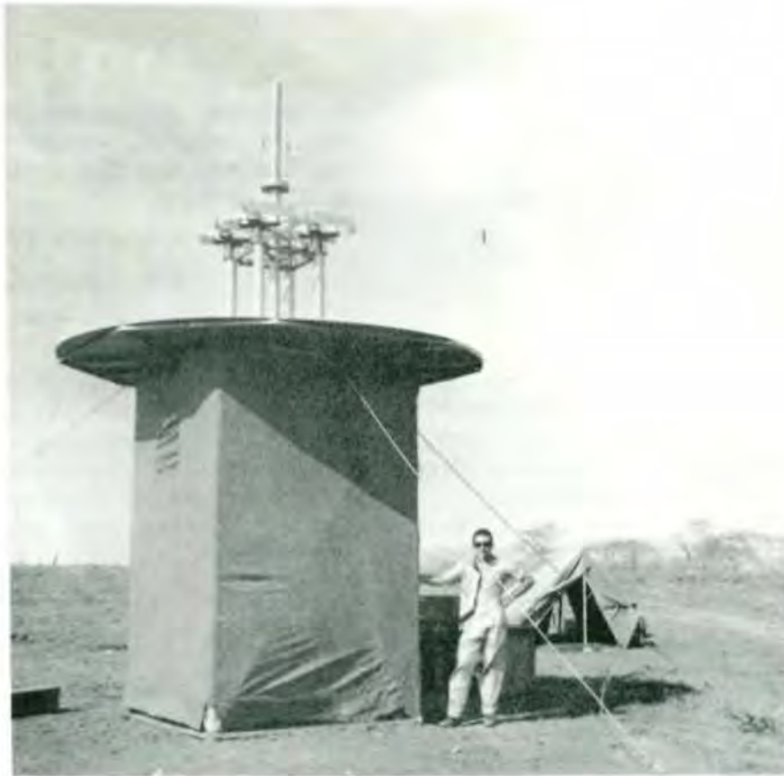
Portable VOR assembled and ready for flight check, Barcelona, Venezuela.
