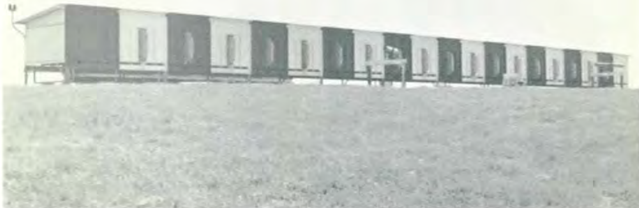
Directional Wave Guide Localizer The very narrow radio beam provided by this facility guides aircraft down the centerline of the runway
