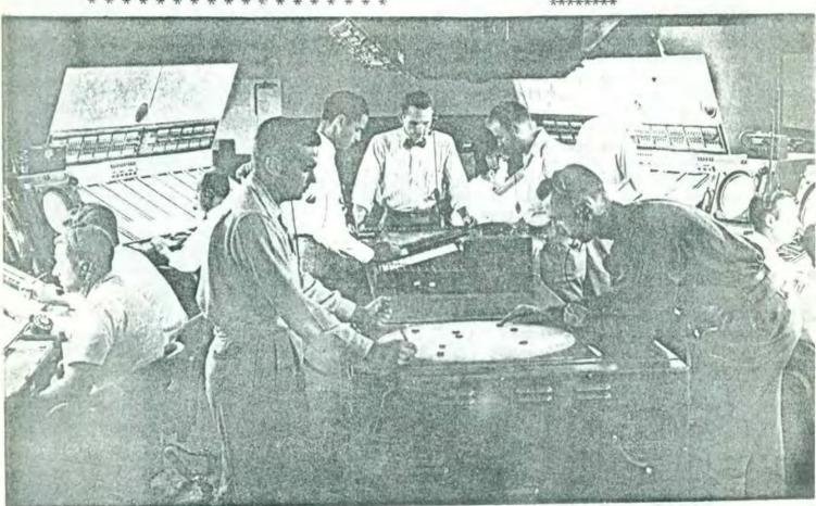
FAM electronics engineers have done an expert job putting Long Range Radars (ARSR-1) into operation as tools for air traffic controllers. Radars now operating at Fort Worth, Memphis, and Raleigh-Durham. Others to go in soon.
