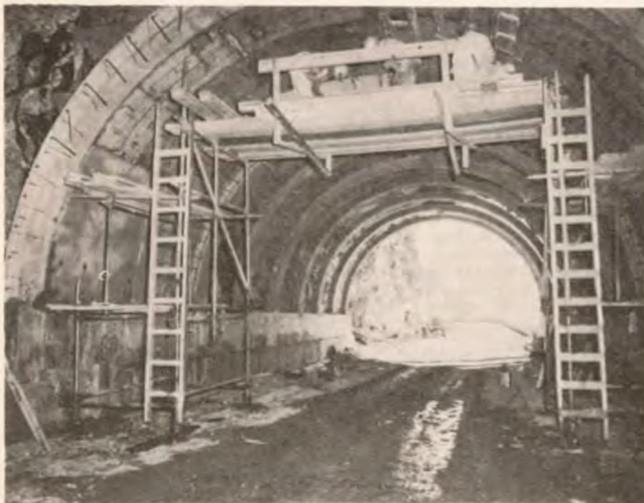
Precast concrete tunnel-liner rings
