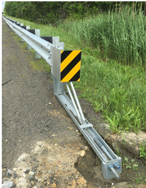
Figure 8. Photograph. X-Tension telescoping end treatment impact head.
