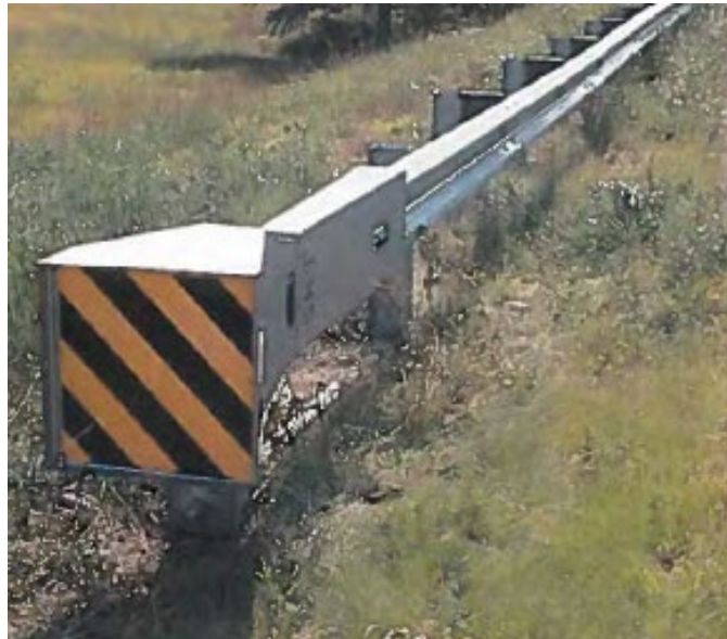
Figure 4. Photograph. SKT extruding end treatment impact head.
