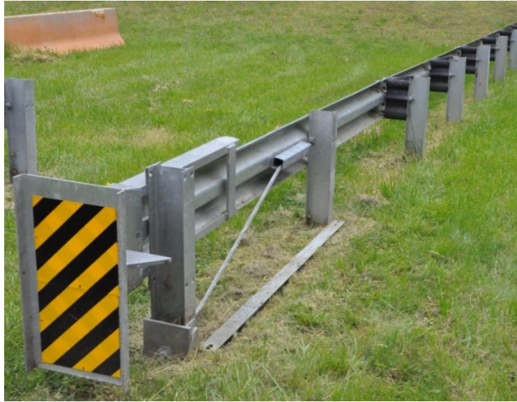
Figure 2. Photograph. ET Plus extruding end treatment impact head (4- and 5-inch guide channels).
