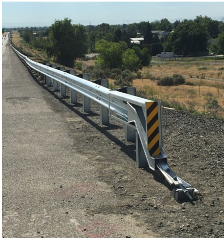
Figure 3. Photograph. SoftStop extruding end treatment impact head.
