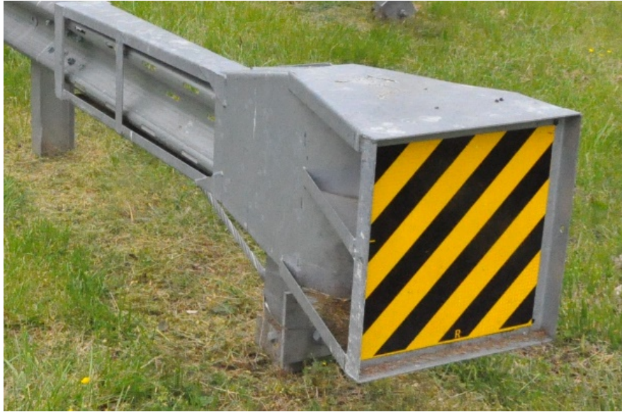
Figure 4. Photograph. SKT extruding end treatment impact head.
