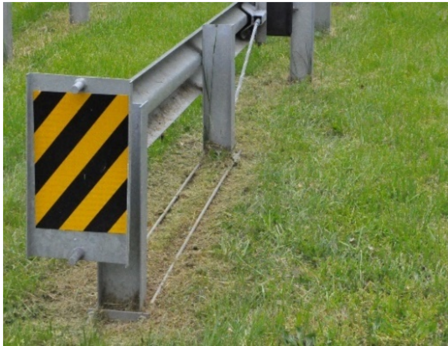
Figure 7. Photograph. X-LITE telescoping end treatment impact head.
