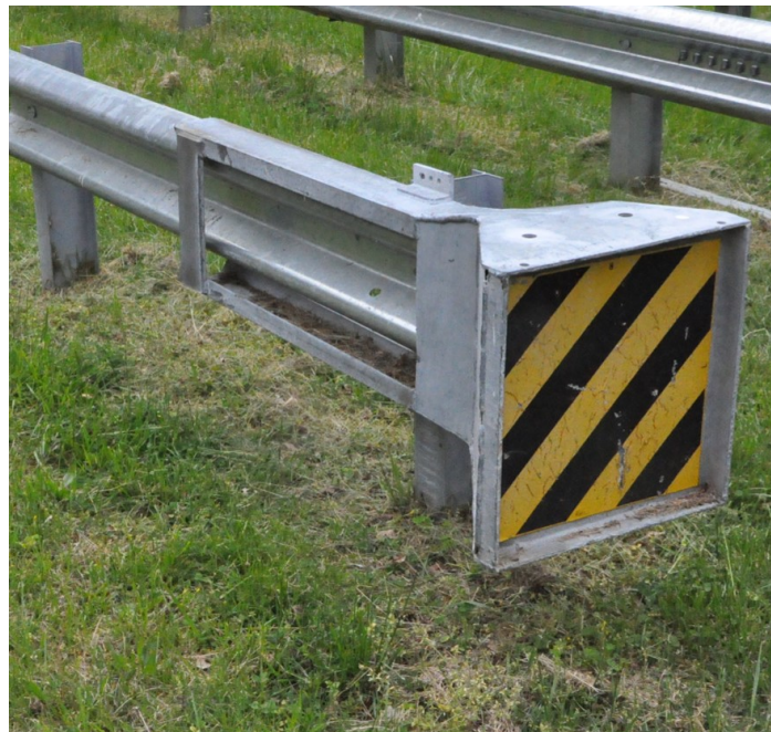
Figure 1. Photograph. ET 2000 extruding end treatment impact head.
