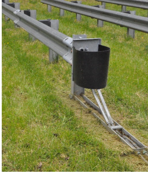
Figure 8. Photograph. X-Tension telescoping end treatment impact head.
