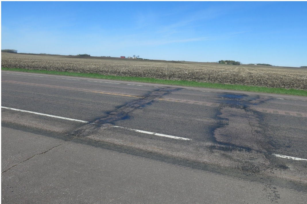
Figure 4.16 Deteriorated pavement surface.
