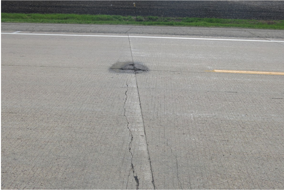
Figure 5.4 Surface distress (Site #2).
