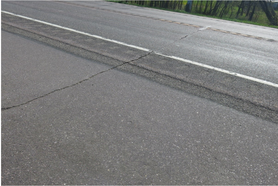
Figure 4.13 Reflective transverse cracking.
