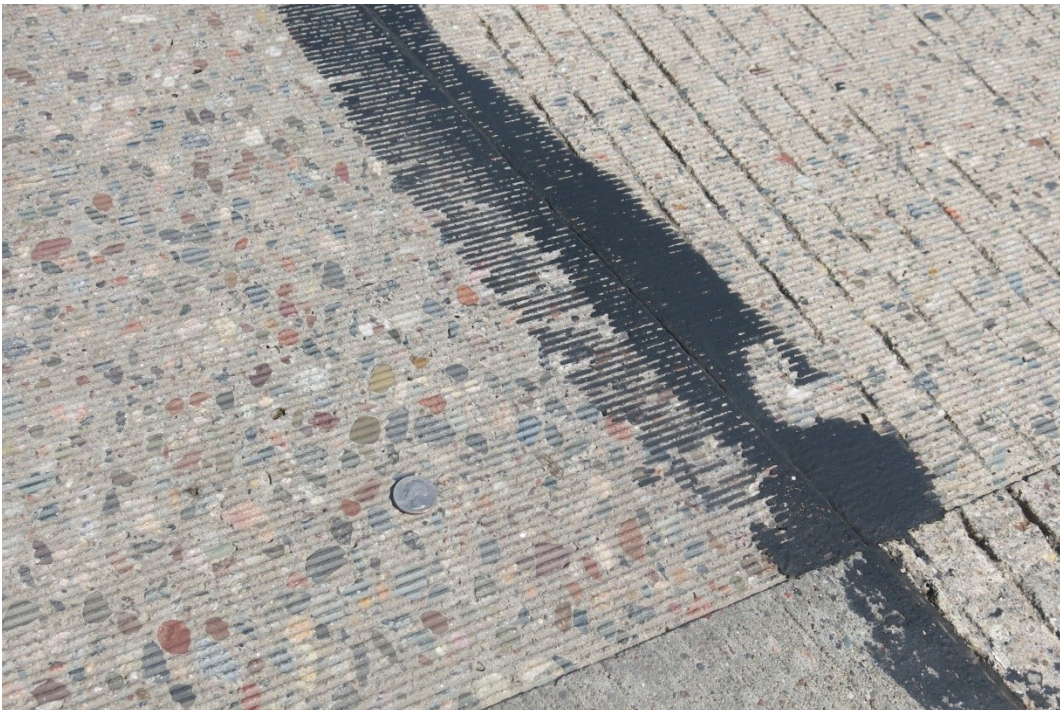
Figure 4.20 Diamond grinding.
