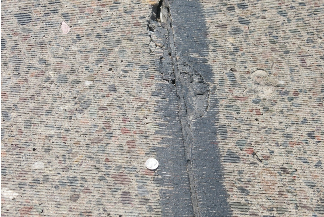
Figure 4.21 Spalling at transverse joint.
