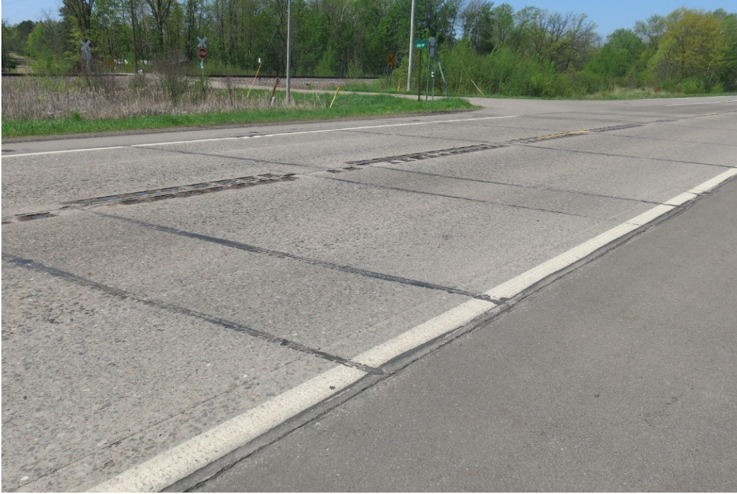
Figure 4.19 Partial- and full-depth repair.
