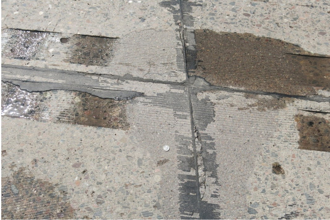
Figure 4.23 Cracking in the vicinity of joints.
