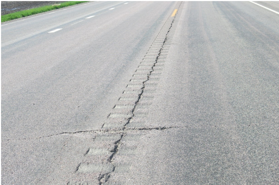
Figure 4.14 Longitudinal cracking on the centerline.
