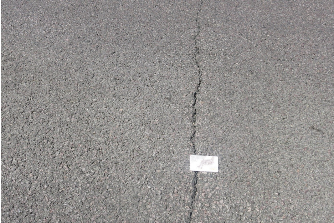
Figure 4.10 Transverse reflective cracking.
