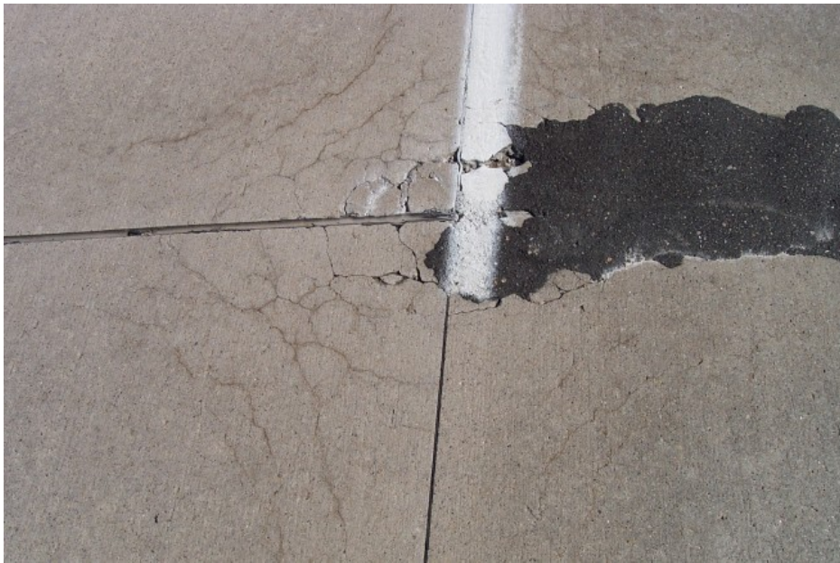
Figure 3.16 D-cracking (MnDOT, 2011).
