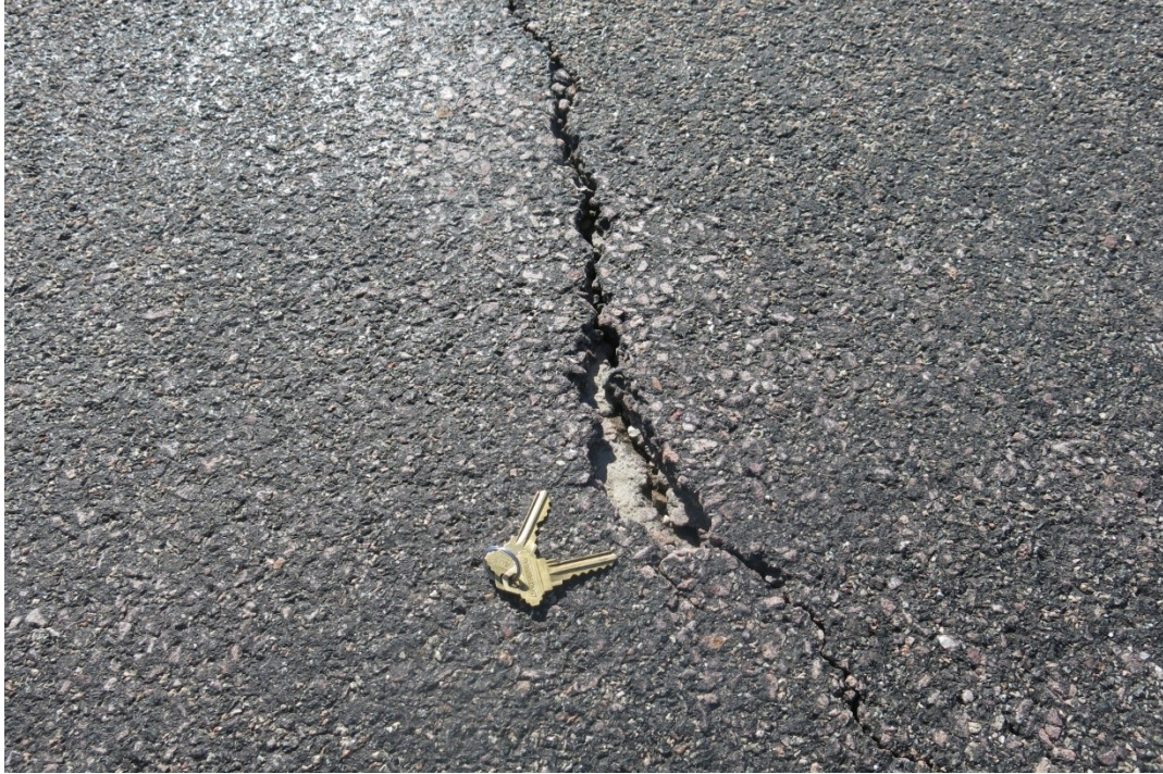
Figure 4.15 Material loss in cracks.
