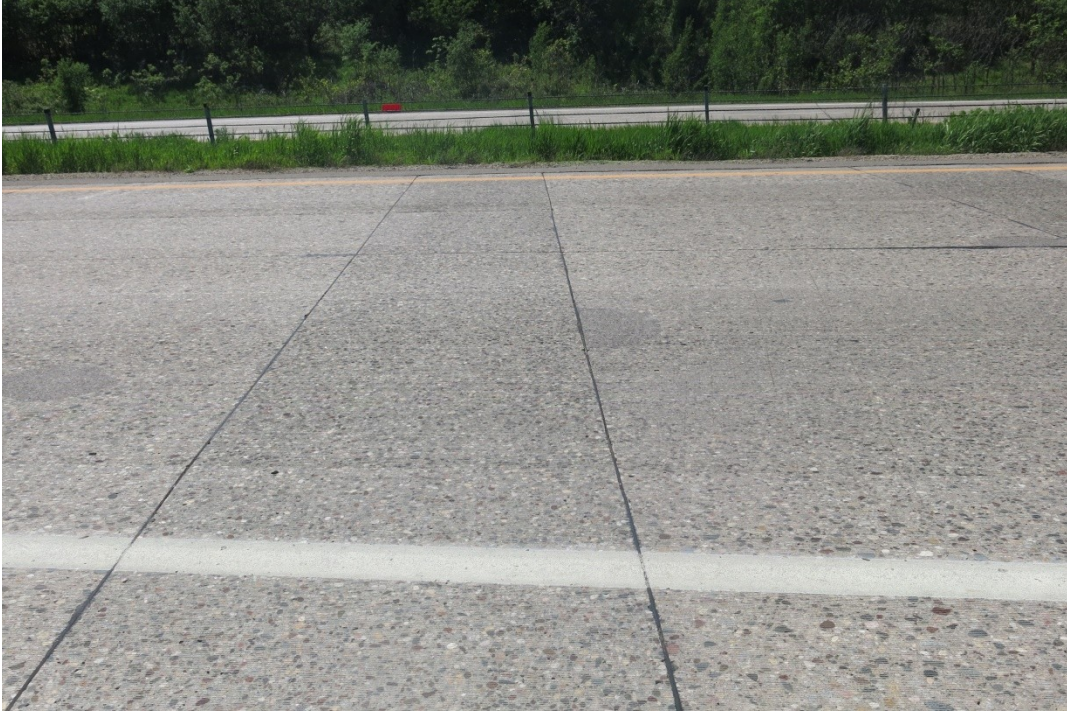
Figure 4.26 Diamond ground pavement surface.
