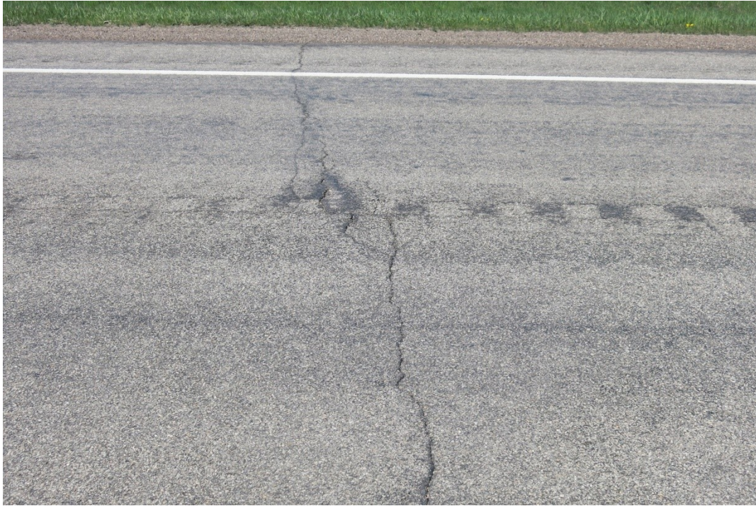
Figure 4.6 Advanced cracking at transverse joint of the original concrete layer.
