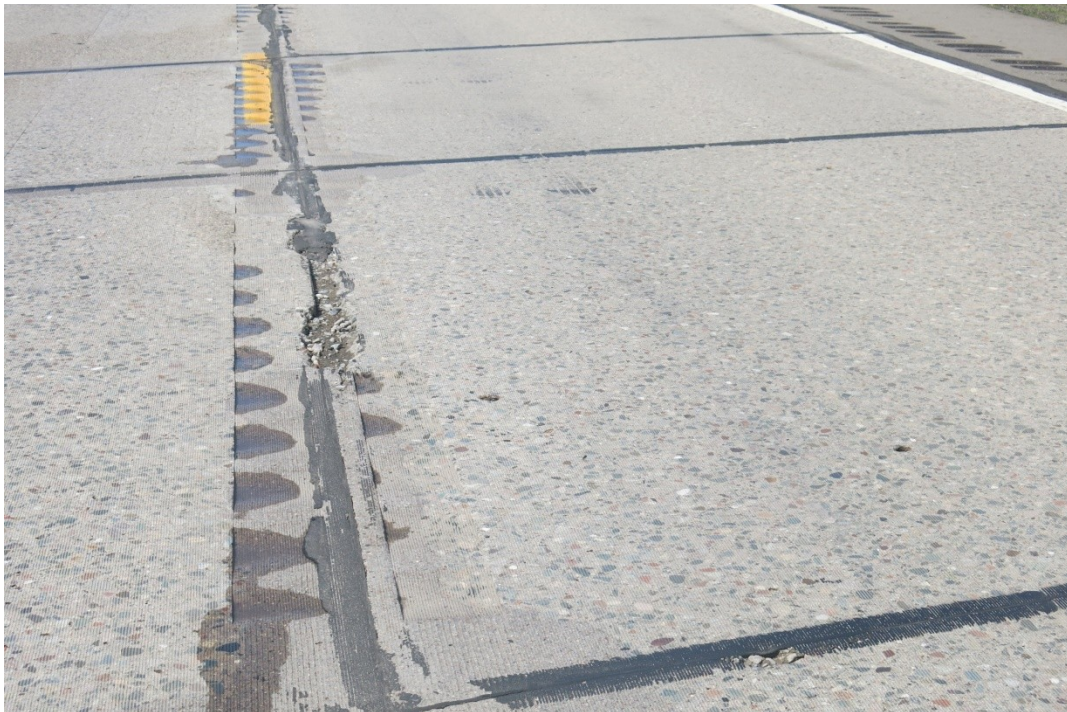
Figure 4.22 Spalling at longitudinal joint.
