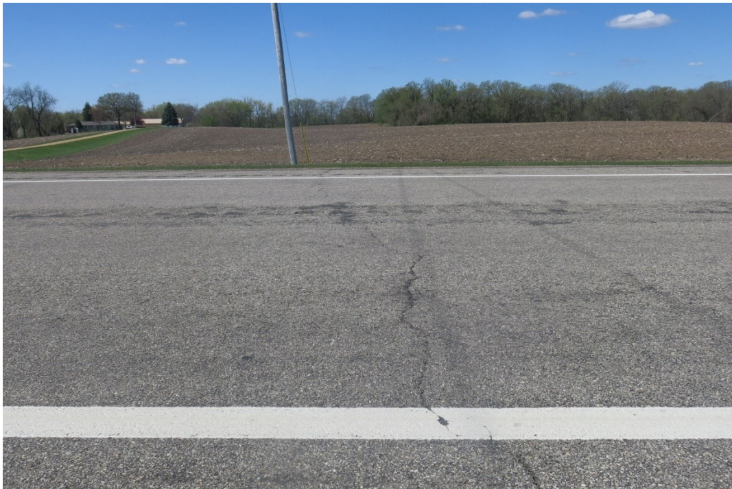
Figure 4.5 Randomly oriented transverse cracking.
