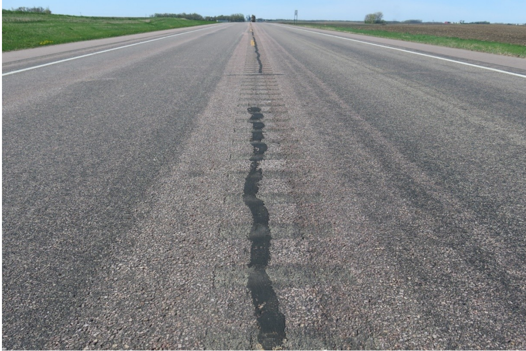
Figure 4.17 Sealed longitudinal cracks.
