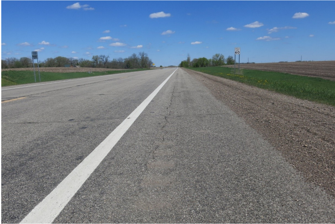
Figure 4.4 Longitudinal cracking on shoulder along the original pavement edge.
