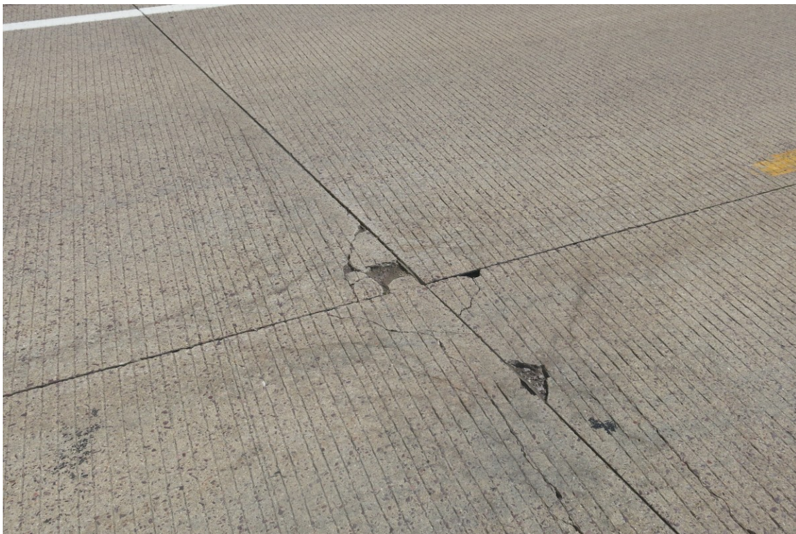
Figure 5.3 Surface distress (Site #2).
