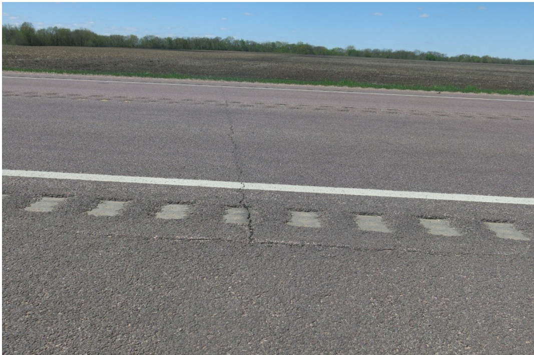
Figure 4.11 Longitudinal cracking along the original pavement edge.
