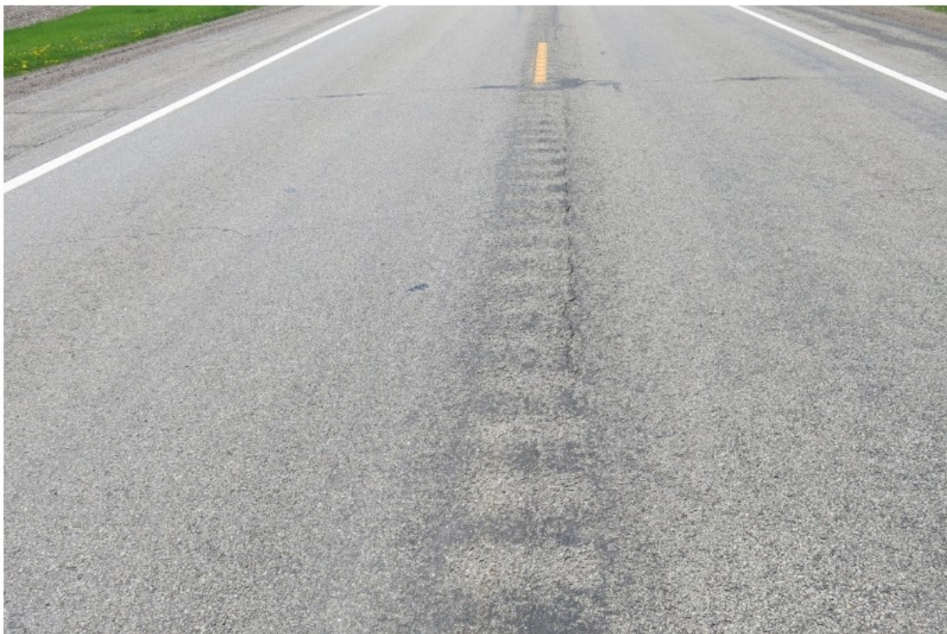
Figure 4.3 Reflective cracking on the centerline.
