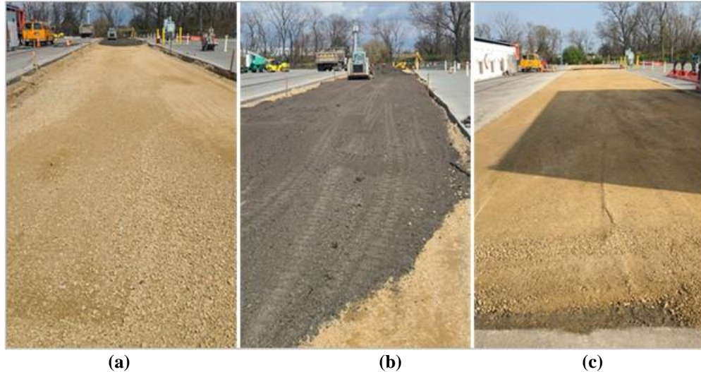
Figure 4. (a) Placement and Partial Compaction of Bottom 4-Inch VDOT 21B; (b) Placement and Partial Compaction of Middle 3-Inch Reclaimed Asphalt Pavement Millings; (c) Placement and Partial Compaction of Top 4-Inch VDOT 21B
