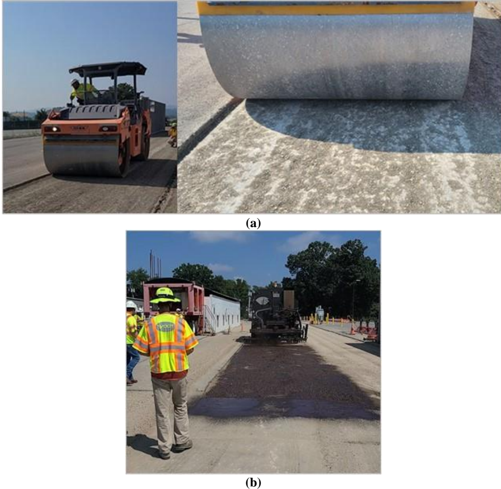
Figure 6. Full-Depth Reclamation Layer: (a) Microcracking; (b) Fog Sealing
